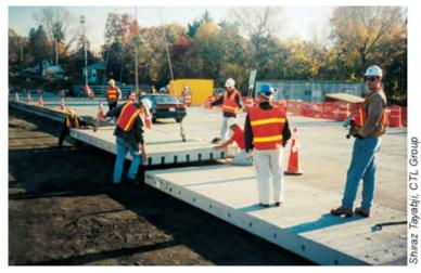
Figure 15. Prefabricated panels used at the Tappan Zee Toll Plaza in New York
