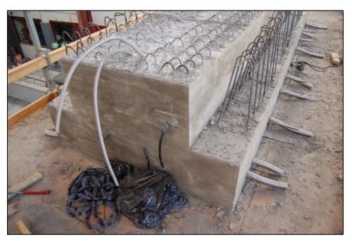
Figure 5.4: Completed Bent Cap Construction on Top of Column
