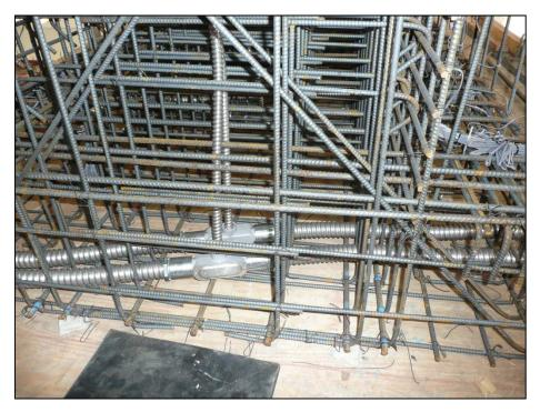
Figure 5.9: Routing of Bent Cap Ducts
