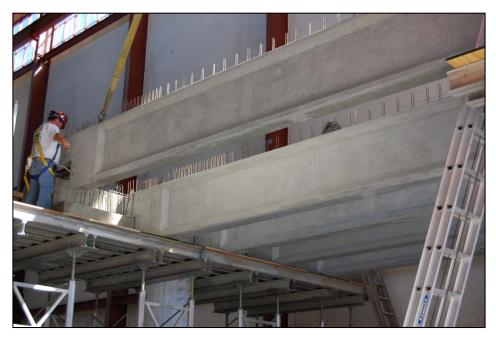
Figure 5.5: Installation of Southern Girders
