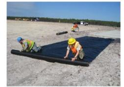
Figure 1. Geosynthetic reinforcement used on TB1: (a) BX geogrid, (b) GC100/150, (c) C30, and (d) PPWF
