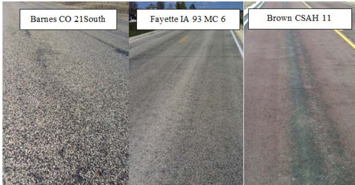
Figure 27. Comparison of surface conditions for CIR sections with chip seal
