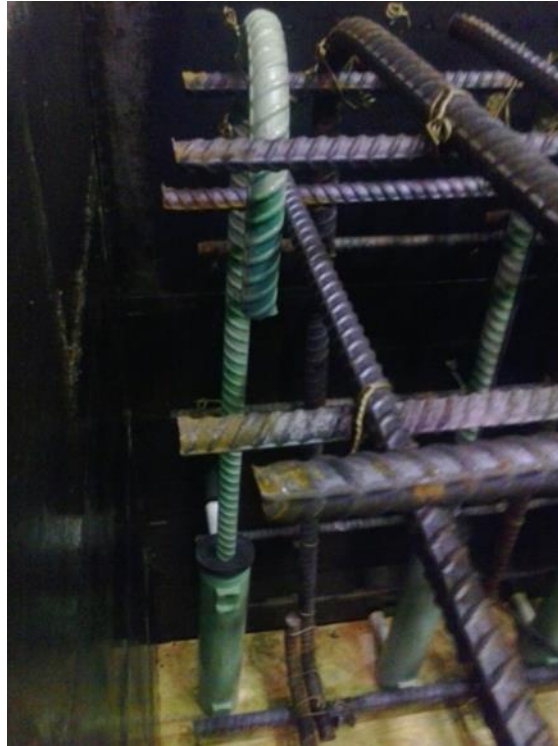
Figure 27. Grouted coupler and reinforcing bar
