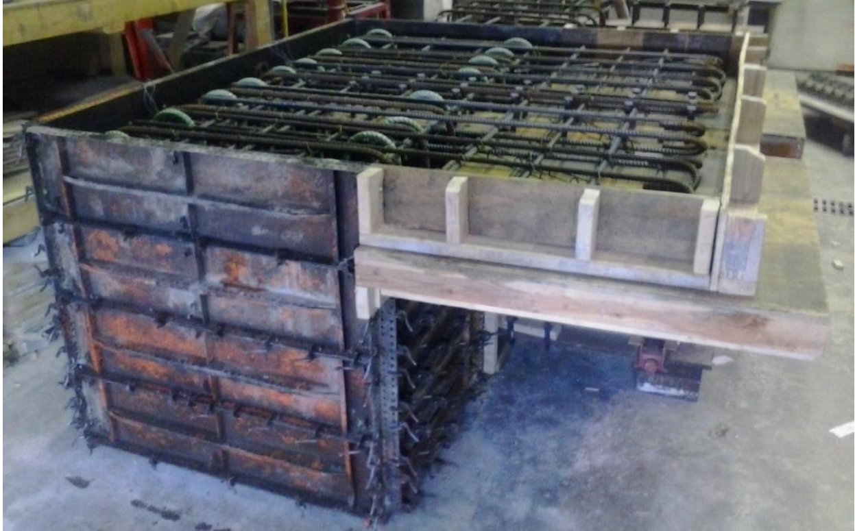
Figure 28. Integral diaphragm and deck, formwork, and reinforcing bar
