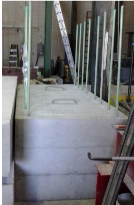
Figure 20. Cast-in-place pile cap
