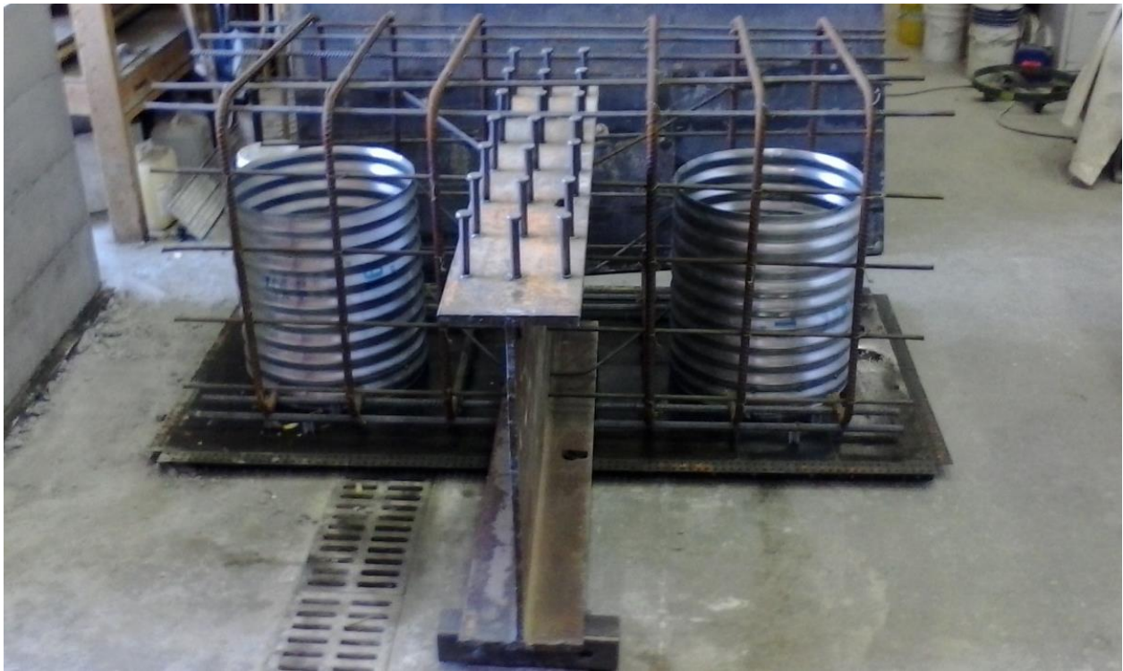
Figure 43. Integral diaphragm reinforcing bar cage
