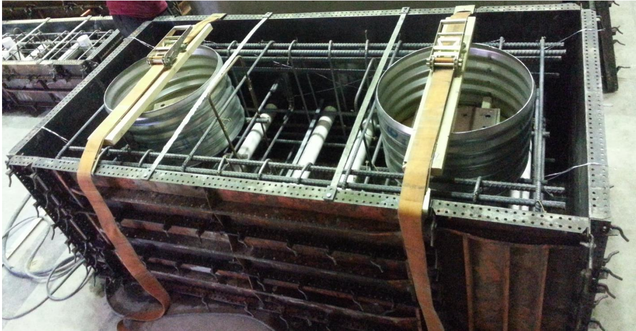
Figure 38. Pile cap reinforcing bar, formwork, and CMP
