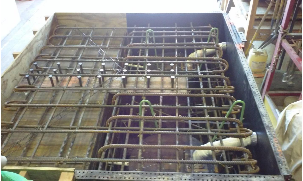
Figure 45. Integral diaphragm deck reinforcing bar
