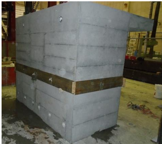
Figure 50. Grout bed formwork front
