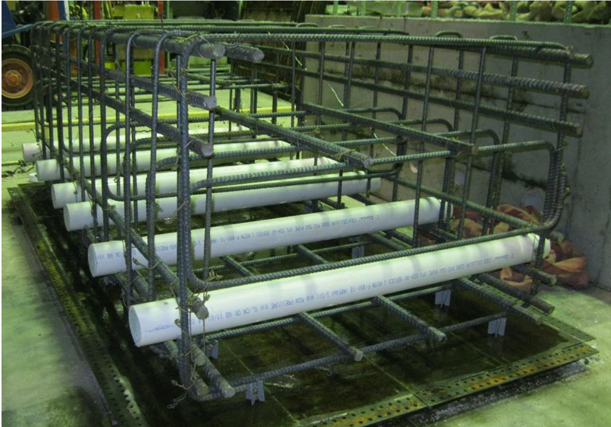
Figure 37. Pile cap reinforcing steel bar cage
