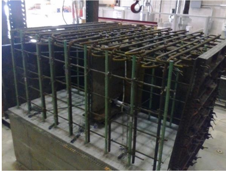
Figure 21. Cast-in-place integral diaphragm
