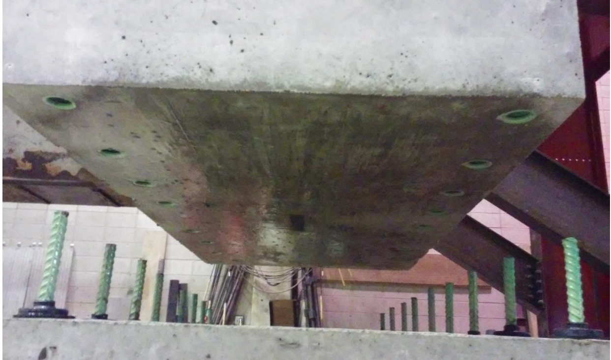
Figure 32. Integral diaphragm placement
