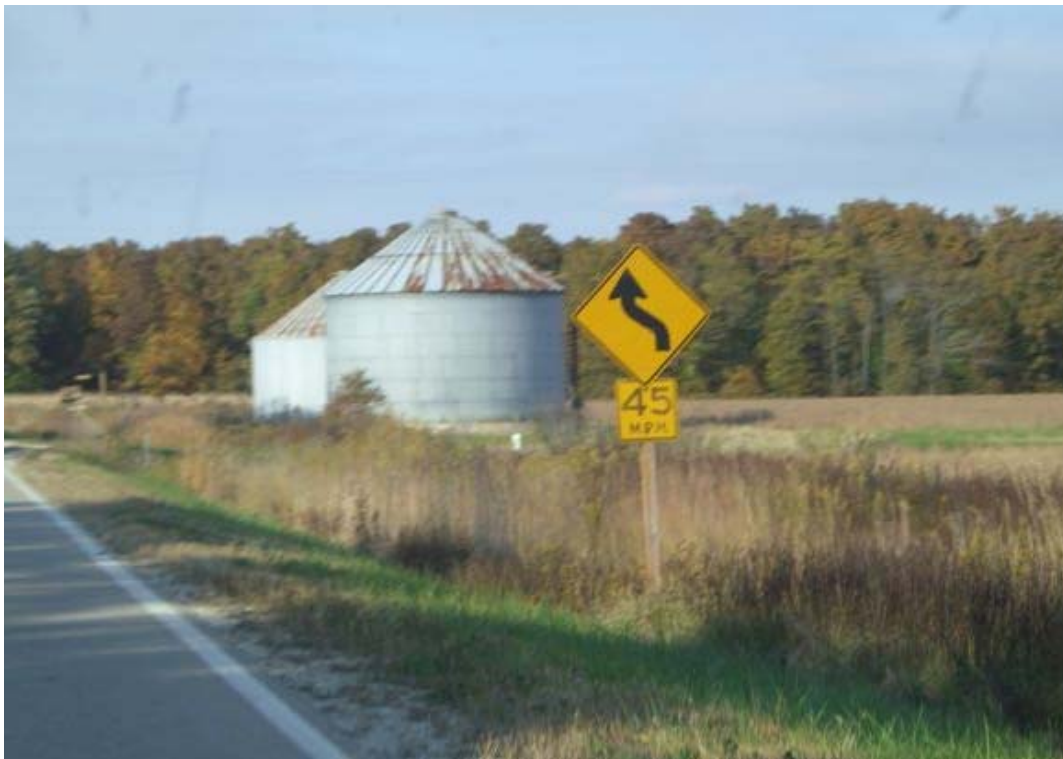
Figure A.12. County Road W-62, reverse curve sign and advisory speed plaque
