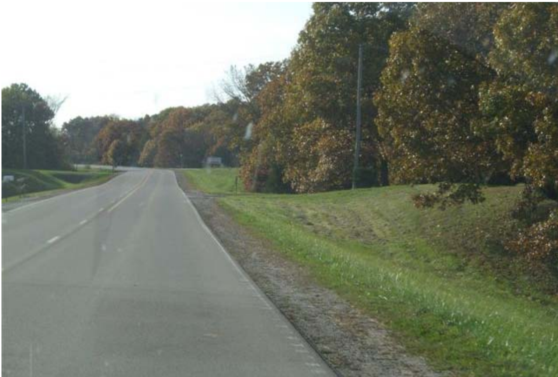
Figure A.8. County Road W-62, alignment and pavement markings
