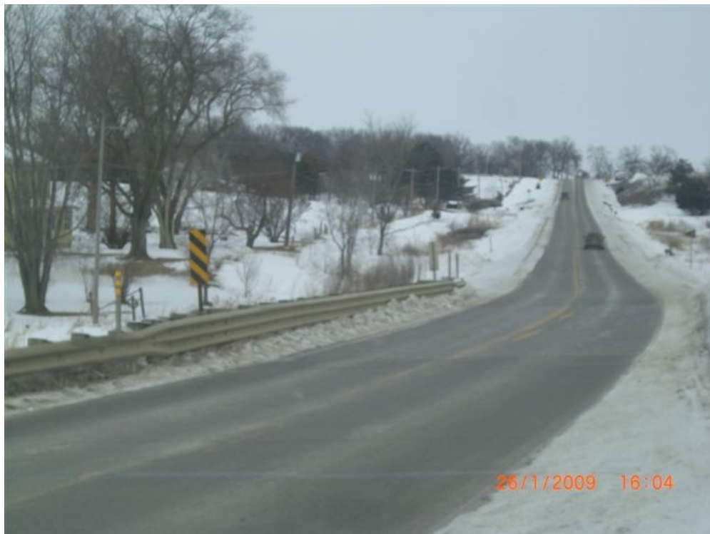
Figure C-2. Small bridge eastbound E-35 just east of Vine Avenue intersection
