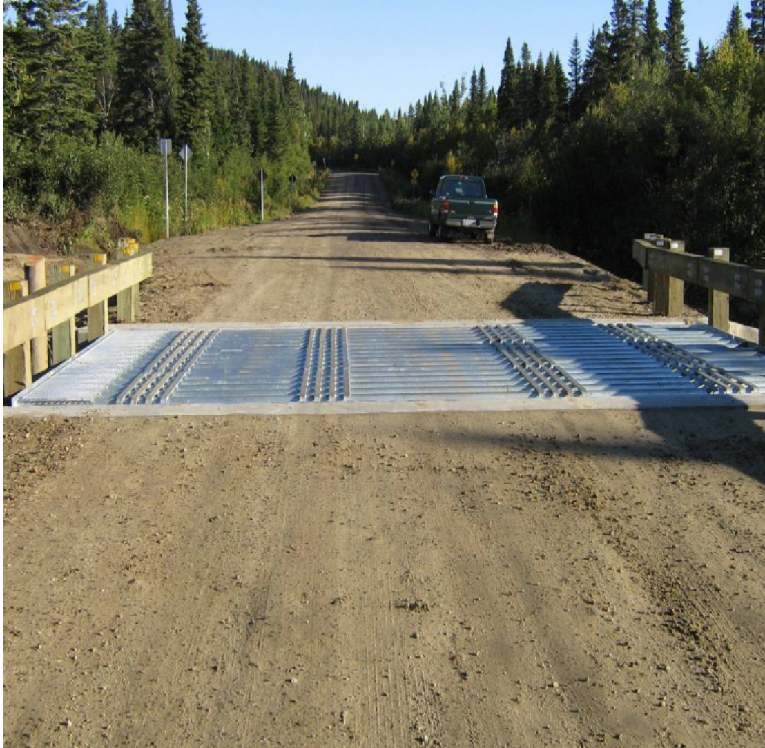
Figure B-2. Cattle gate across access road
