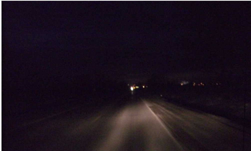
Figure C-8. Night view of E-35 showing painted pavement markings
