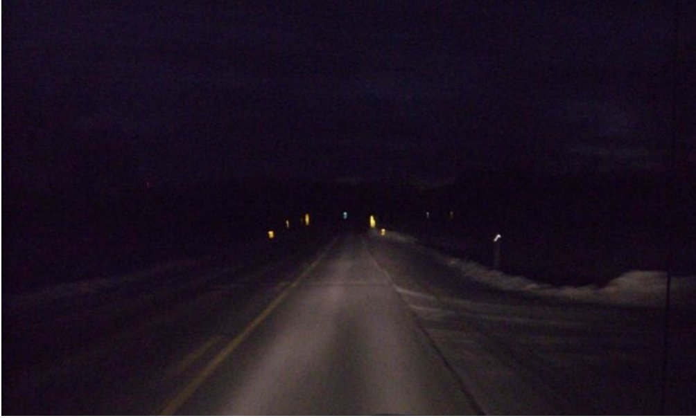
Figure C-11. Painted pavement markings and traffic control devices at night
