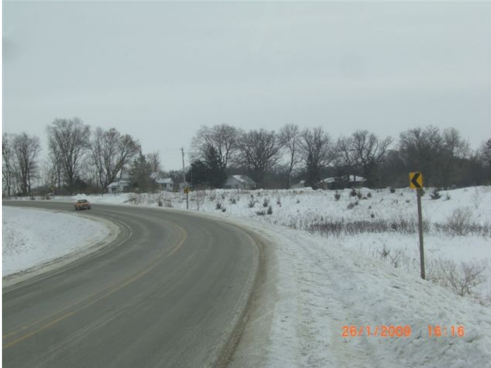
Figure C-5. Eastbound E-35 just south of Wallace Avenue intersection
