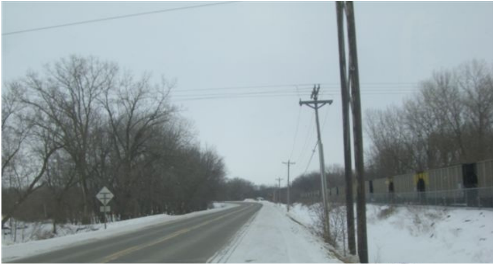
Figure C-1. Eastbound E-35 near beginning of review area
