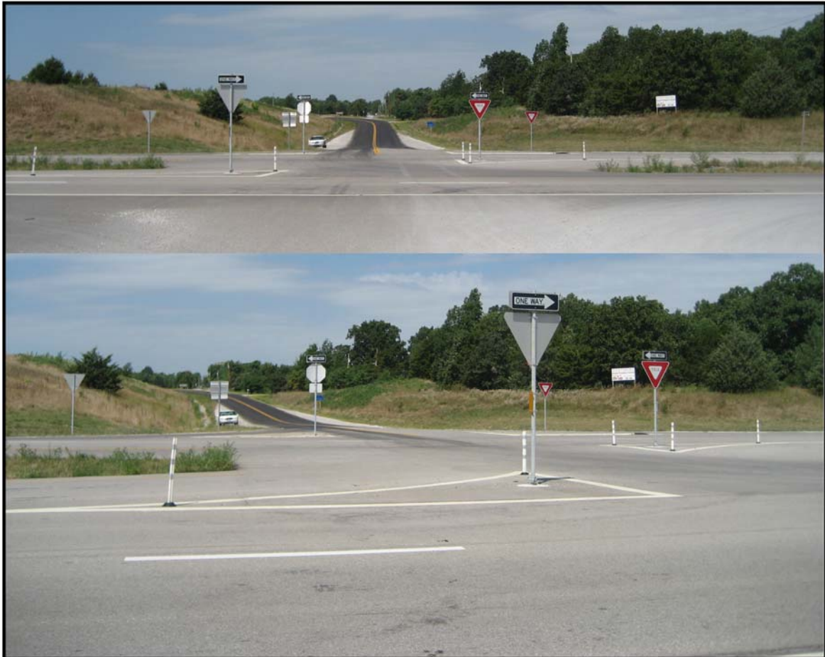
FIGURE 5: Pictures of MoDOT Median Channelization Islands with Delineators
