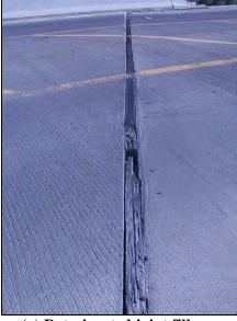
(a) Deteriorated joint filler (Bridge No. 2034.20035, District 5)
