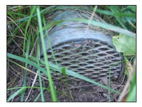
Figure 2. Example of a blocked subdrain outlet (Bridge No. 9266.2R218, District 5)
