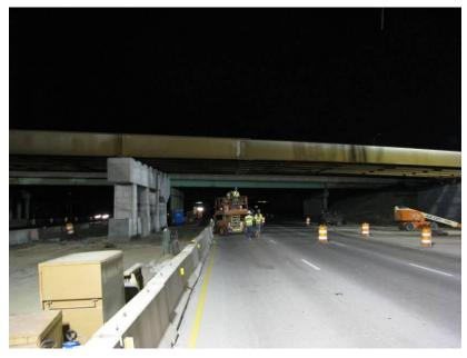
Figure 4.7. Construction workers performing bridge deck tie placement in Indiana
