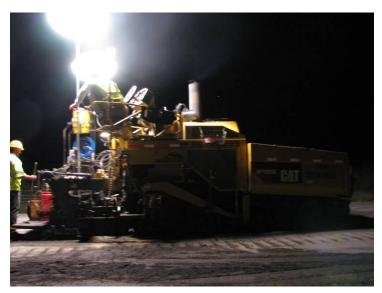
Figure 4.3. Milling and paving on SR 10 and I-66 using equipment-mounted balloon lighting
