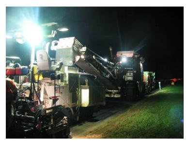
Figure 4.6. Milling and paving in New Jersey using equipment-mounted lighting
