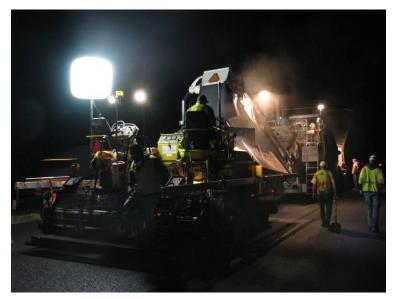
Figure 4.4. Mainline paving on SB I-55 using equipment-mounted balloon lighting
