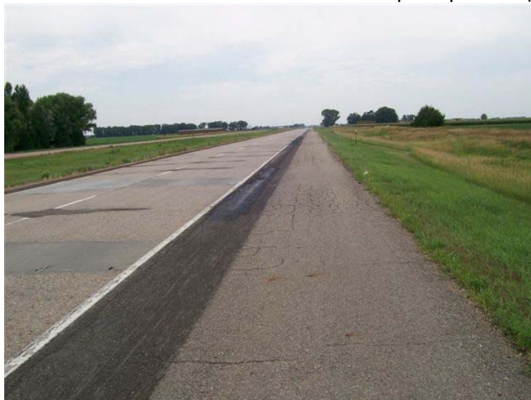
Figure 4 – Typical Existing Condition of SD Route 50 (westbound lanes looking west)
