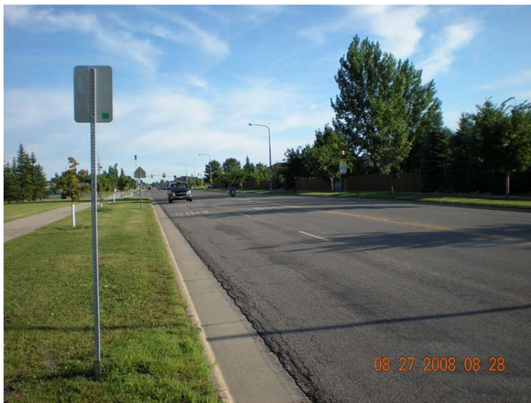
Figure 24 – Fargo, North Dakota; South 25 th Street Existing Condition
