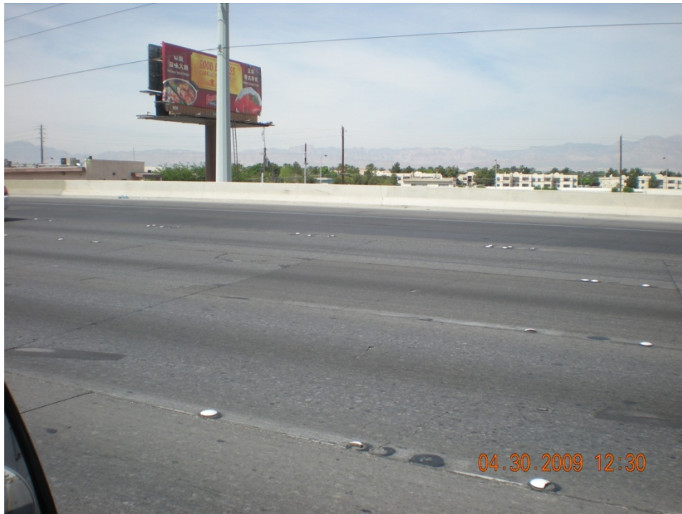
Figure 36 – Nevada I-15 Typical Pavement Condition Requiring Minimal Repair
