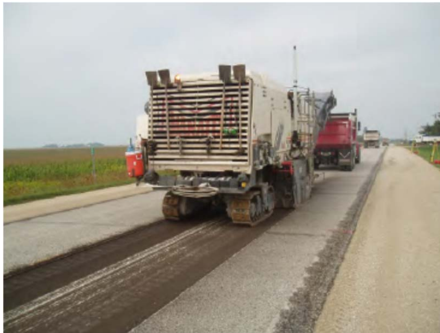
Figure 50 – Milling to Grade Using Automatic Machine Control
