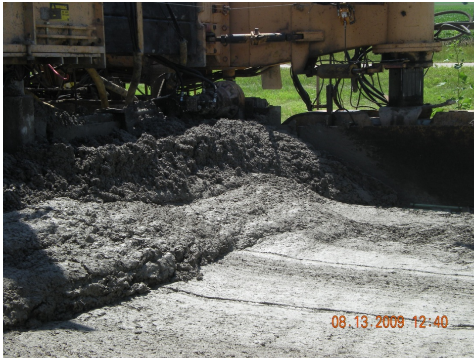
Figure 7 – SD Route 50 Concrete Head In Front of the Paver
