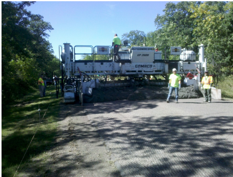
Figure 30 – Concrete Overlay Construction Near Devils Lake, ND
