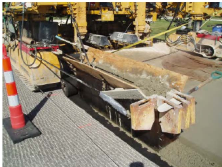
Figure 51 – Iowa US-18, Construction of the Temporary Safety Edge
