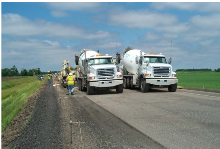
Figure 22 – North Dakota, Cass County Route 11 Concrete Overlay Construction
