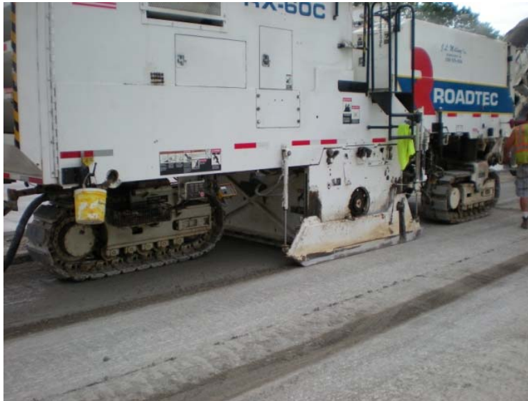
Figure 48 – Milling Concrete Prior to Placing a 4” Thick Unbonded Concrete Overlay
