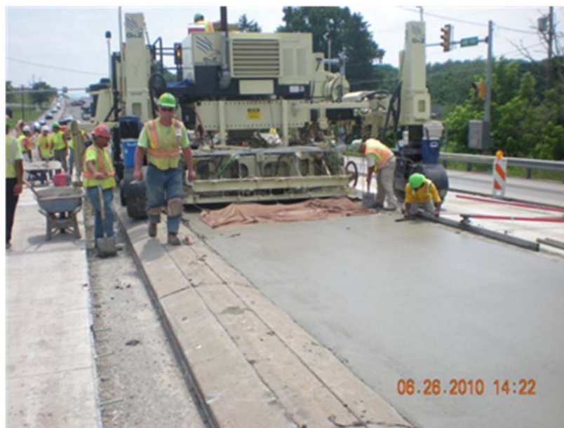
Figure 13 – Placement of the 6" Bonded Concrete Overlay on Pennsylvania SR-119
