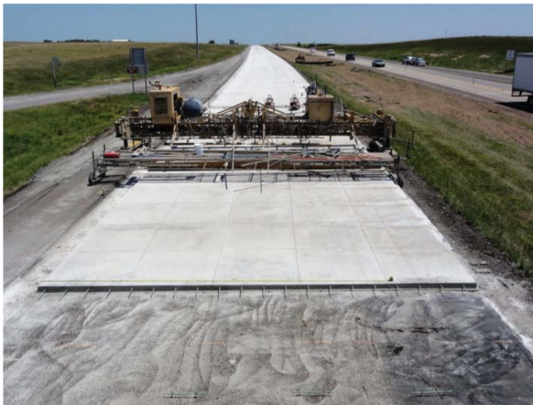
Figure 46 – Kansas, I-70 Bonded Overlay Construction
