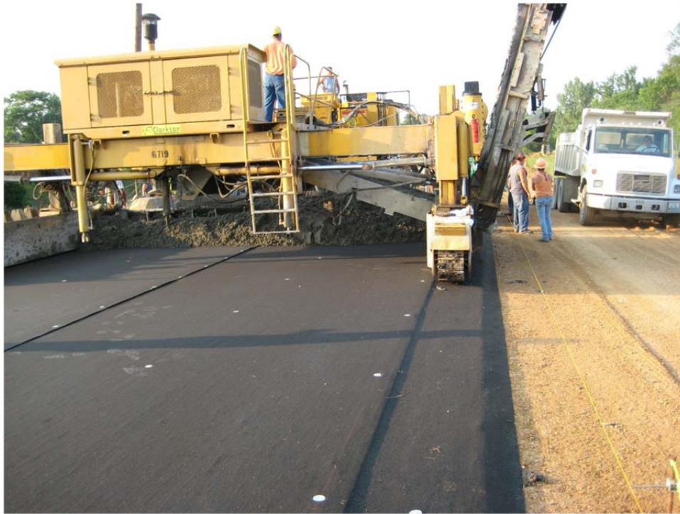
Figure 47 – Geotextile Separation Layer Used in Missouri
