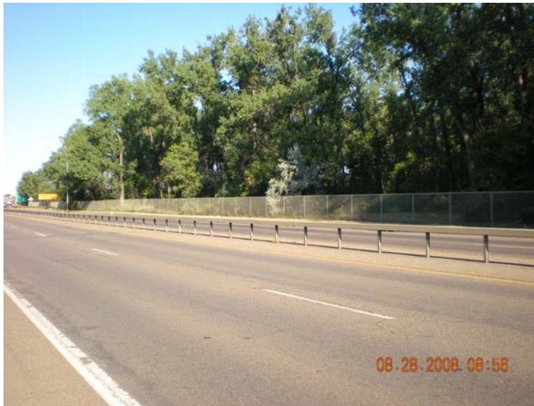
Figure 26 – Existing Conditions, Bismarck Expressway (ND)
