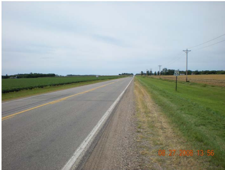
Figure 23 – North Dakota, Cass County Route 11 Existing Condition
