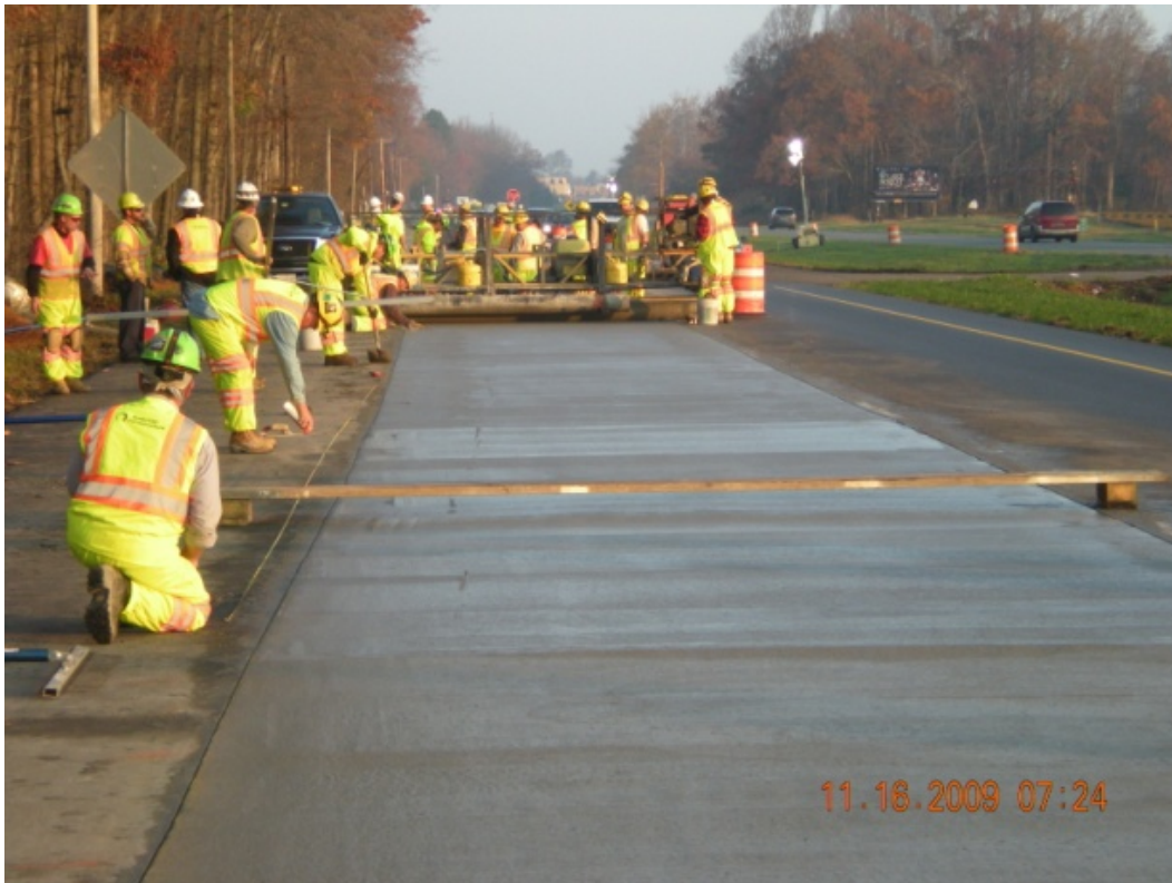
Figure 18 – US-13 Bonded Concrete Overlay Construction
