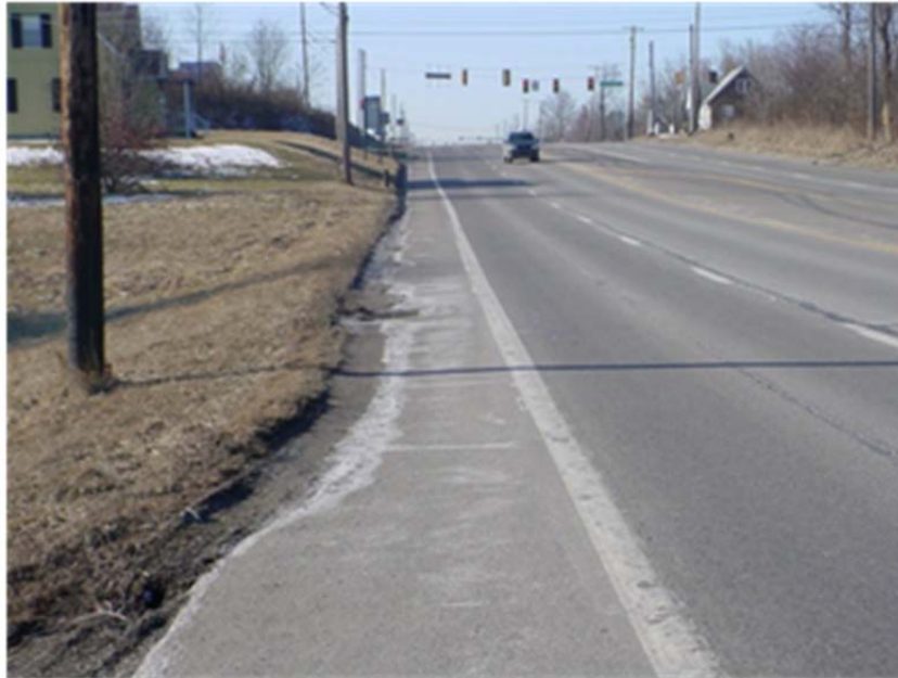
Figure 9 – Existing Condition of Pennsylvania SR-119 Looking South
