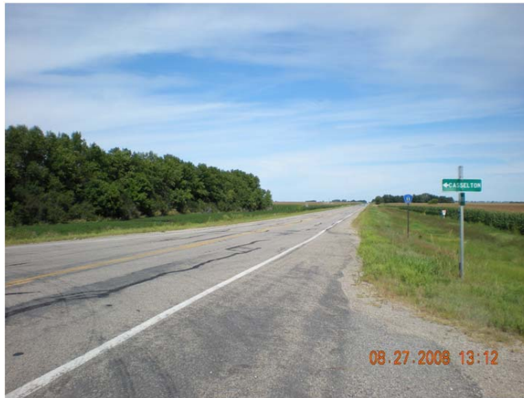
Figure 21 – North Dakota, Cass County Route 11 Existing Condition
