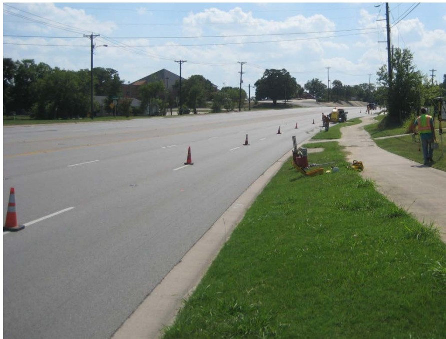
Figure 25. Site overview FM 1709 Fort Worth, Texas
