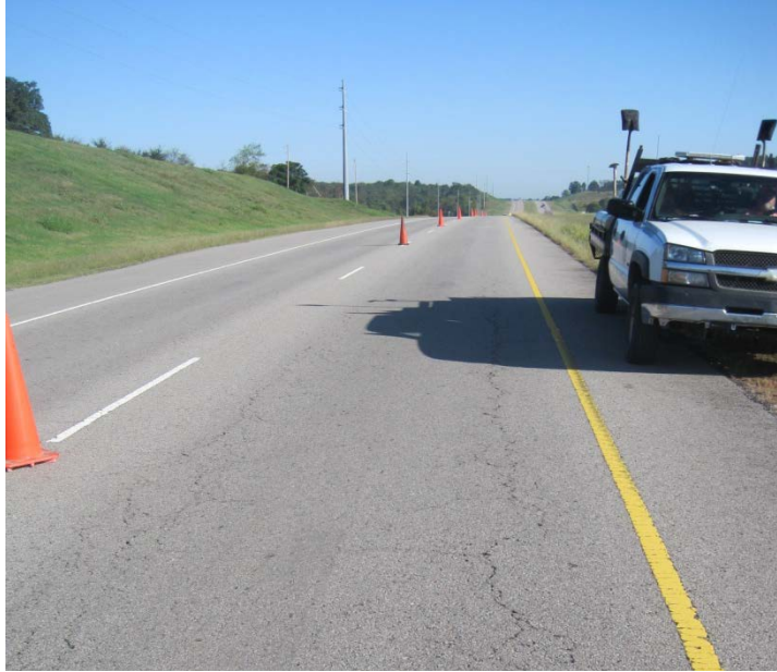
Figure 85. Site overview US 59 Le Flore County, Oklahoma
