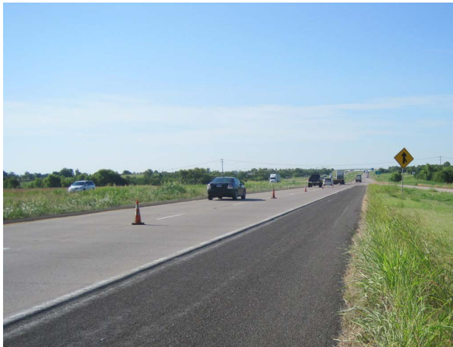
Figure 37. Site overview US 287 Mansfield, Texas
