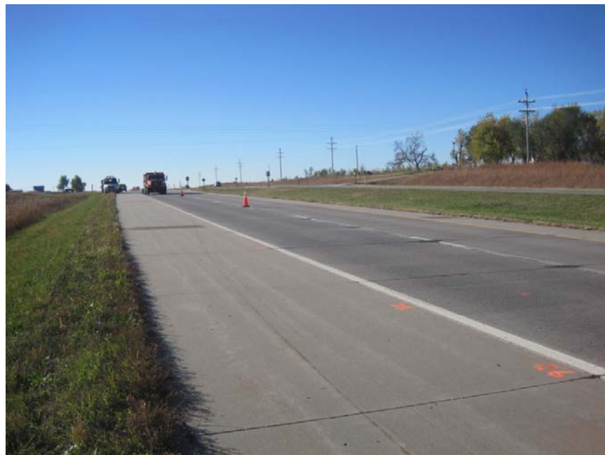
Figure 115. Site overview US 75 NB Jackson County, Kansas
