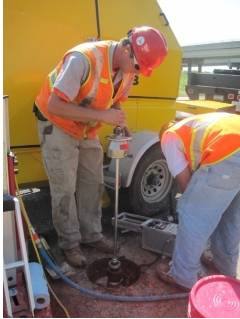
Figure 3. Light weight deflectometer test
