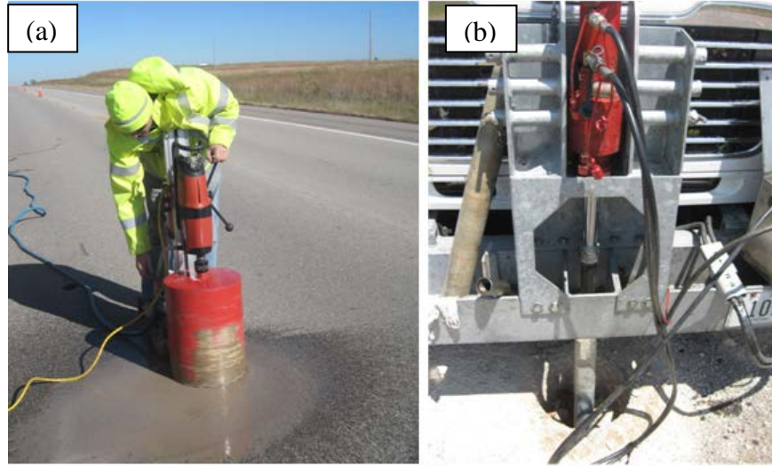
Figure 5. (a) Paving coring (b) collecting of undisturbed Shelby tube sample
