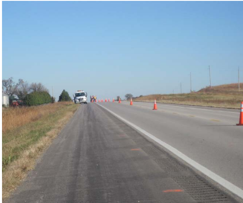
Figure 97. Site overview south bound lane US 75 Osage County, Kansas
