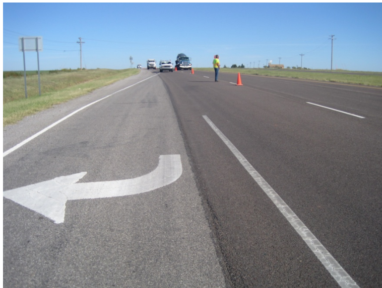
Figure 53. Site overview US 183 Clinton, Oklahoma
