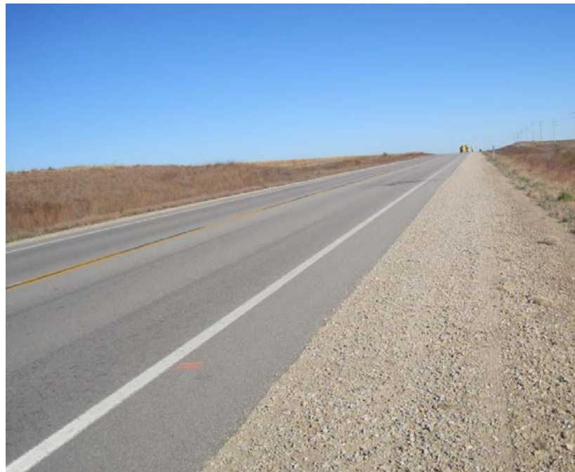
Figure 131. Site overview K 7 NB Doniphan County, Kansas
