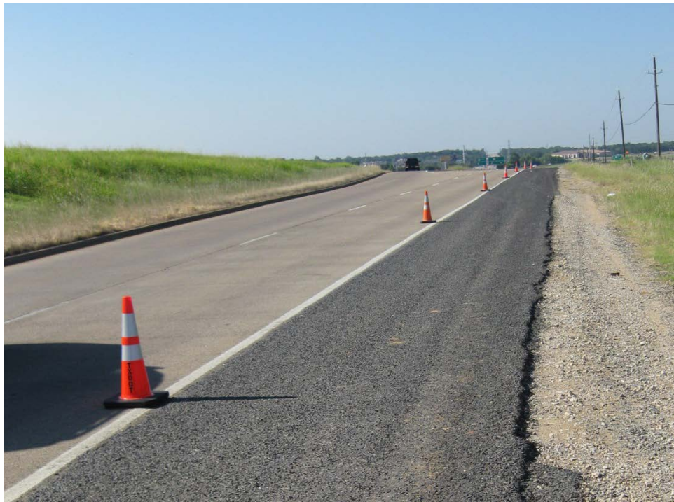
Figure 12. Site overview SH 121 Fort Worth, Texas
