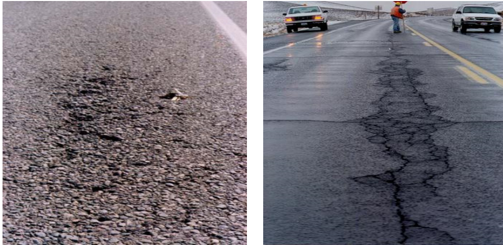
Figure 2.11. A Pictorial View of Raveling
