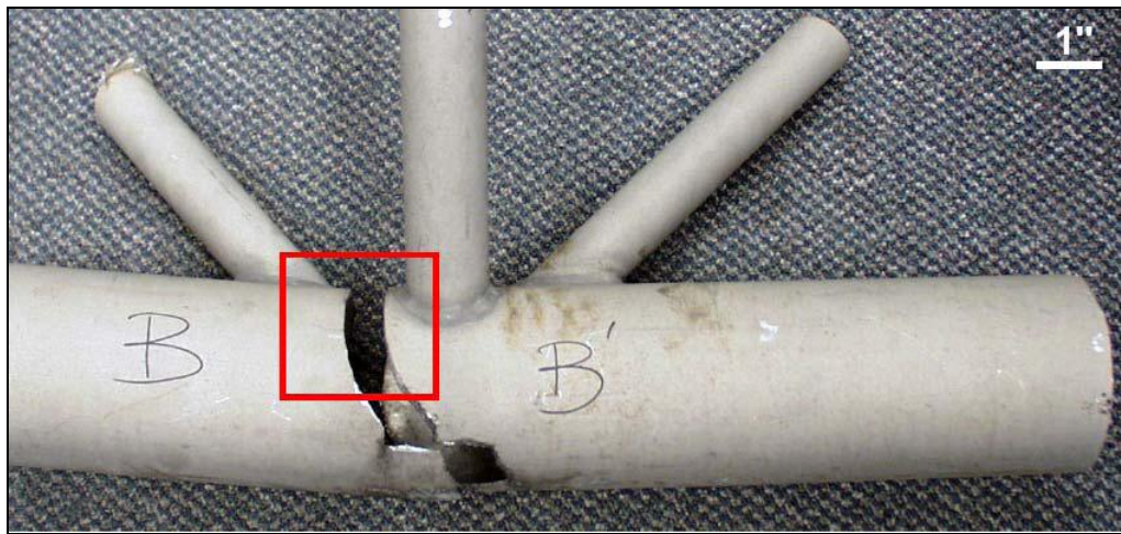
b) Crack at welding heat zone
