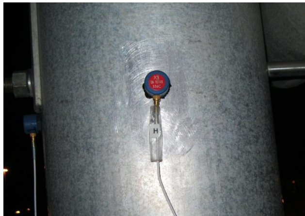
Fig. 29 View of an accelerometer attached to a truss member
