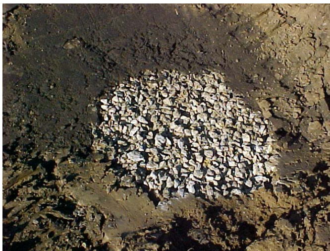
Figure 23. Geopier Construction Operations
