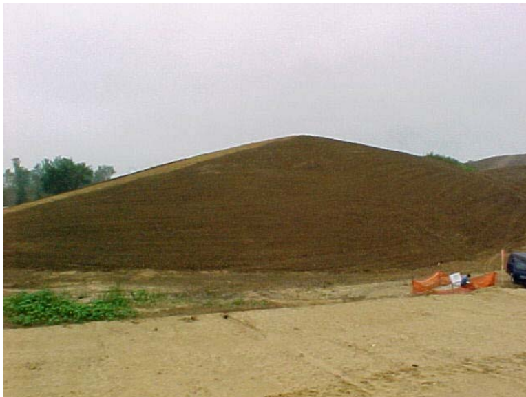
Figure 12. Ramp B Stone Column Supported Embankment
