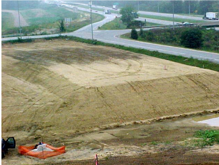
Figure 11. Ramp C Geopier Supported Embankment
