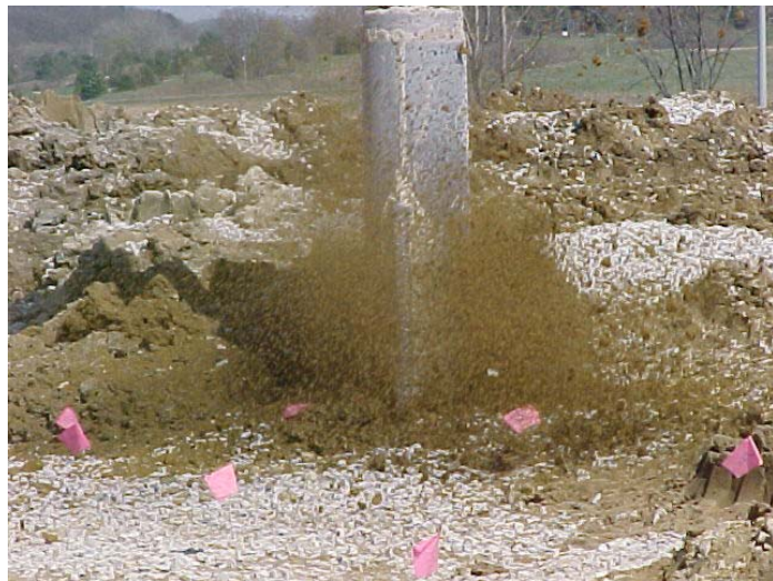
Figure 17. Stone Column Construction Operations
