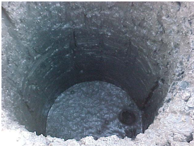
Figure 76. Wet Conditions during Piezometer Borehole Installation and Geopier Construction
