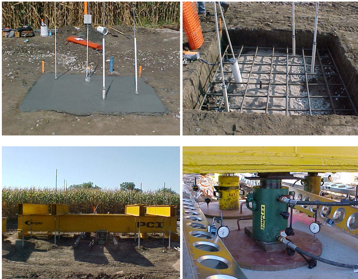
Figure 67. Group Load Test No. 1 Construction and Load Frame
