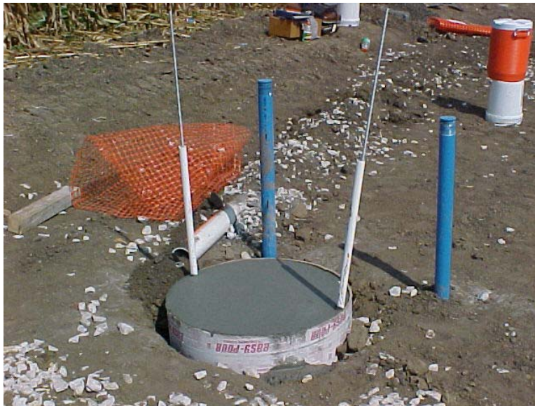
Figure 54. Test Pier No. 1
