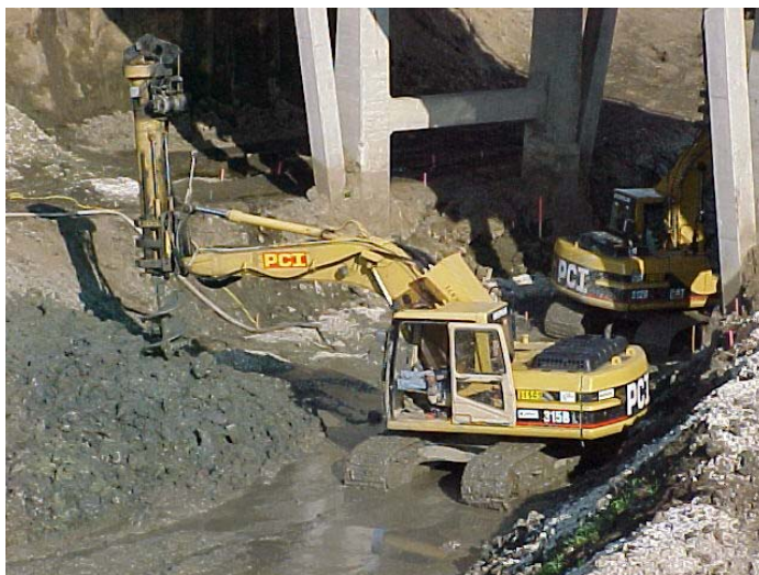
Figure 41. Project Site and Grading Operations for Box Culvert
