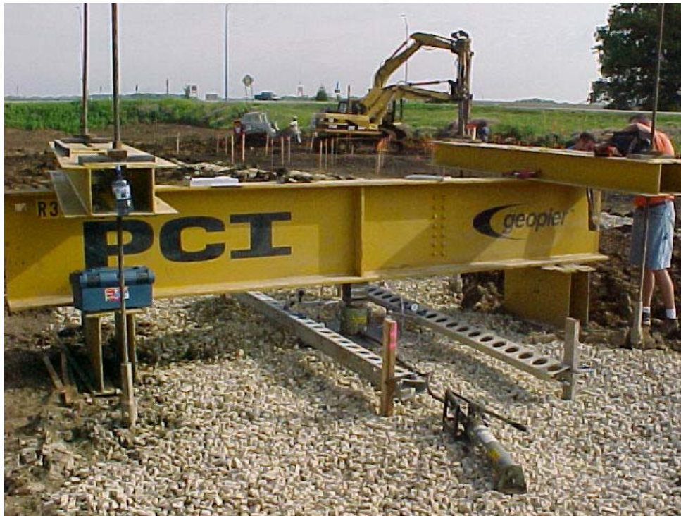
Figure 30. Geopier Field Modulus Load Test
