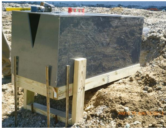
Figure 47. Weir box with base and supports
