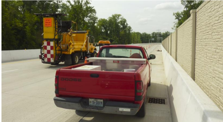
Figure 53. Traffic safety in place during sampling with truck-mounted TMA
