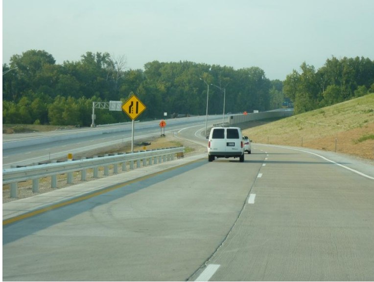
Figure 35. Operating Highway 141 perspective along southbound Olive Road ramp
