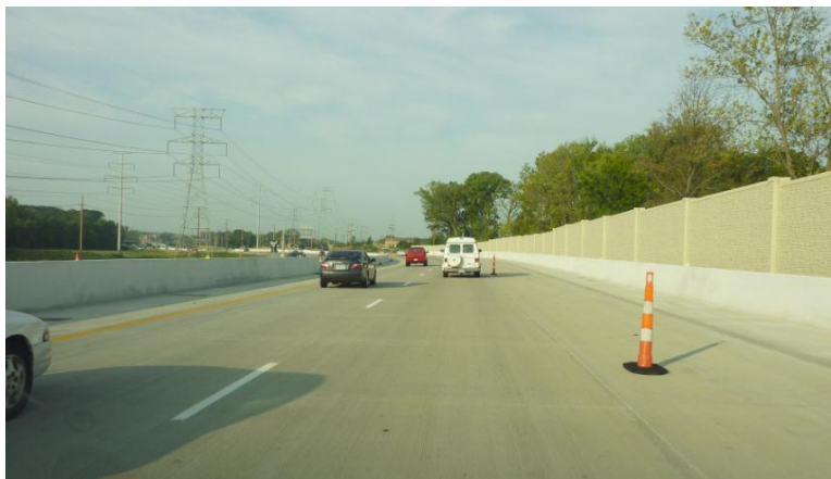
Figure 36. Operating Highway 141 perspective within TX Active paving zone and showing adjacent crash barrier and sound wall
