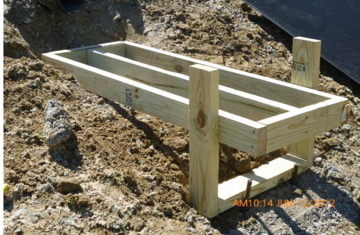
Figure 46. Base for weir box
