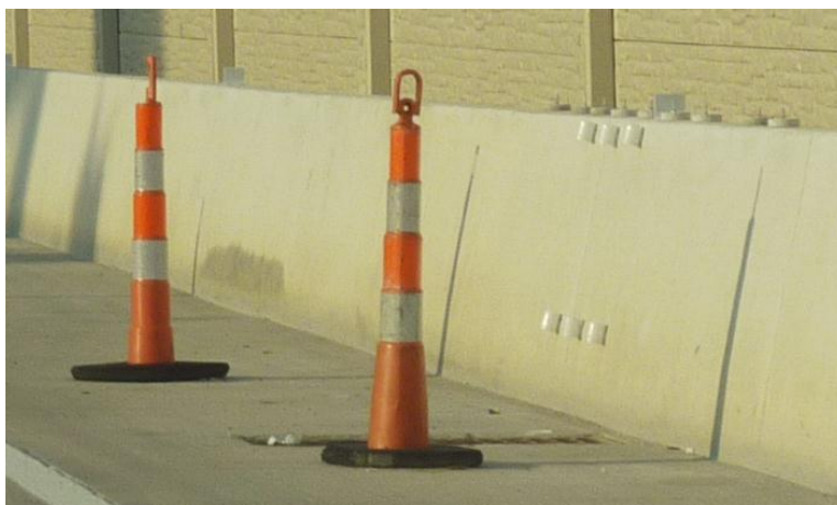
Figure 18. Ogawa analyzers mounted on adjacent crash barrier wall (i.e., including three upper and three lower samplers per each location)
