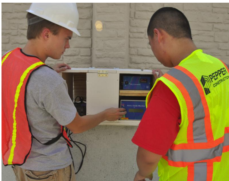
Figure 20. On-site use of Active NO x 2B Technologies instrumentation
