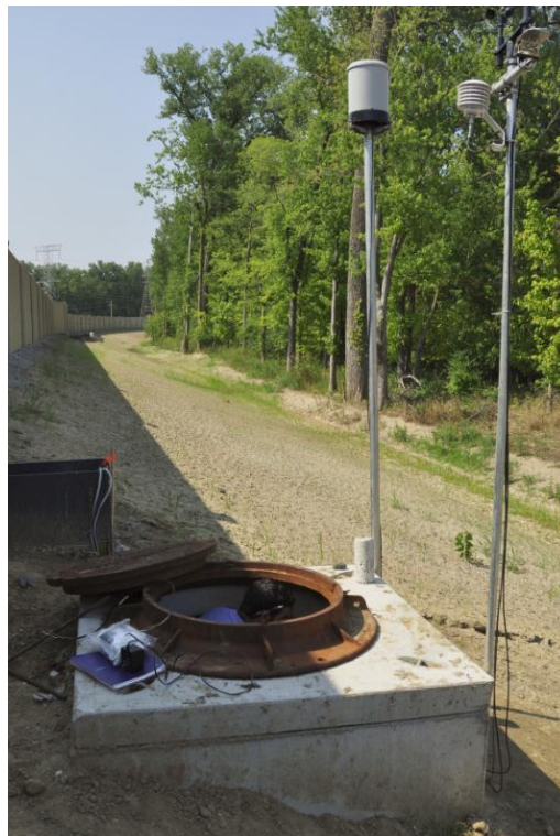
Figure 28. Sensor vault and temporary weather station installation
