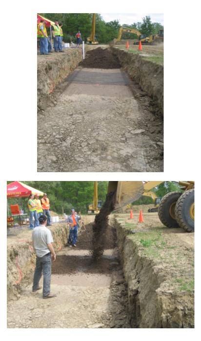
Figure 47. Placement of biaxial Geogrid in TB 1
