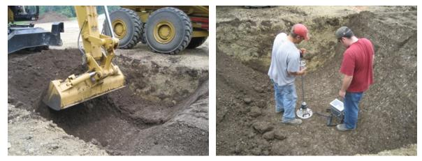
Figure 86. Process of excavation to the top of each underlying lift to perform LWD testing
