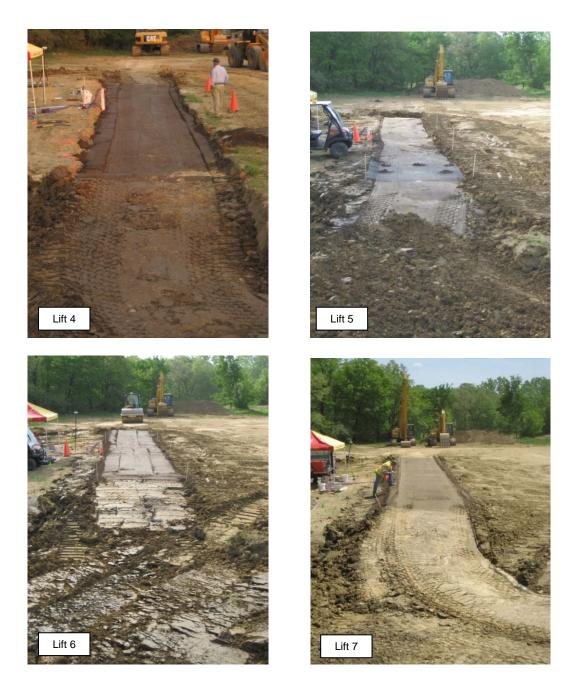
Figure 46. Lifts 4 to 7 of CA6-G material placed in TB 1
