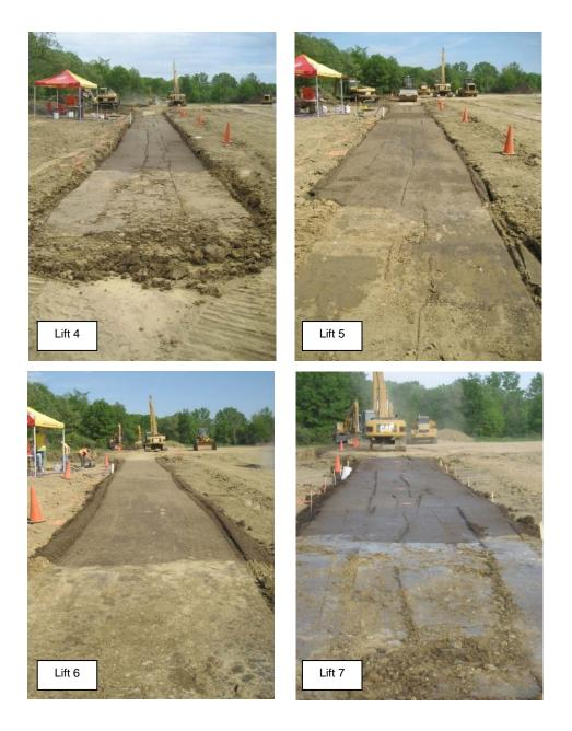
Figure 68. Lifts 4 to 7 of CA6-G material placed in TB 2
