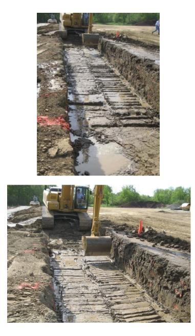
Figure 66. Preparation of wet subgrade portion of TB 2
