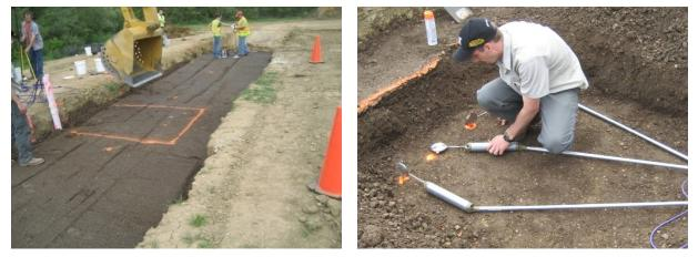
Figure 13. Excavation to install EPC's (left) and installation of EPC's in orthogonal directions
