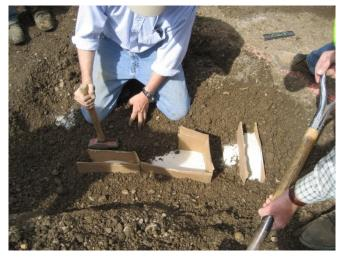
Figure 16. Placement of sand (~ 2 in) around the EPCs
