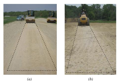
Figure 20. (a) Strip 1 – CS-563 and CS-683 smooth drum rollers (CMV, RMV) – hard unsurfaced aggregate road, (b) Strip 2 – CP-563 padfoot roller (MDP, CMV, and RMV) – hard compacted glacial till subgrade
