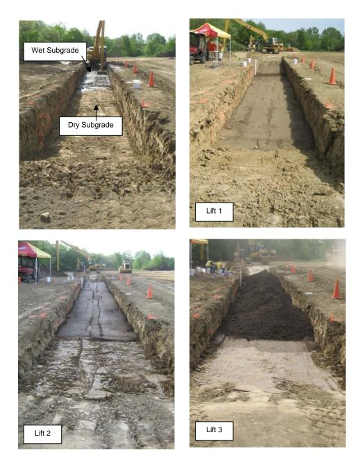
Figure 67. Wet/dry subgrade and lifts 1 to 3 of CA6-G material placed in TB 2
