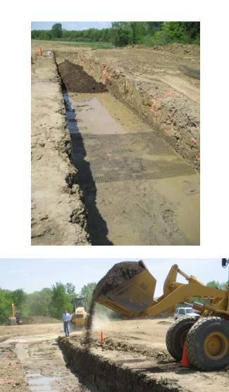
Figure 69. Placement of geogrid layer on soft subgrade
