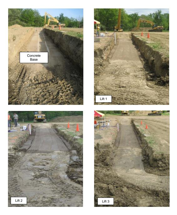
Figure 45. Concrete base and lifts 1 to 3 of CA6-G material in TB 1
