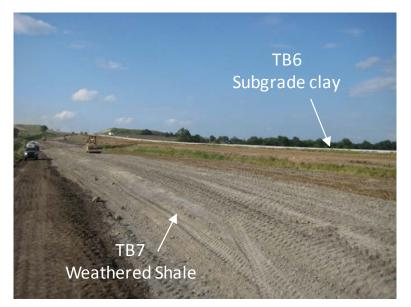
Figure 48. Picture showing TBs 6 and 7
