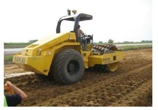
Sakai SV610 padfoot roller used for compaction
