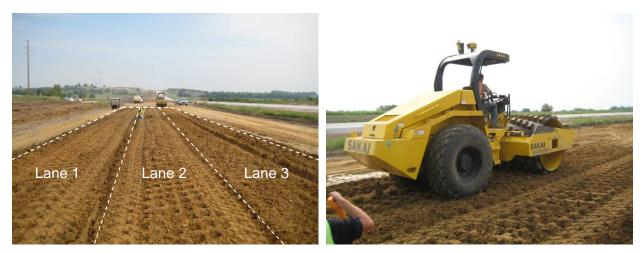
Figure 25. Photographs showing construction and setup of lanes for compaction and testing on TB4 subgrade clay material
