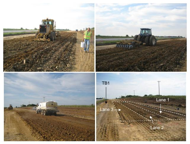
Figure 17. Photographs showing construction process and test bed layout – TB 2 lanes 1, 2, and 3 subgrade clay material (TB1 shown for reference)
