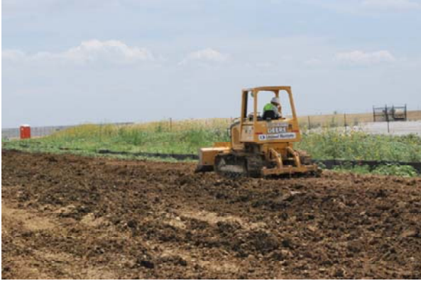
Subgrade scarification using grader
