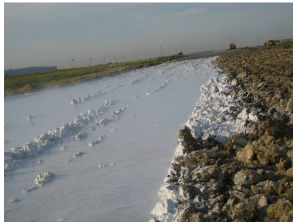
Figure 25. Picture showing ponding of lime slurry on the scarified subgrade (picture taken 07/21/2008)
