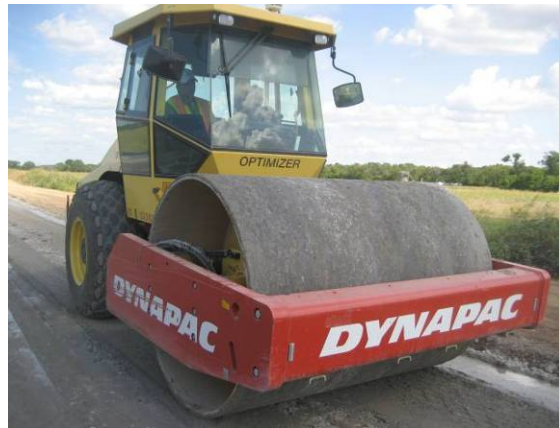
Figure 4. CA-362 smooth drum roller used on the project
