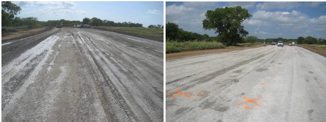
Figure 39. Moisture on flex base material during compaction (TB 6 left) and a day after compaction (TB 7 right)
