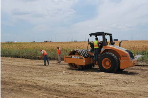
Compaction using Case/Ammann padfoot roller
