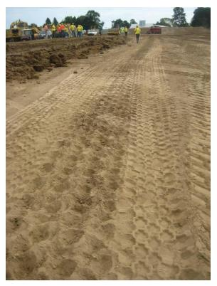
Figure 30. TB5 cohesive embankment fill test strip
