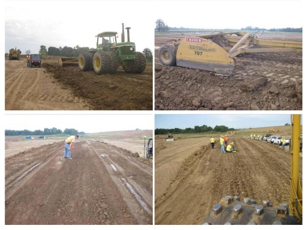
Figure 23. Construction of TB4 silty clay subgrade calibration test strips
