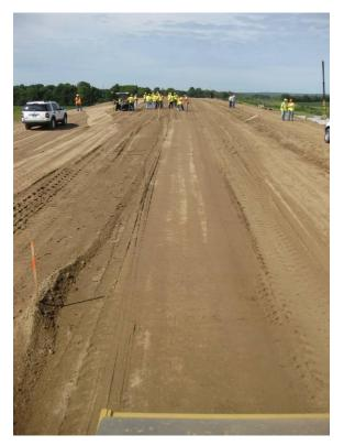
Figure 10. TB1 granular embankment fill calibration test strips
