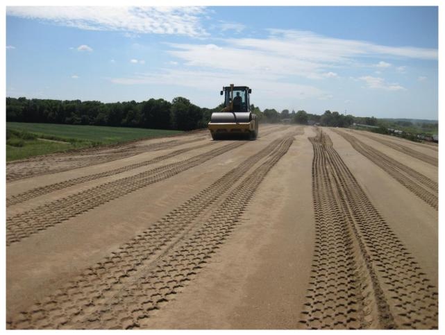
Figure 32. TB6 granular embankment fill production area lift # 2
