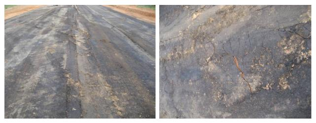
Figure 18. Cracks observed on the treated base material following the Sakai vibratory roller pass – TB2
