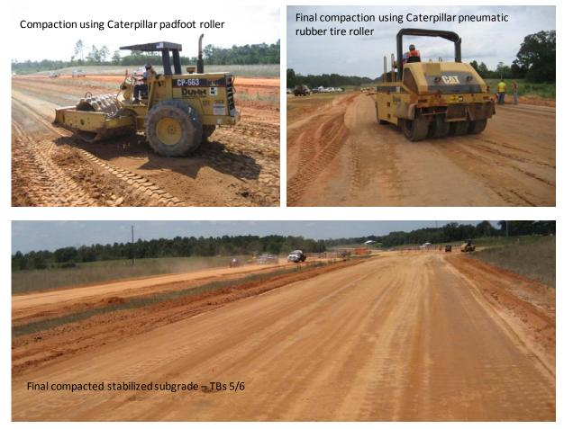
Figure 39. Pictures showing construction process and final compacted surface on TBs 5/6 treated subgrade
