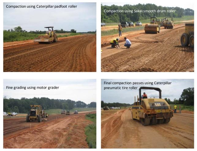
Figure 21. Pictures showing construction process on TB3 treated base
