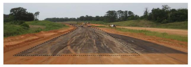
Figure 14. Picture of the test bed – TB2 treated base material
