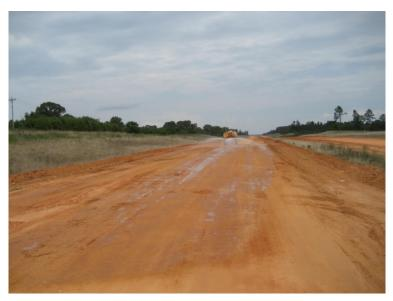
Figure 31. TB4 compacted granular subgrade material
