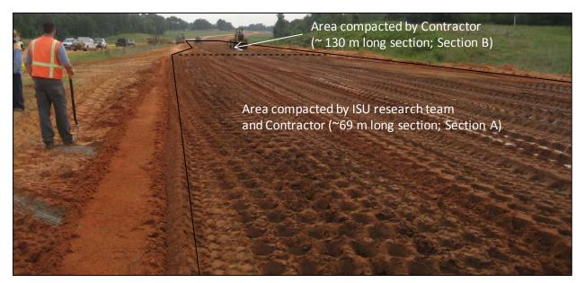
Figure 19. TB3 treated base material compacted by ISU research team (section A) and contractor (section B)
