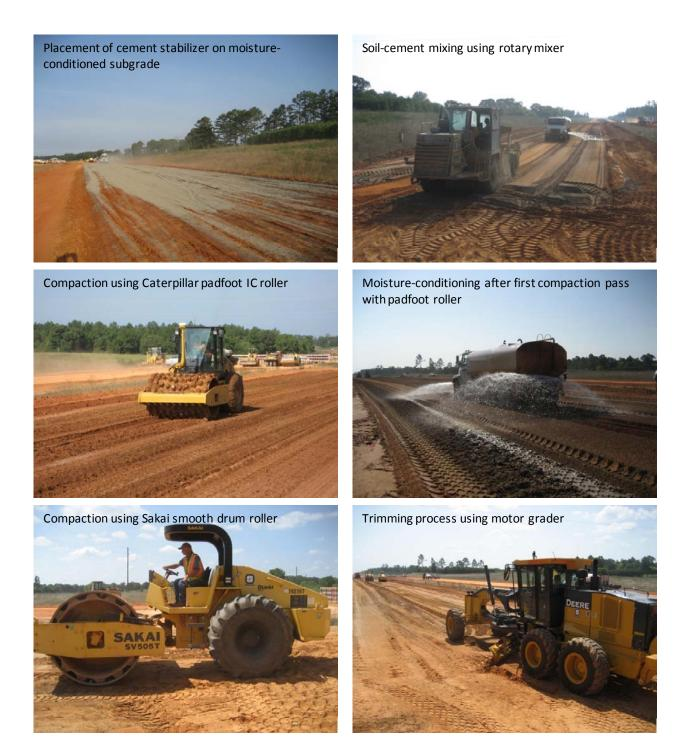
Figure 38. Pictures showing construction process on TBs 5/6 treated subgrade
