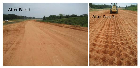
Figure 10. TB1 granular base material after pass 1 with Sakai smooth drum roller (left) and pass 3 with Caterpillar padfoot roller (right)
