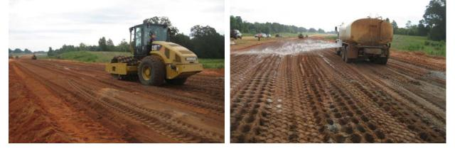
Figure 20. Pictures showing construction process on TB3 treated base
