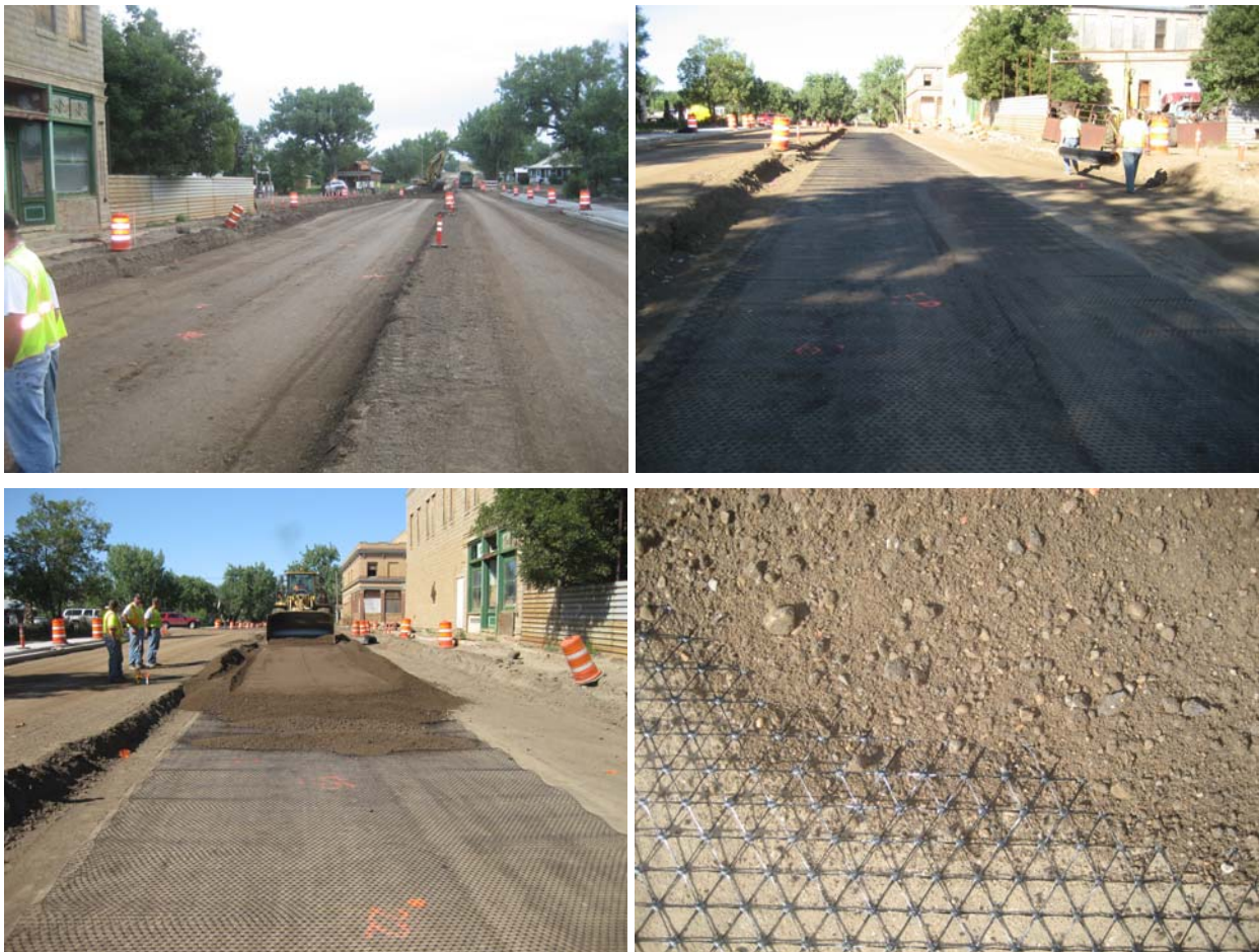
Figure 43. Photographs of TB4 during placement of TX5 geogrid and salvage base layers and
