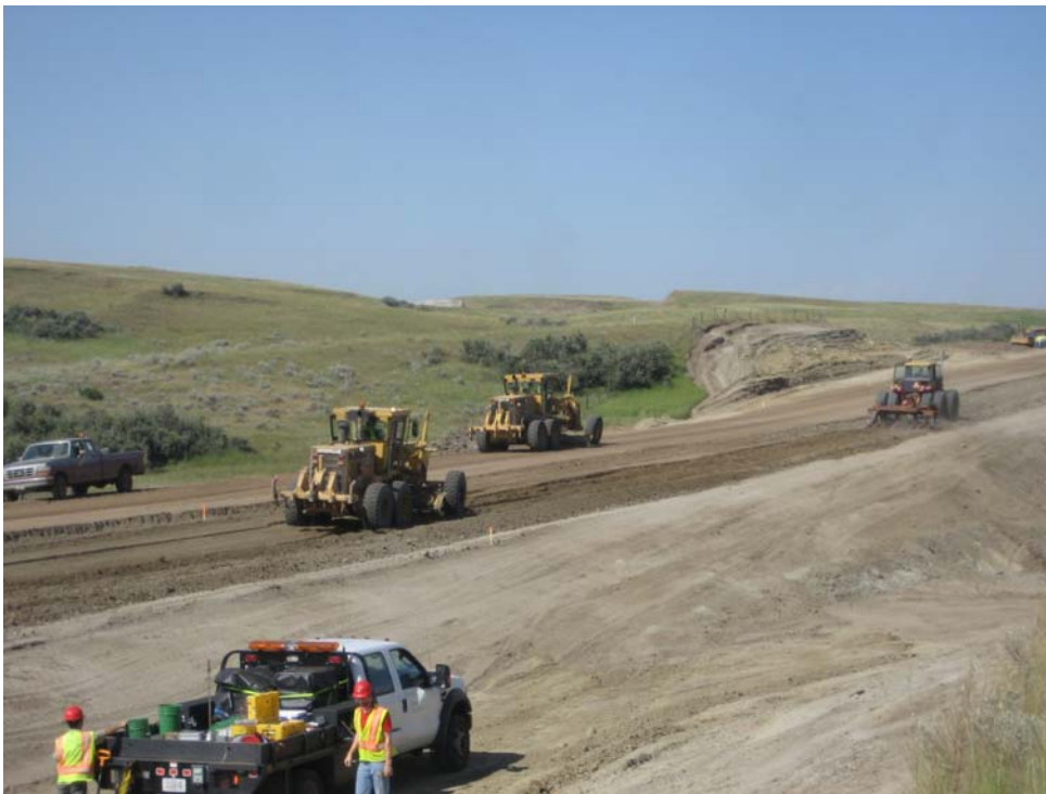
Figure 12. Photographs of construction and testing of TB1
