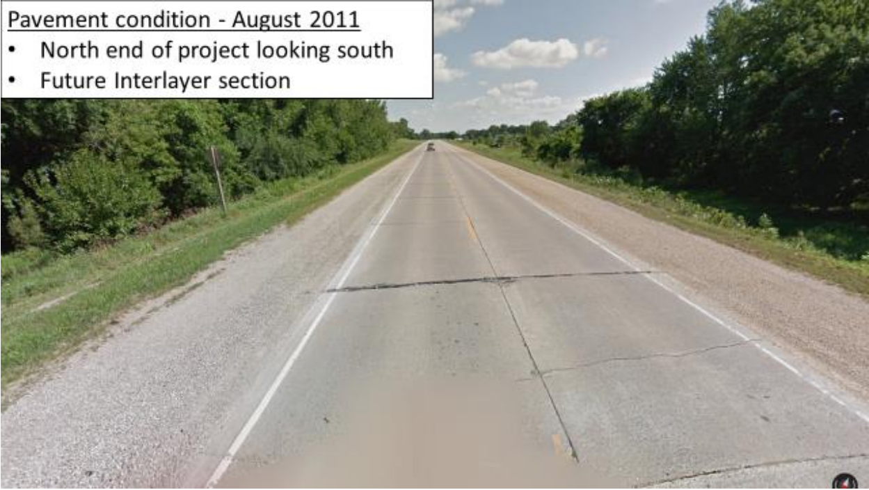
Figure 10. Pre-construction view of interlayer overlay section on US 169
