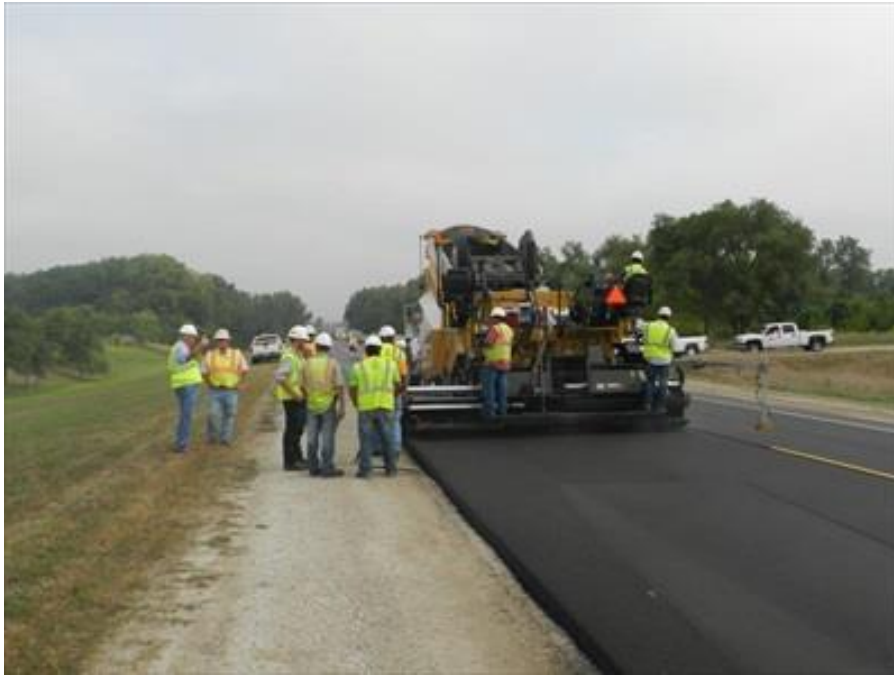
Figure 5. Interlayer paving on US 169
