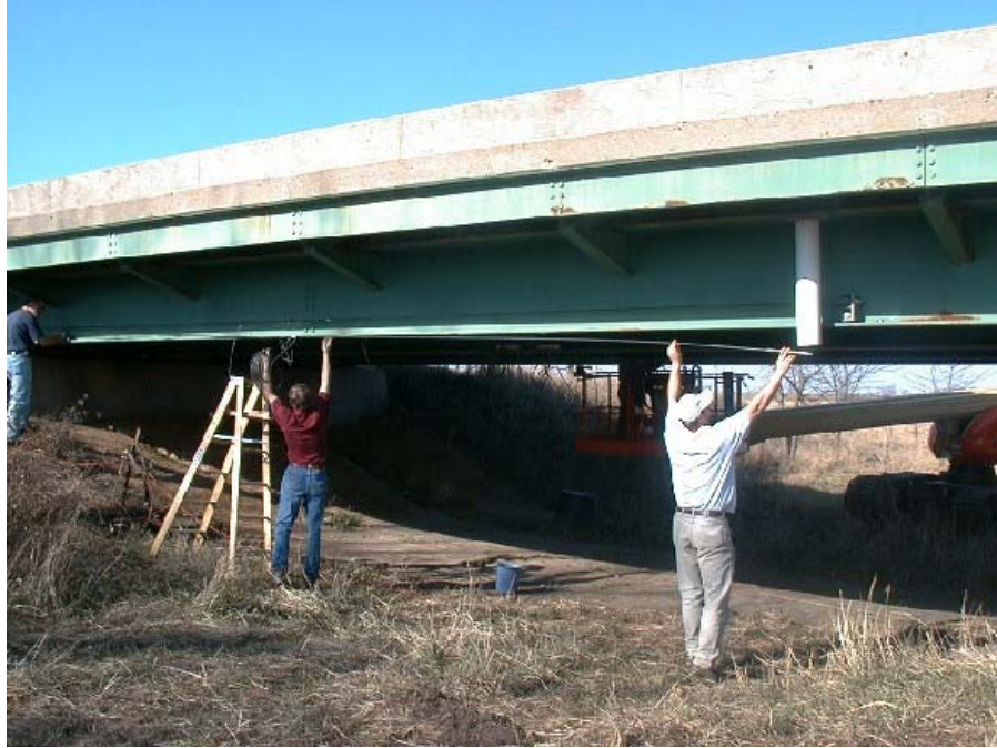
(a) Placement of a CFRP bar
