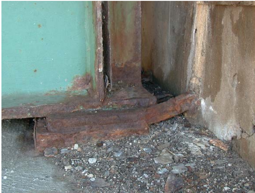
(d) Typical east abutment condition
