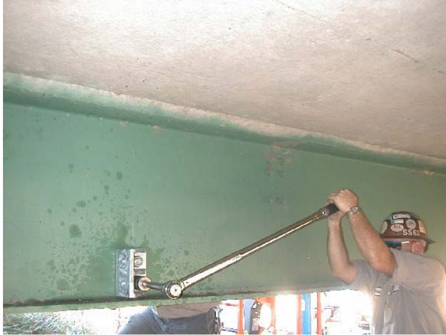
Figure 5. Installing anchorage assembly.
