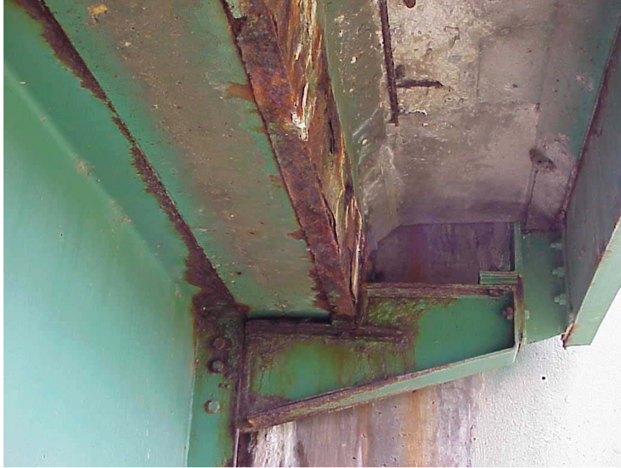
(e) Typical condition of deck soffit and deck channel
