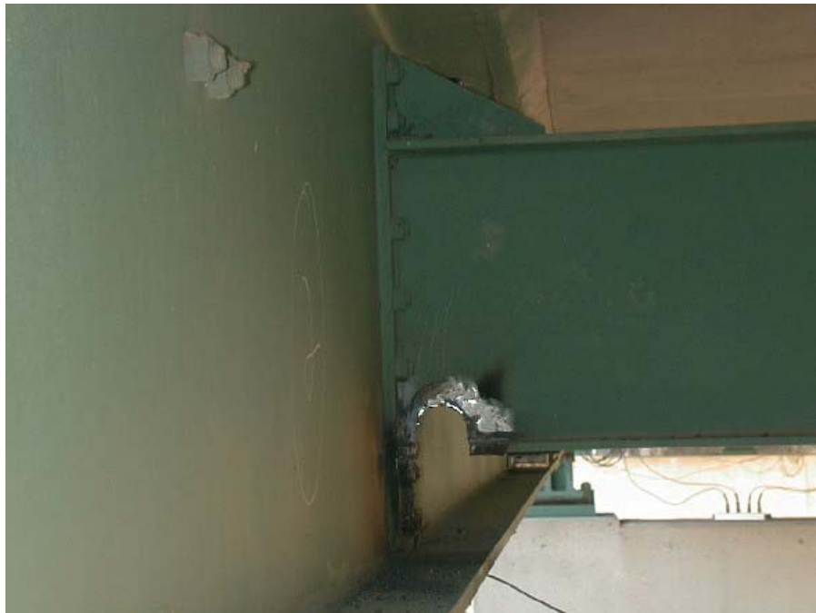
Figure 6. Removal of a portion of the diaphragm/stiffener assembly.
