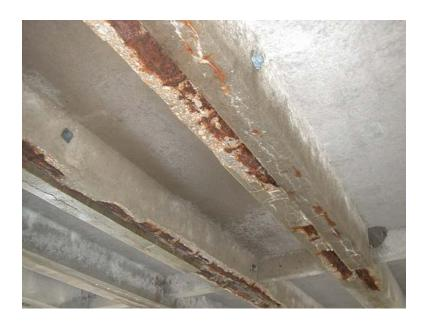
**FIGURE 4. Typical PCB Deterioration**
