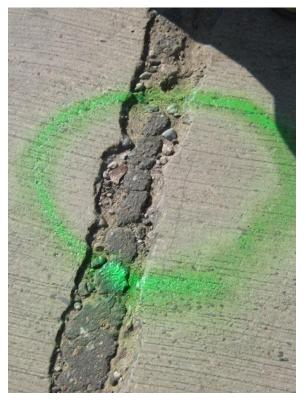
Figure 1. Crack formed about 1 in. from the free surface
