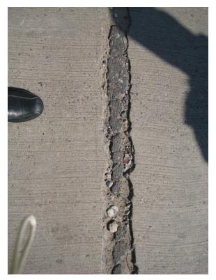
Figure 2. Distress in transverse joint
