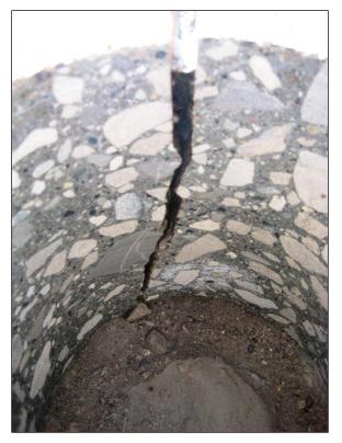
Figure 3. Faulting and loss of aggregate interlock
