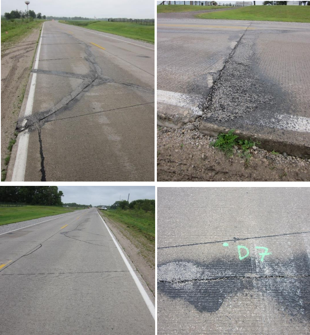
Figure 46. Photographs of field test site during testing — E63, Story County
