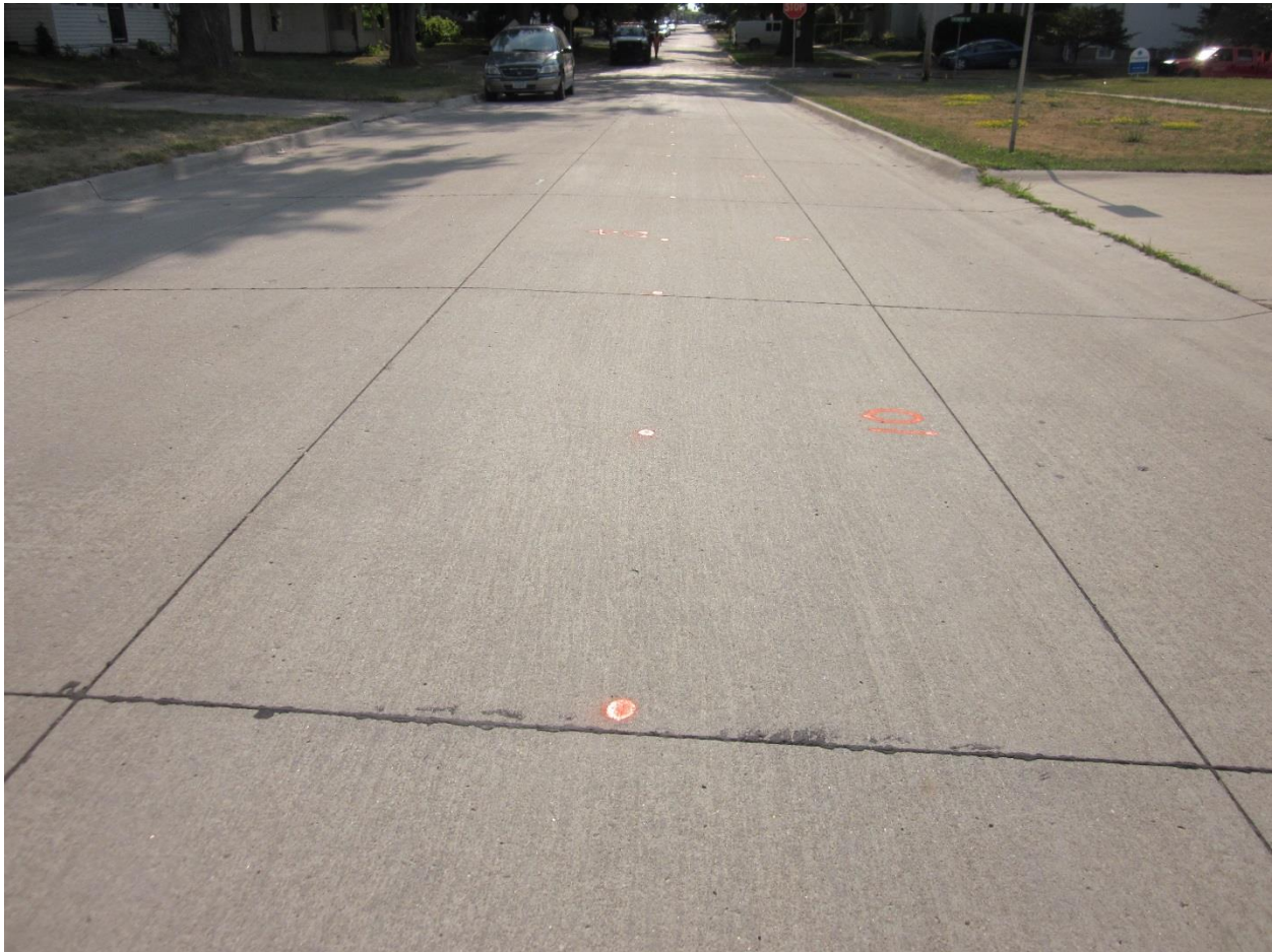
Figure 81. Photographs of field test site during testing — West Main Street, Knoxville
