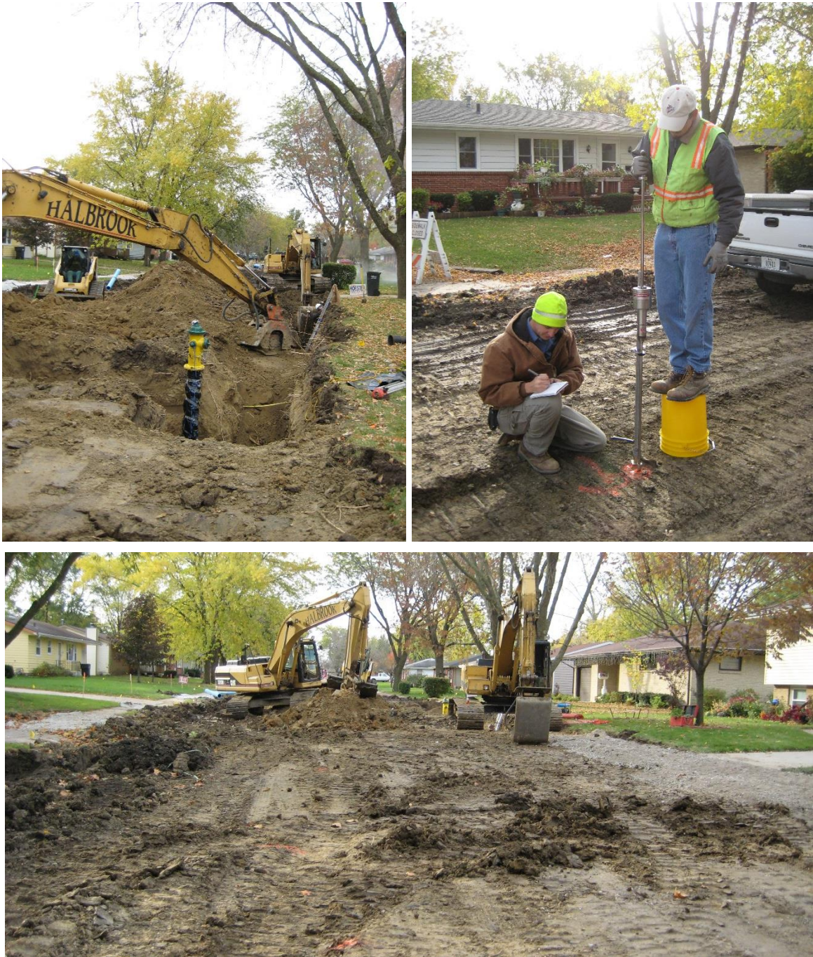
Figure 74. Photos during construction and testing in 2008 — SW Westlawn Drive, Ankeny
