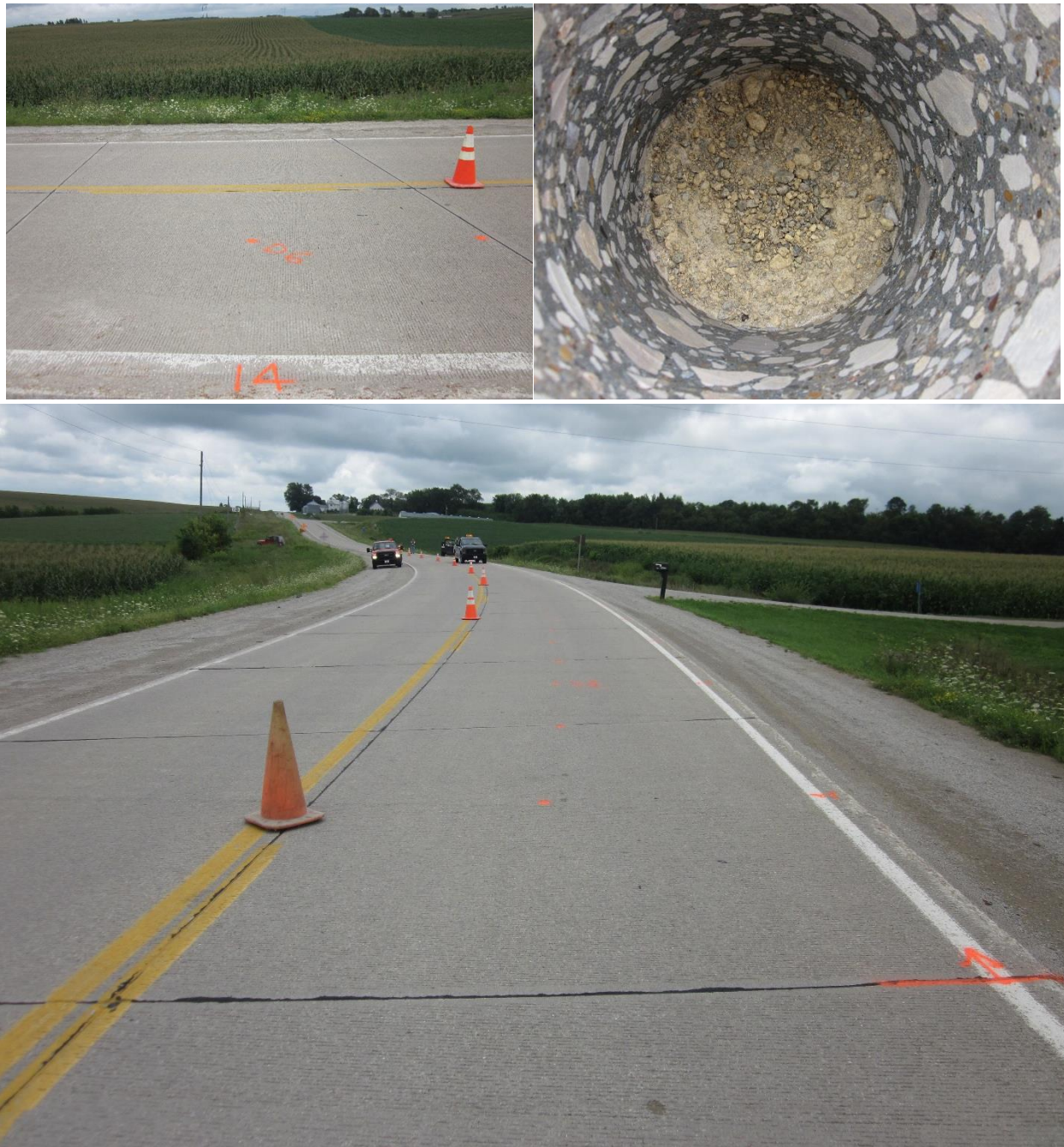
Figure 123. Photographs of field test site during testing — W38/Locust Road, Winneshiek County
