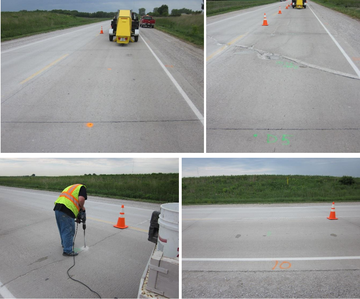
Figure 53. Photographs of field test site during testing — Riverside Road, Ames
