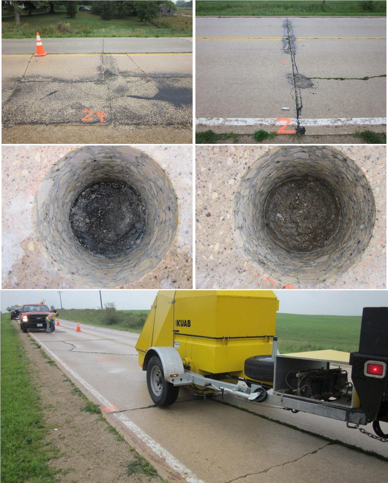
Figure 128. Photographs of field test site during testing — 175 th Street, Winneshiek County
