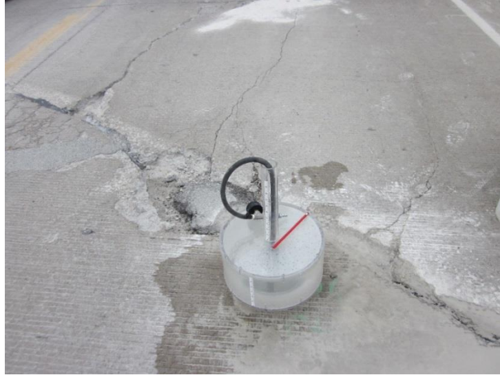
Figure 18. Core hore permeability testing in situ
