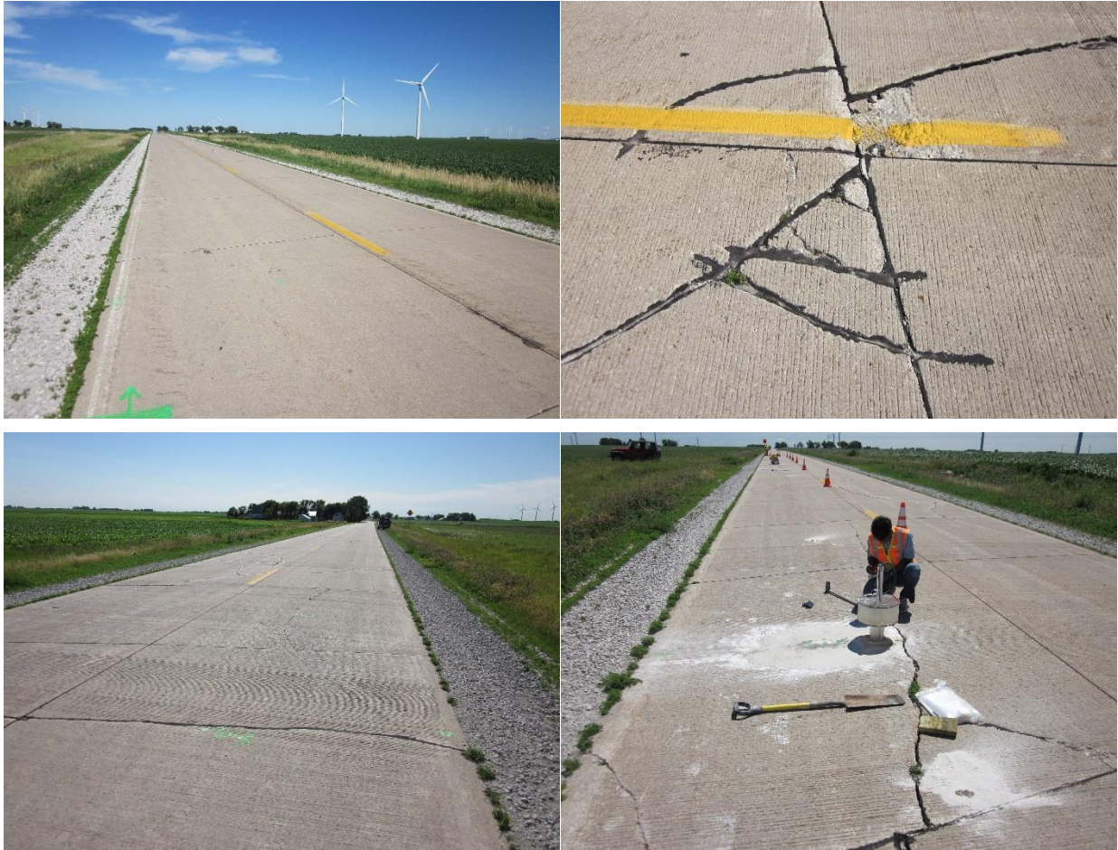
Figure 61. Photographs of field test site during testing — E23, Story County
