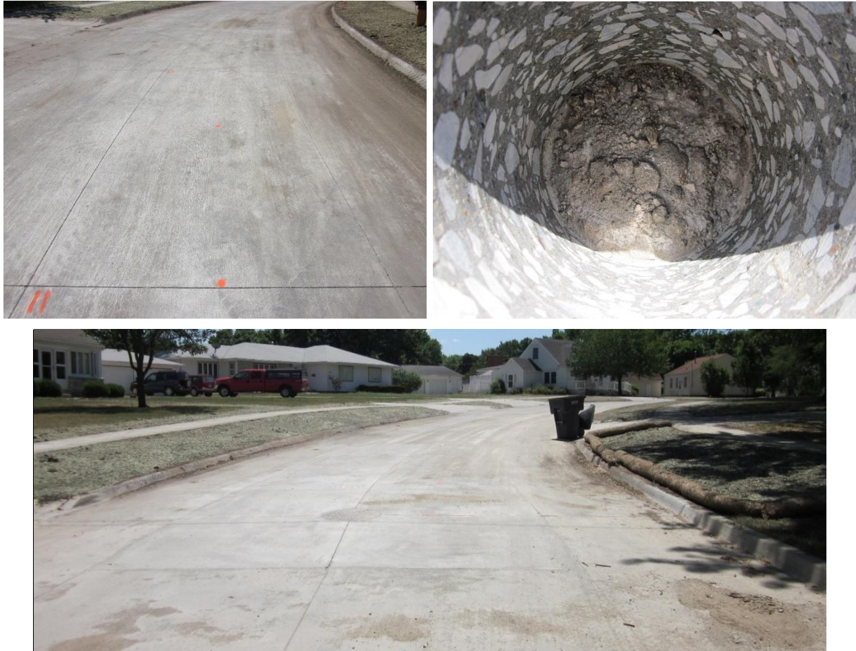
Figure 76. Photographs of field test site during testing — SW Logan Street, Ankeny
