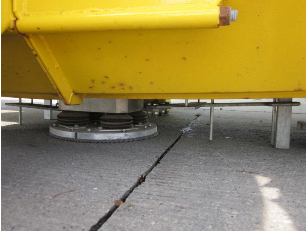
Figure 12. FWD test at a joint for LTE determination
