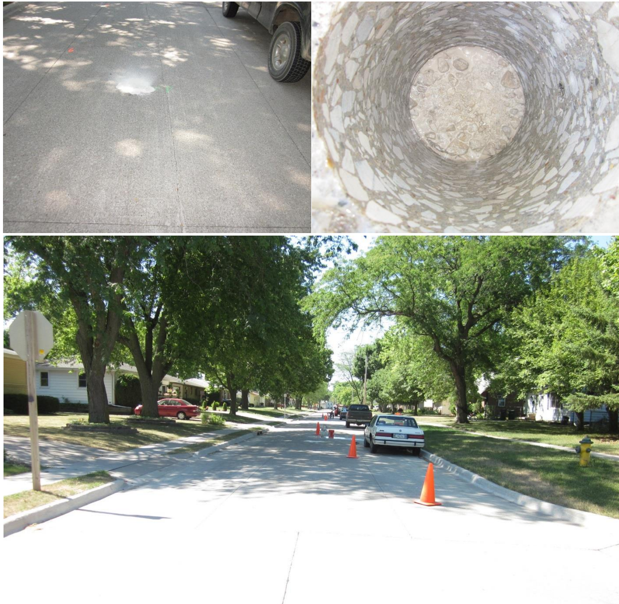
Figure 68. Photographs of field test site during testing — SW Westlawn Drive, Ankeny
