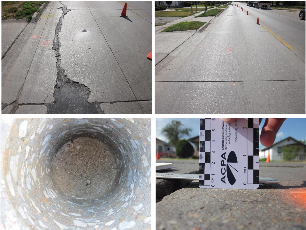
Figure 99. Photographs of field test site during testing — 9 th Avenue, Council Bluffs
