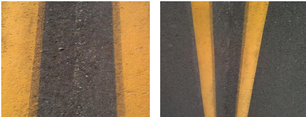
Figure 43. Longitudinal joint performance for the US 6 project
