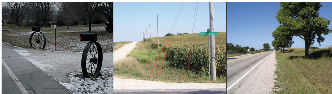
Removal of hazard(s) in clear zone (photos courtesy of Jack Latterell)
