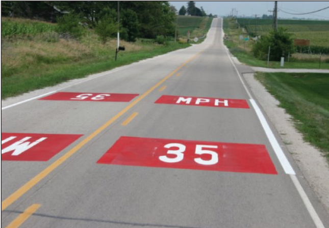
East entrance after treatments were installed (left) and west entrance treatment illustrating fading of pavement markings at nine-month data collection period (right) (photos courtesy of Shauna Hallmark)
