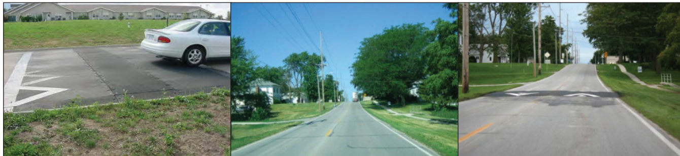
30 mph speed table used in the CTRE study for residential traffic calming (photos courtesy of Shauna Hallmark)
