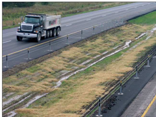
I-35 from bridge overpass (photo courtesy of Ryan Pettit)
