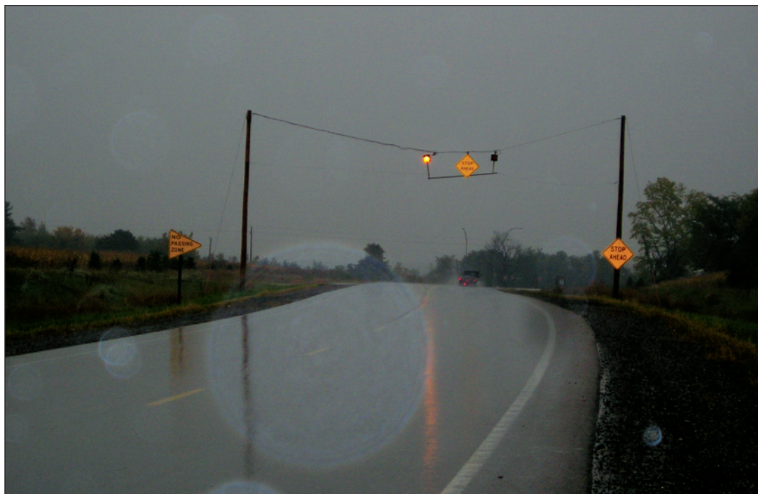
Warning beacon and sign(s) are an effective combination (photo courtesy of Tom McDonald) (Formerly county road—now Iowa 415)
