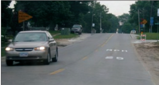
Speed limit pavement markings in Roland, IA (photo courtesy of Shauna Hallmark)
