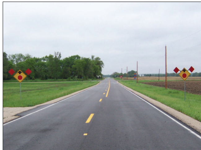
View of flags on warning signs
