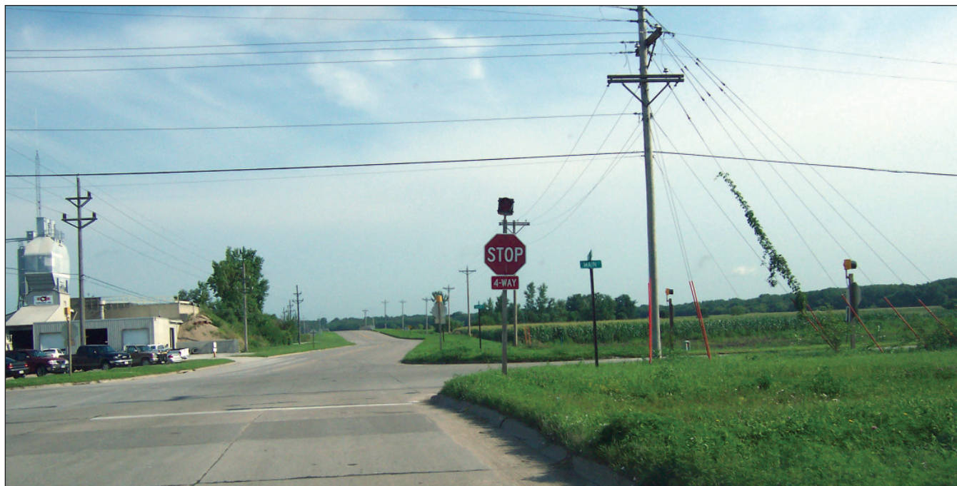
36 in. Stop sign at paved/paved intersection (photo courtesy of Grundy County)
