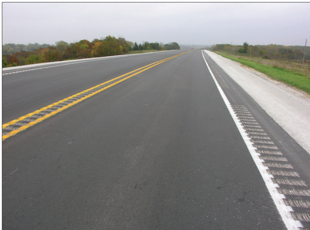
Centerline and shoulder rumble strips (photo courtesy of Jack Latterell)
