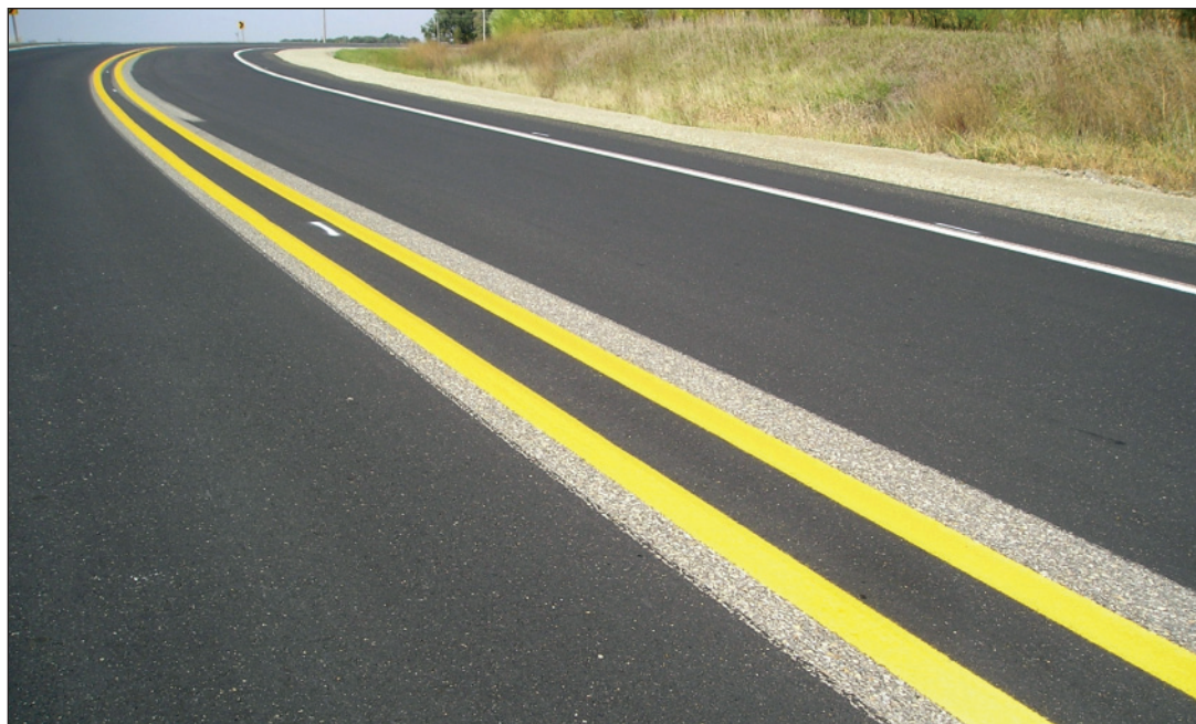
Milled in centerline pavement markings (photo courtesy of Tom McDonald)
