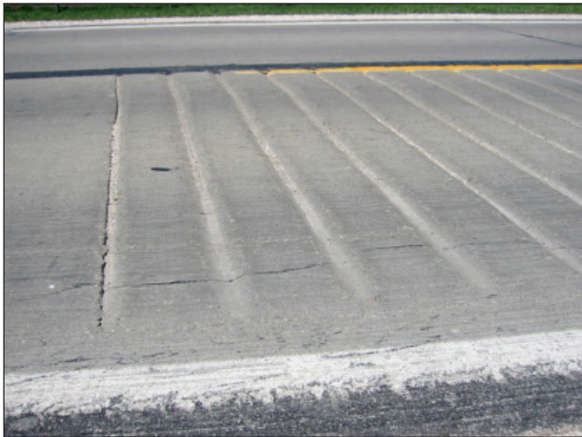
Advance rumble strips on PCC approach (photo courtesy of Bob Sperry)
