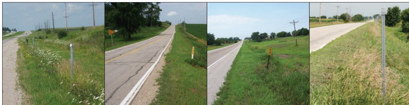
Single reflective and triple amber delineators and markers (photos courtesy of Bob Sperry)
