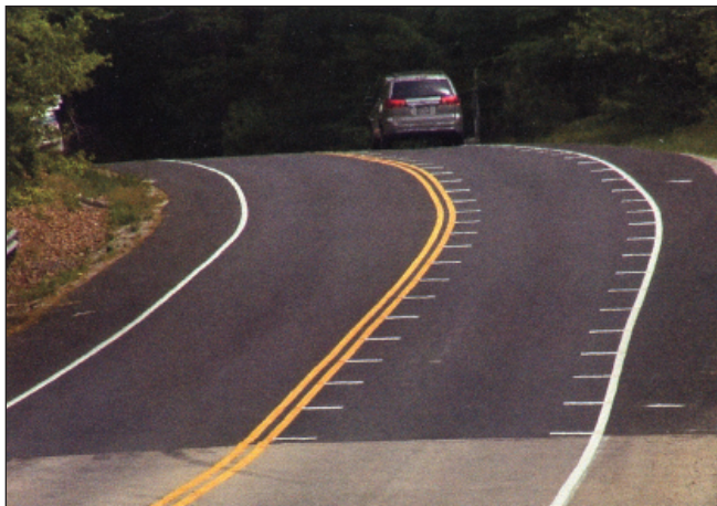
Optical speed bars used to reduce vehicle speed (photo courtesy of Virginia Department of Transportation)
