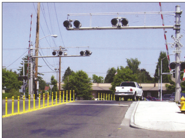
Longitudinal channelizers at railroad crossings reduce gate violations (left photo courtesy of Peter Speer)
