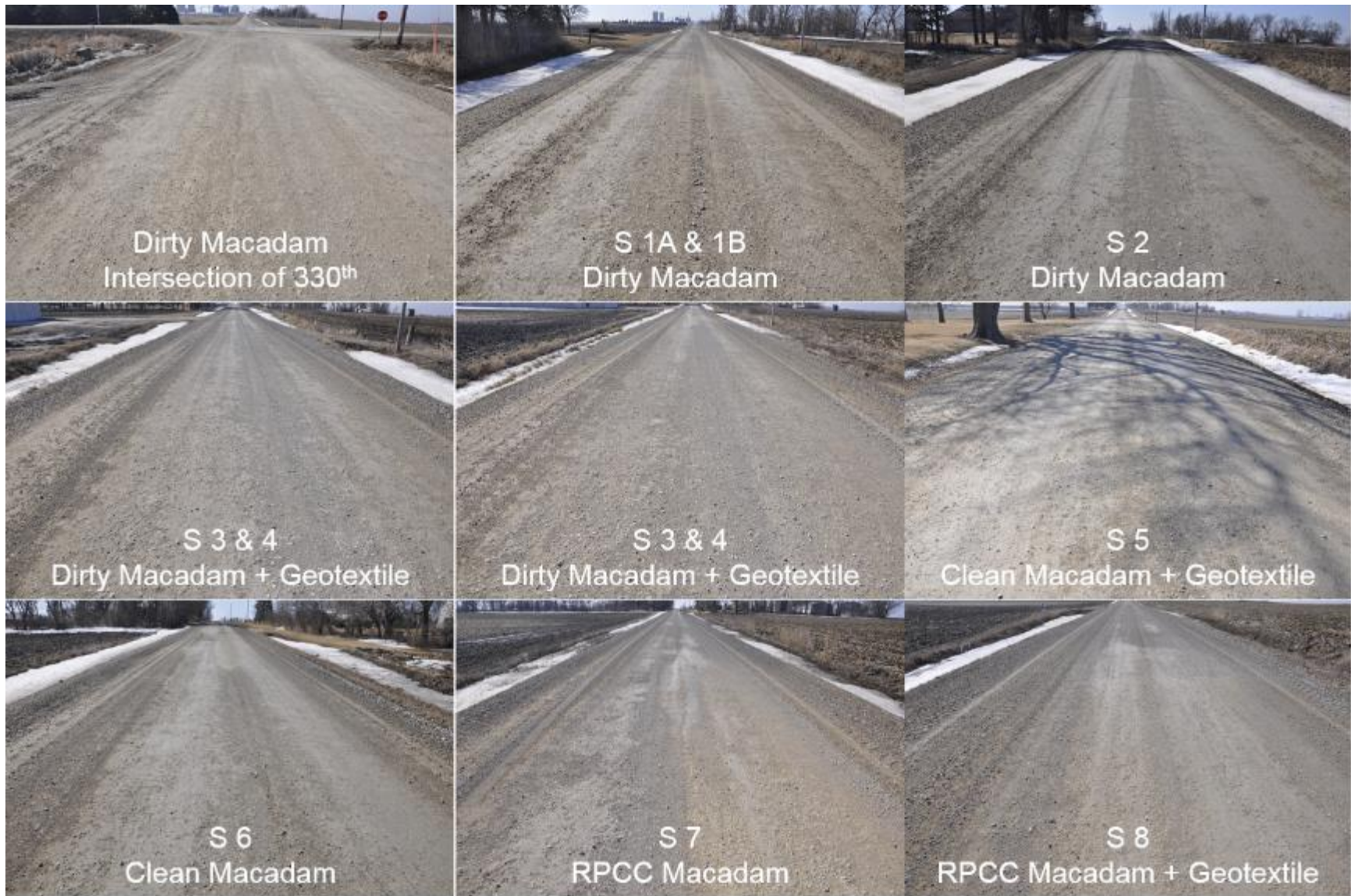
Figure 124. Survey photos of Vail Avenue demonstration sections (March 20, 2014)
