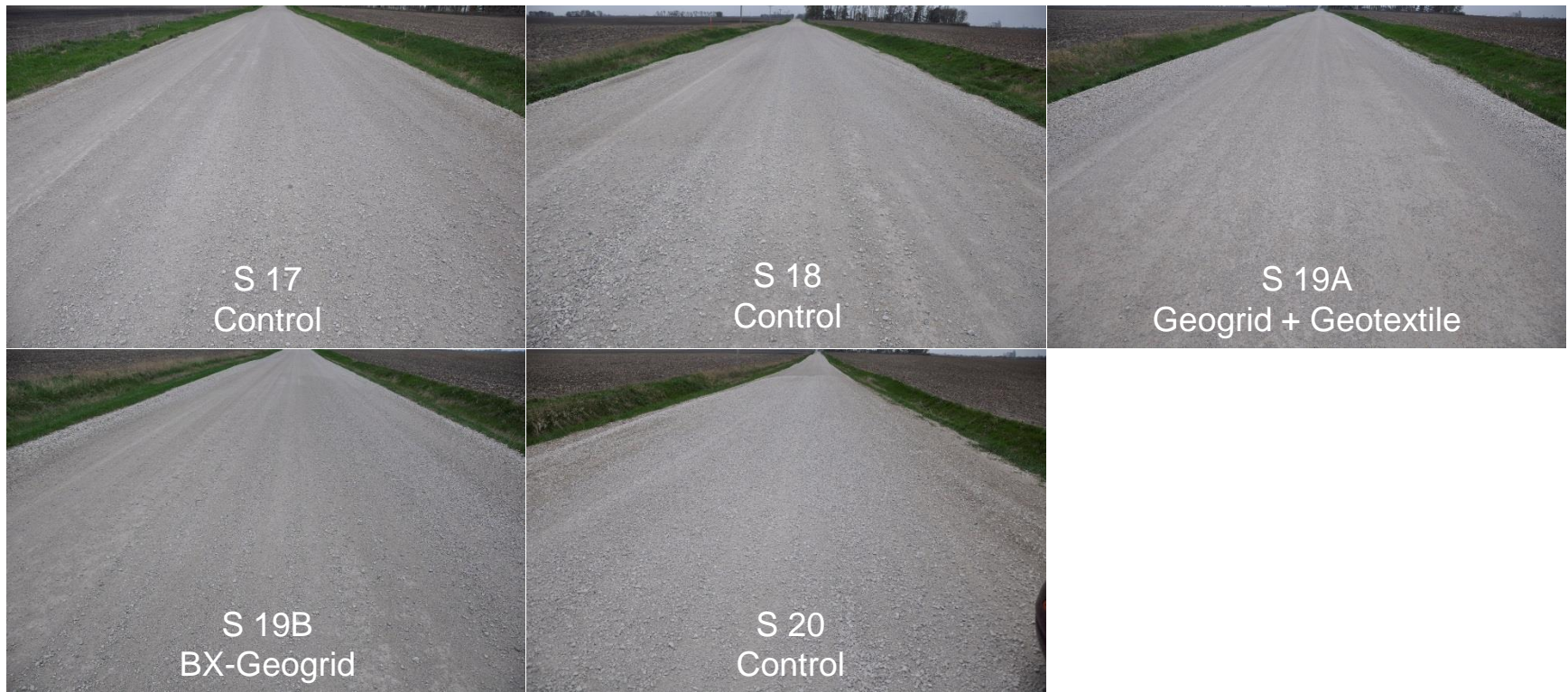
Figure 126. (continued). Survey photos of Vail Avenue demonstration sections (May 8, 2014)
