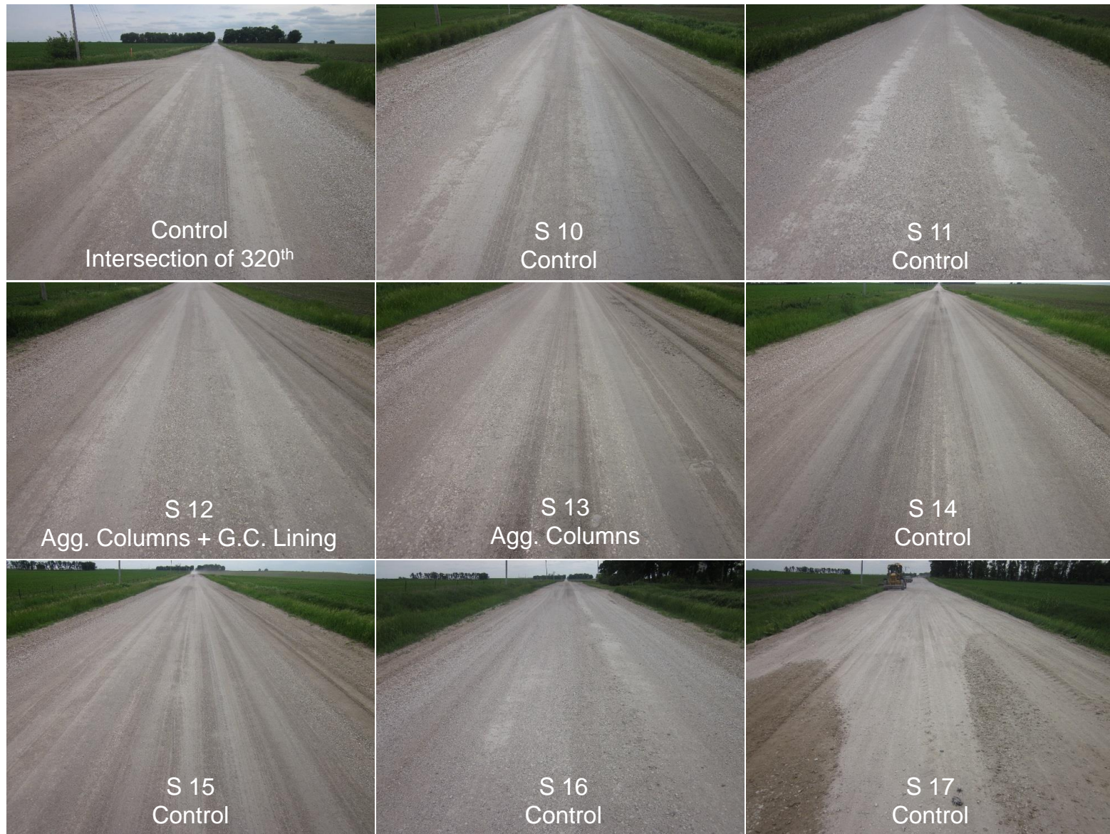
Figure 127. (continued). Survey photos of Vail Avenue demonstration sections (June 6, 2014)
