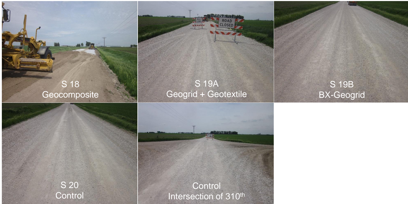
Figure 127. (continued). Survey photos of Vail Avenue demonstration sections (June 6, 2014)
