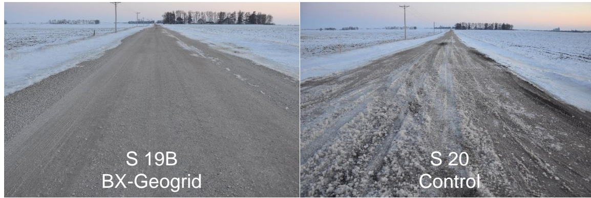
Figure 123. (continued). Survey photos of Vail Avenue demonstration sections (March 8, 2014)
