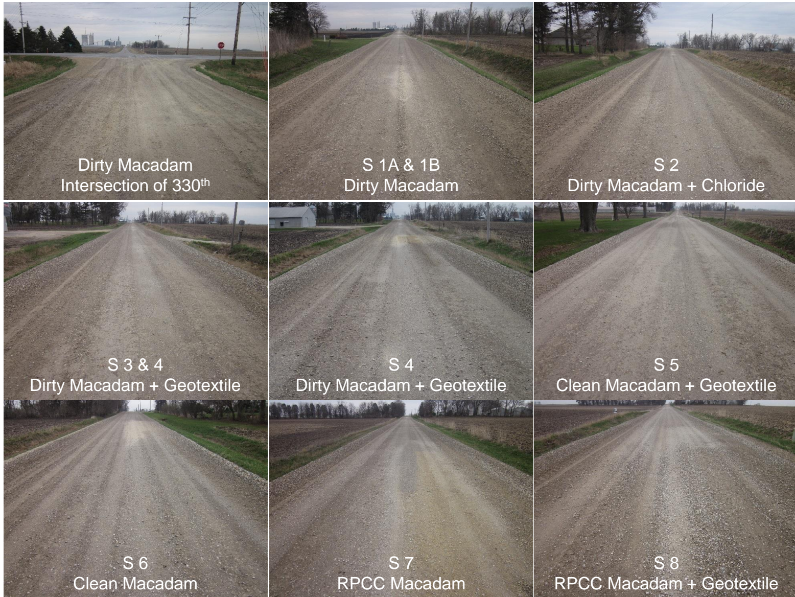
Figure 125. Survey photos of Vail Avenue demonstration sections (April 21, 2014)
