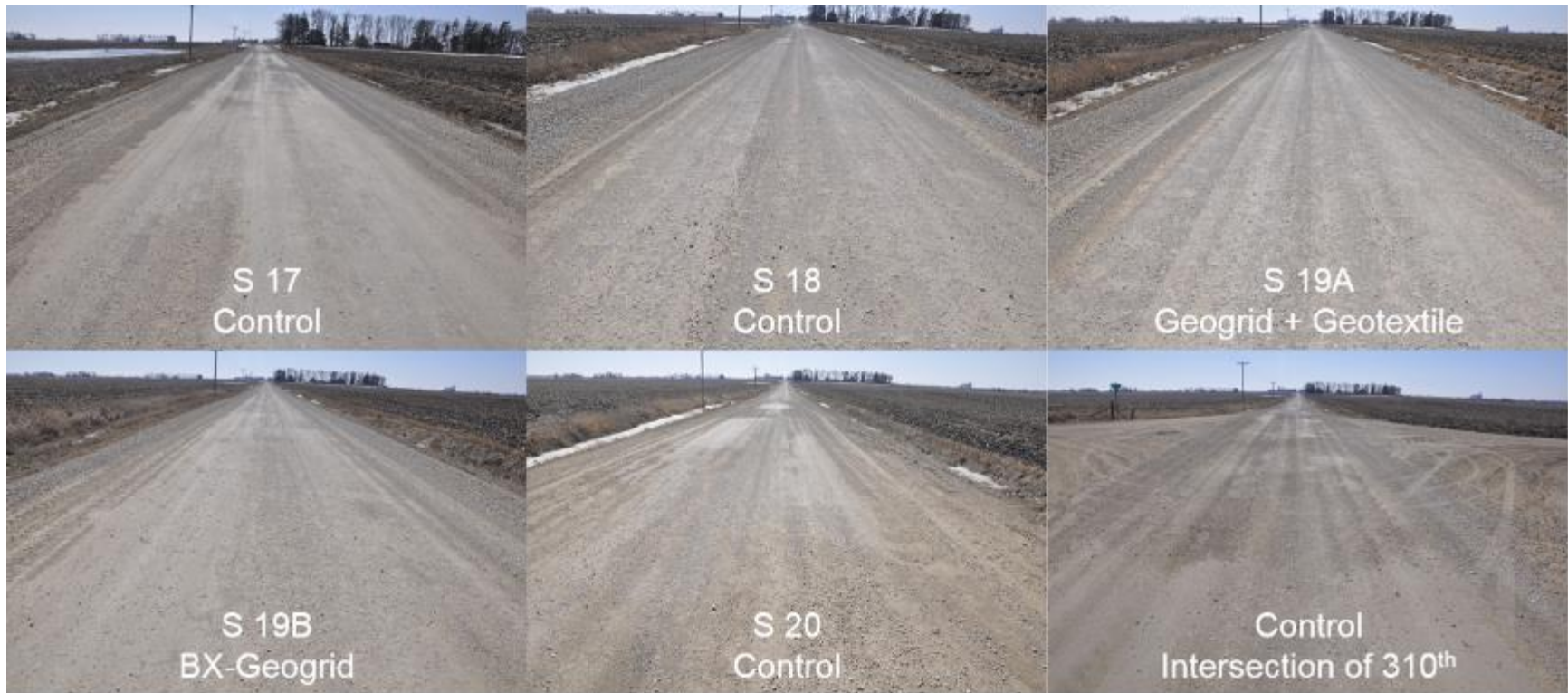
Figure 124. (continued). Survey photos of Vail Avenue demonstration sections (March 20, 2014)
