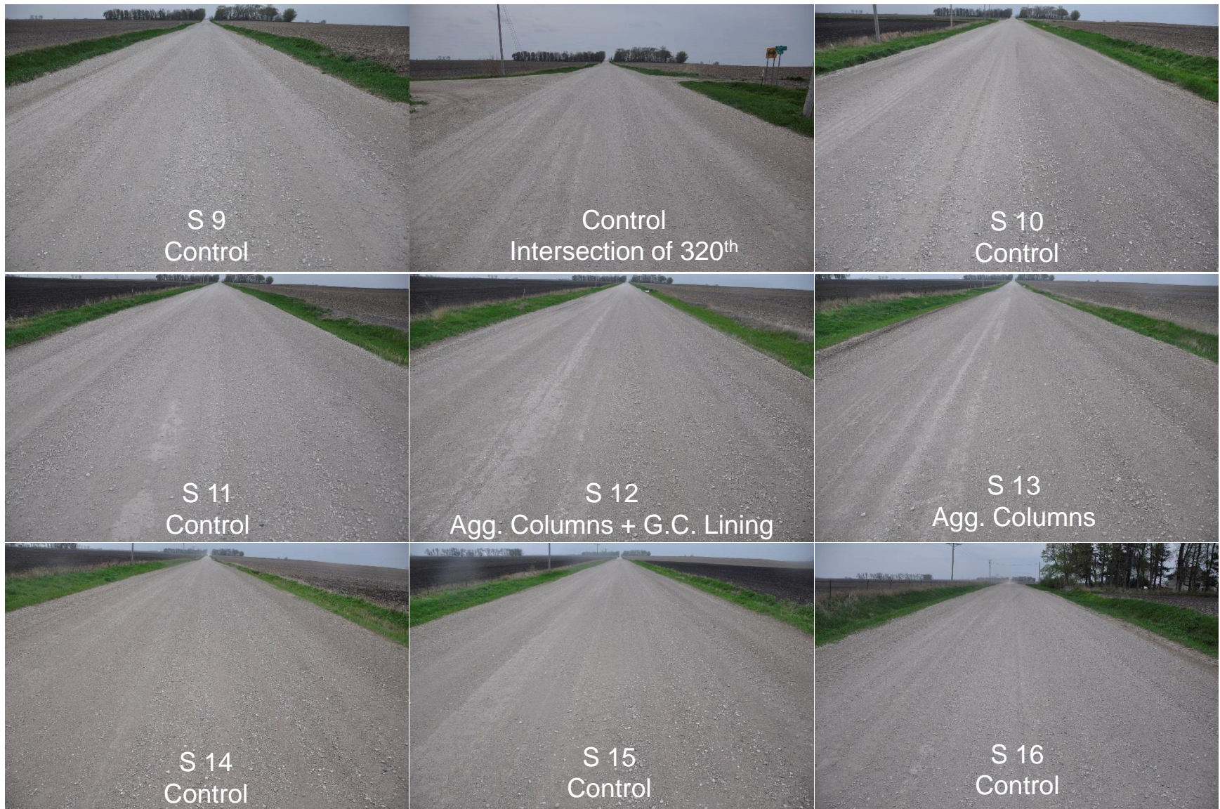
Figure 126. (continued). Survey photos of Vail Avenue demonstration sections (May 8, 2014)
