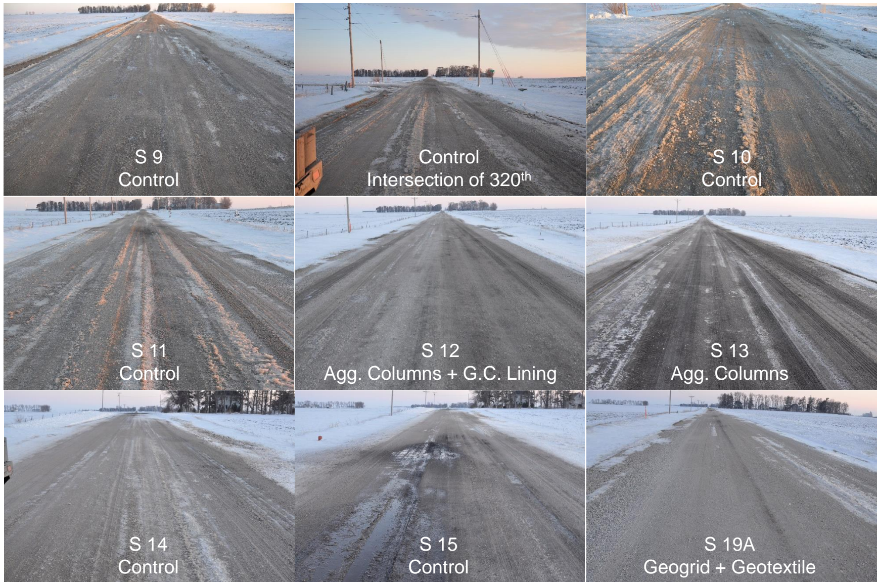
Figure 123. (continued). Survey photos of Vail Avenue demonstration sections (March 8, 2014)
