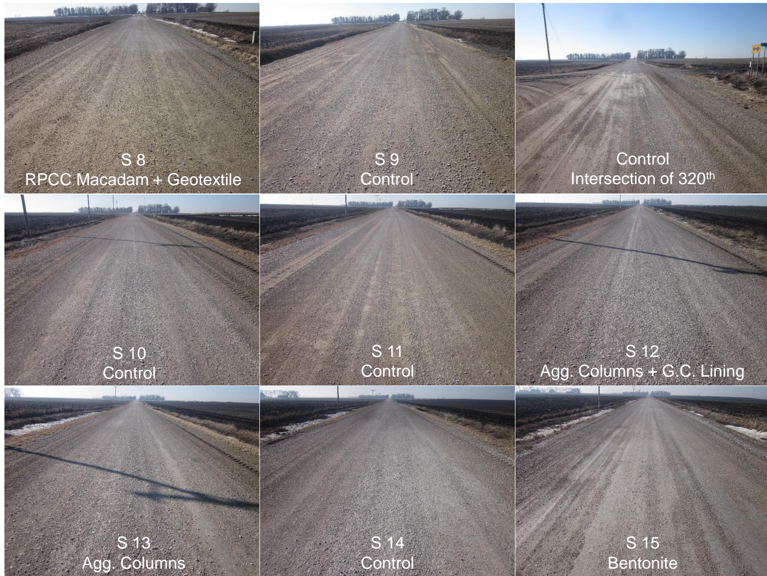
Figure 132. (continued). Survey photos of Vail Avenue demonstration sections (March 10, 2015)
