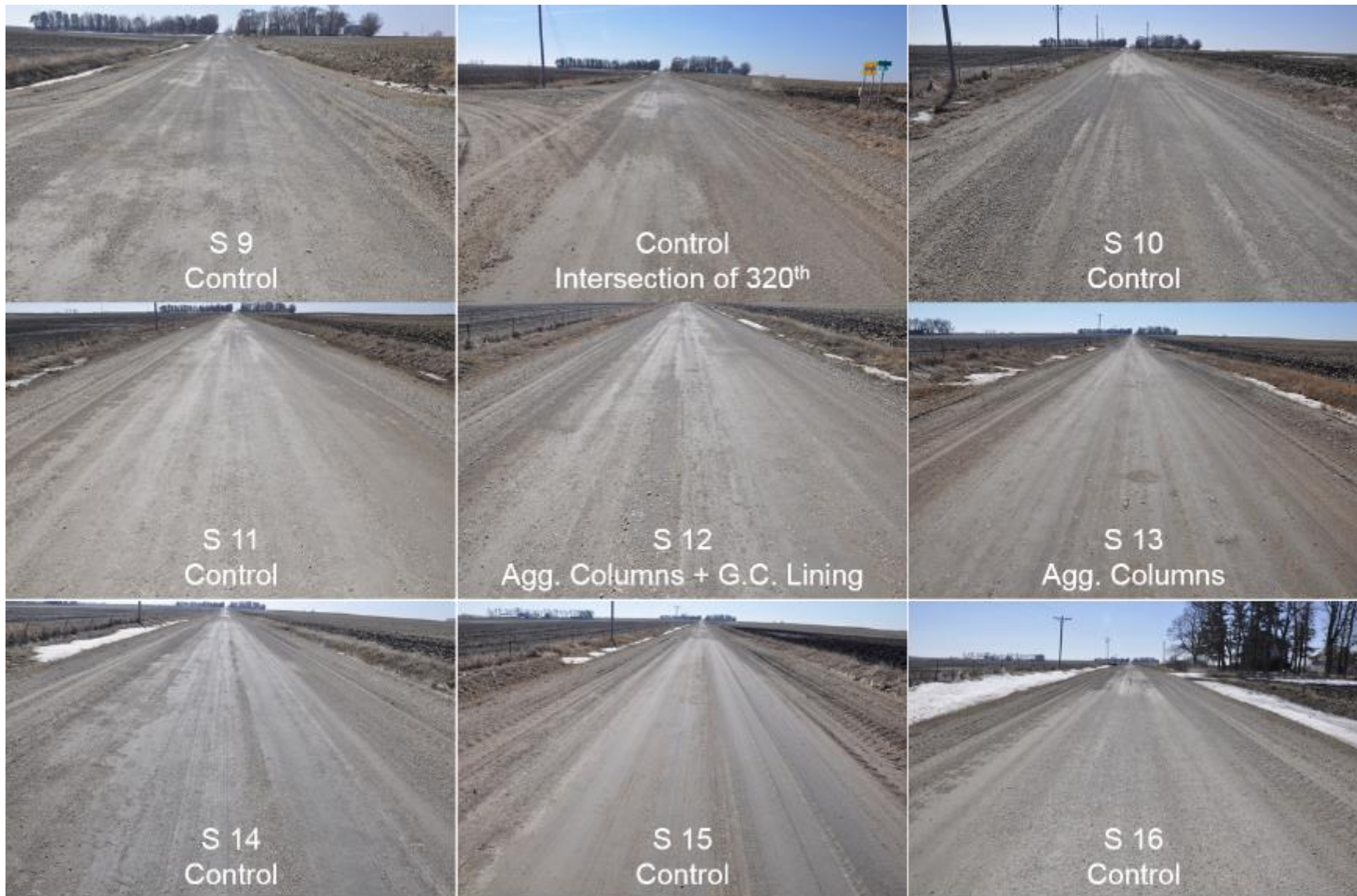
Figure 124. (continued). Survey photos of Vail Avenue demonstration sections (March 20, 2014)
