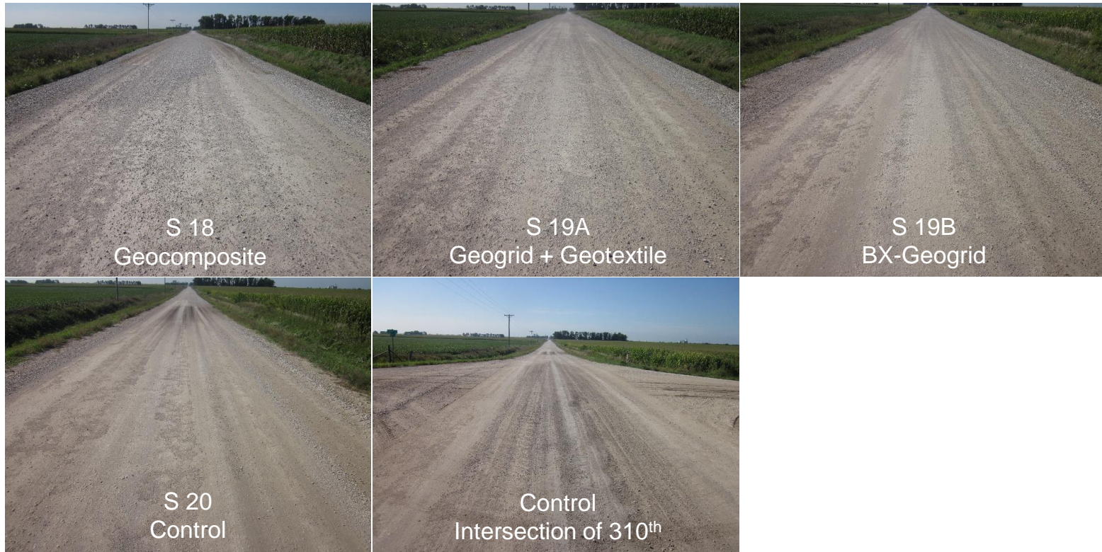
Figure 129. (continued). Survey photos of Vail Avenue demonstration sections (September 2, 2014)
