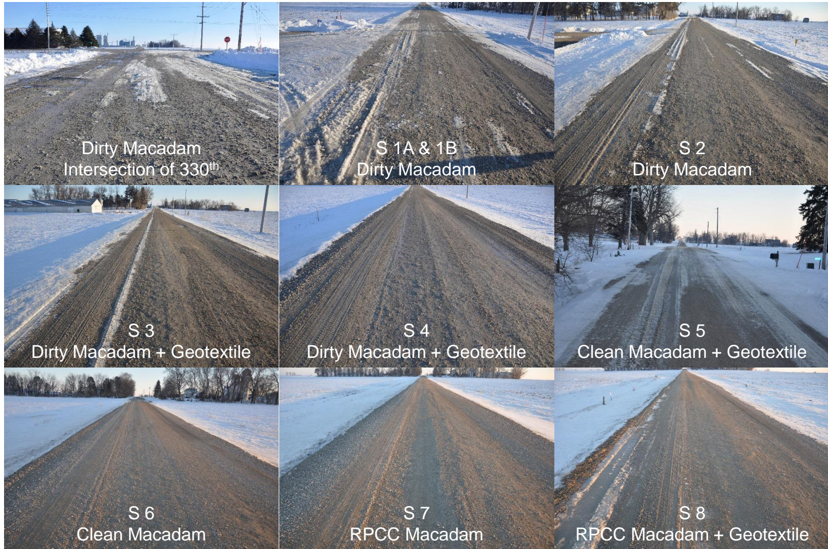
Figure 123. Survey photos of Vail Avenue demonstration sections (March 8, 2014)
