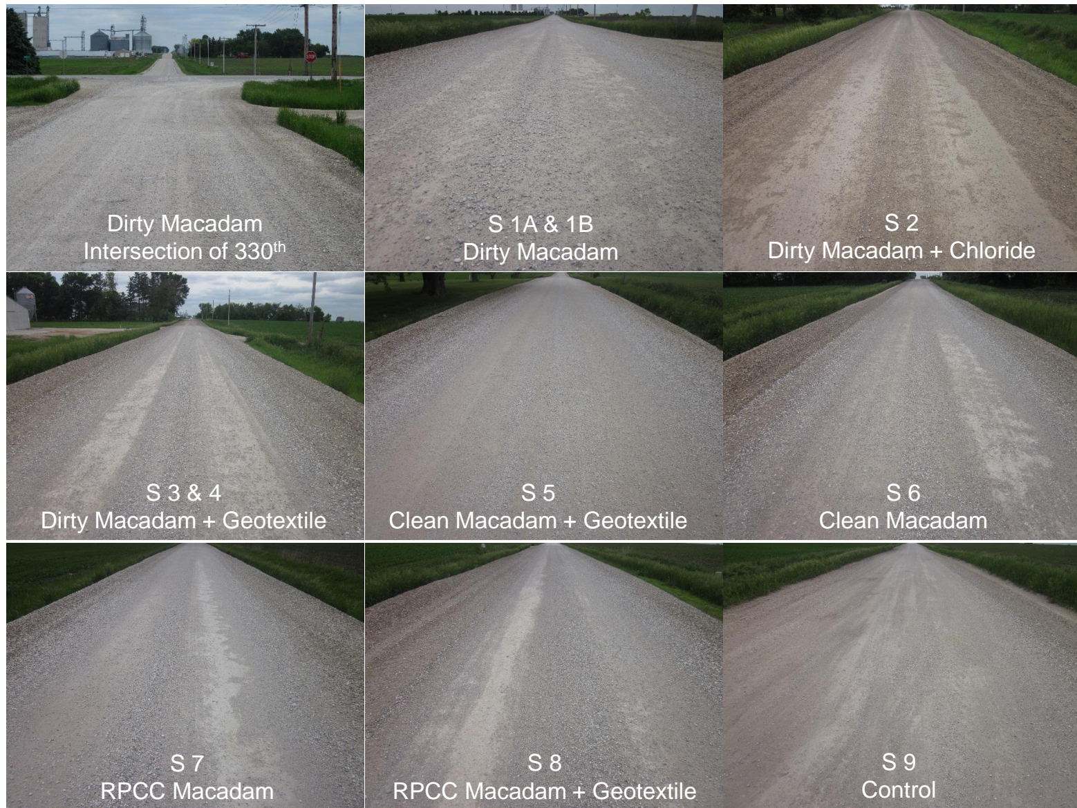
Figure 127. Survey photos of Vail Avenue demonstration sections (June 6, 2014)
