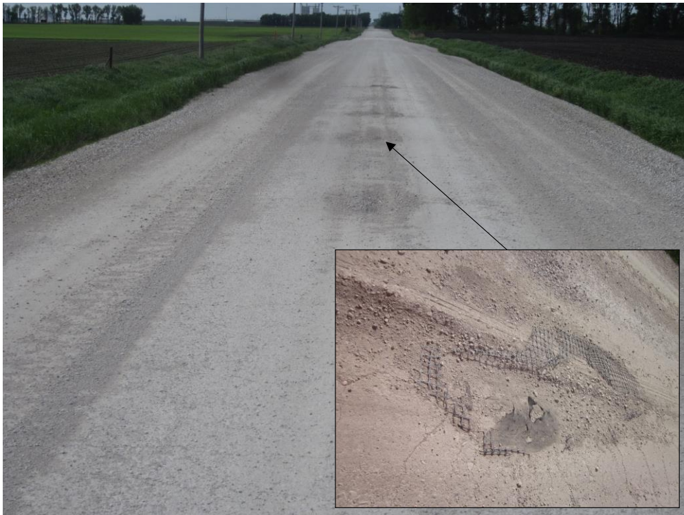
Figure 103. Surface condition of BX-geogrid+NW-geotextile Section 19A showing exposed geosynthetics (May 20, 2015)
