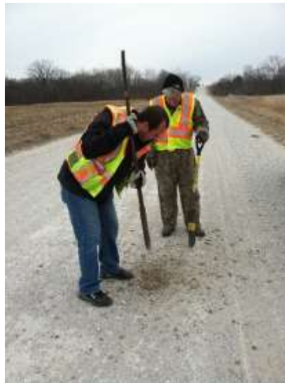
Figure 3. Installation of buried Numetric plate
