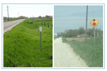
Sample Mitigation: New, highly-reflective delineators and signs installed in Dallas and Story counties
