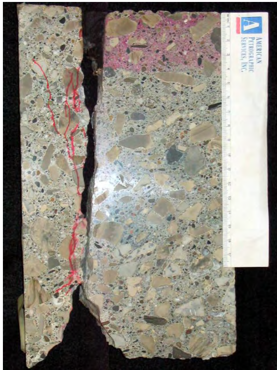
Figure 12. High water-cement ratio and cracking left half of the cold joint
