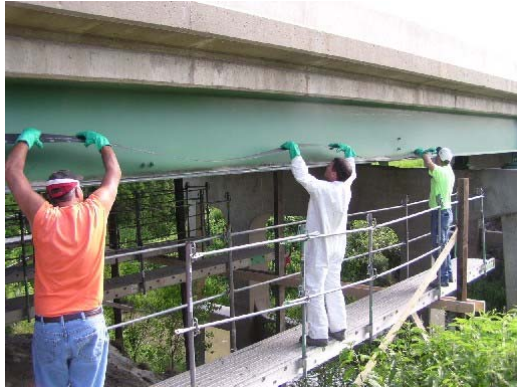
(e) Placement of CFRP plate
