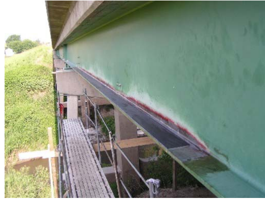
(f) CFRP plate installed.
