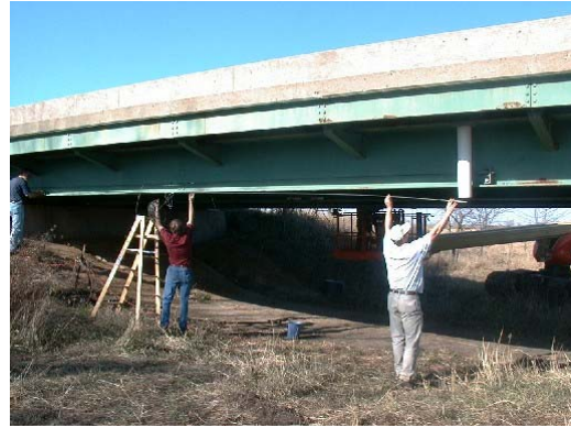
(b) Placement of CFRP rod
