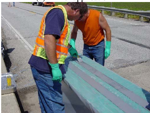
(c) Epoxy application on CFRP plates
