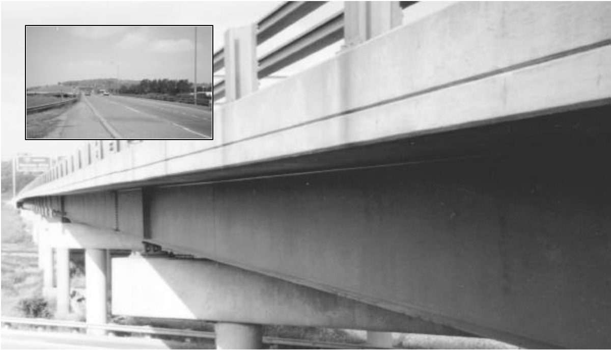
(a) Overview and roadway
