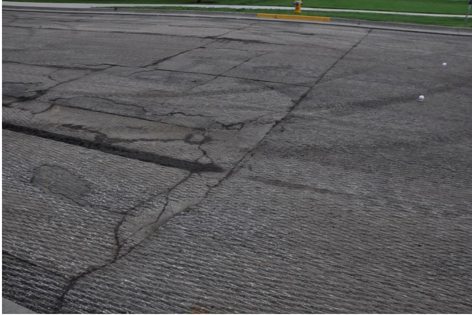
Figure 20. Wilson parking lot before paving
