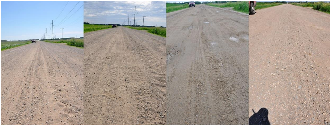
Figure 15. East section of 210th Street at different times: June 5 (left), June 6 (middle-left), June 8 (middle-right), and June 9 (right); blading occurred June 4 and June 15
