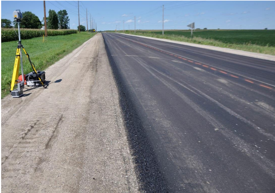
Figure 24. Intermediate asphalt layer of the north section of Highway 69
