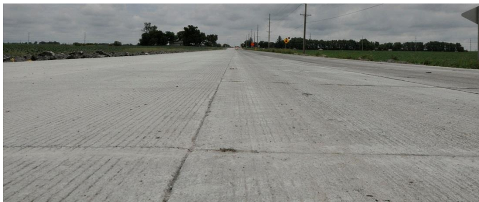
Figure 23. Concrete surface of the south section of Highway 69 after paving
