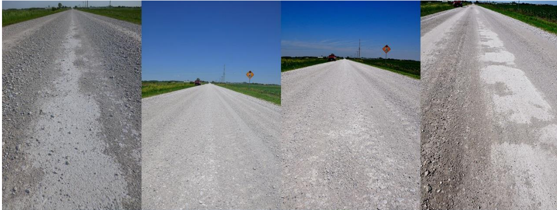
Figure 18. 520th Avenue in Story County at different times: June 1, June 9, June 10, and June 16. Blading occurred June 9 and June 29
