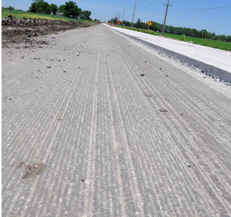
Figure 22. Milled concrete surface of the south section of Highway 69 before paving
