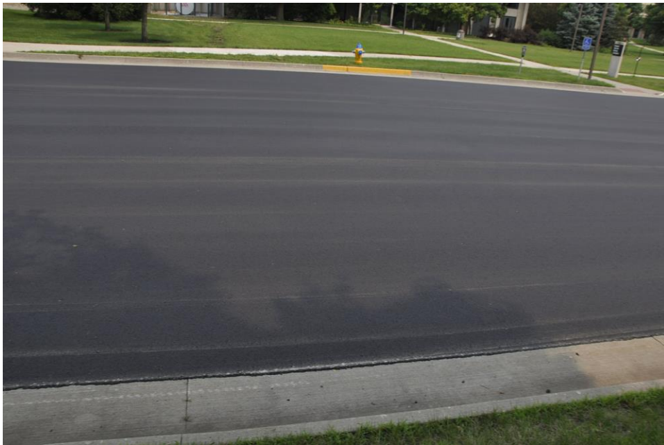
Figure 21. Wilson parking lot after paving
