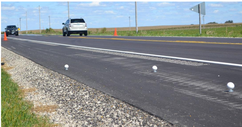
Figure 25. Finished asphalt layer of the north section of Highway 69
