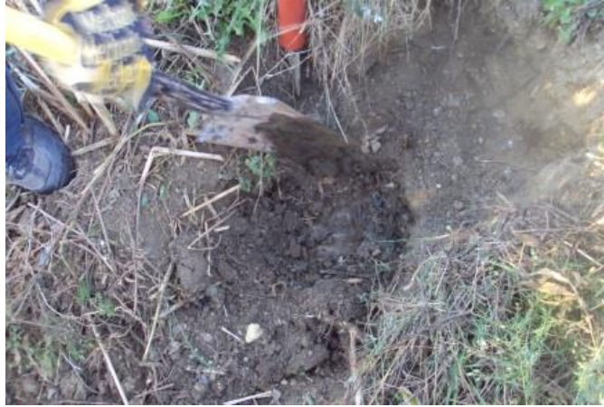
Figure 15. Clearing debris surrounding subsurface drainage outlet in I-35/N/MP140.35
