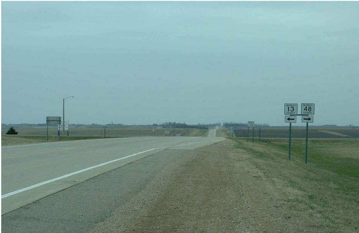
Murray County: US59 and CSAH 13/CSAH 48 (looking south)
