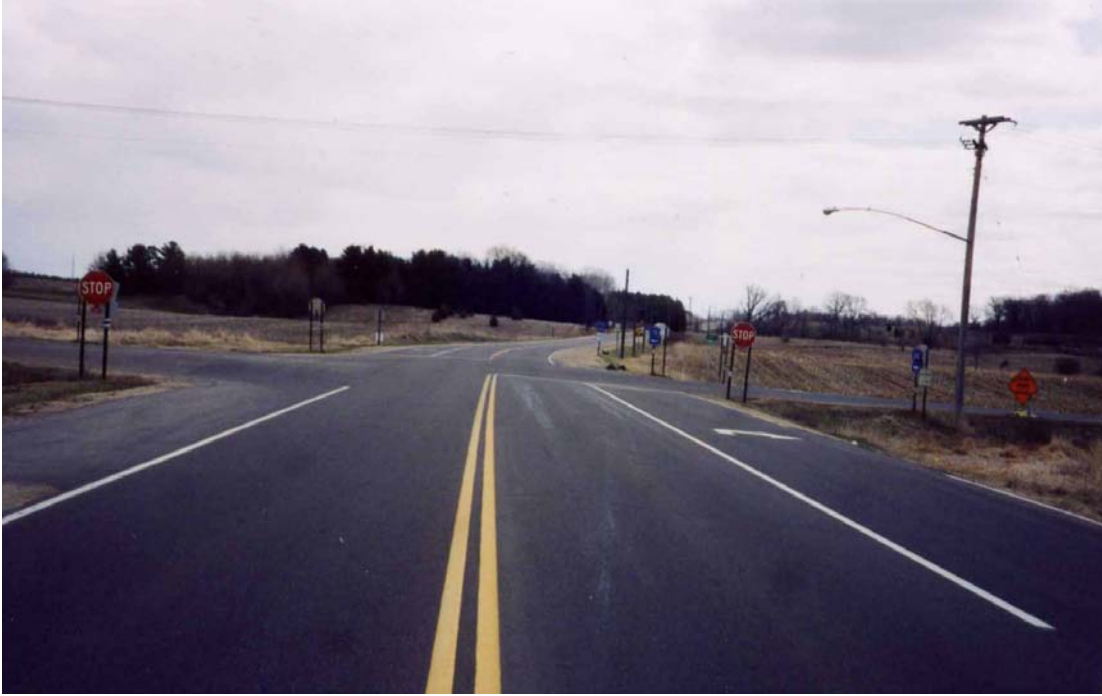
Washington County: CSAH 20 and CSAH 13 N (looking east)
