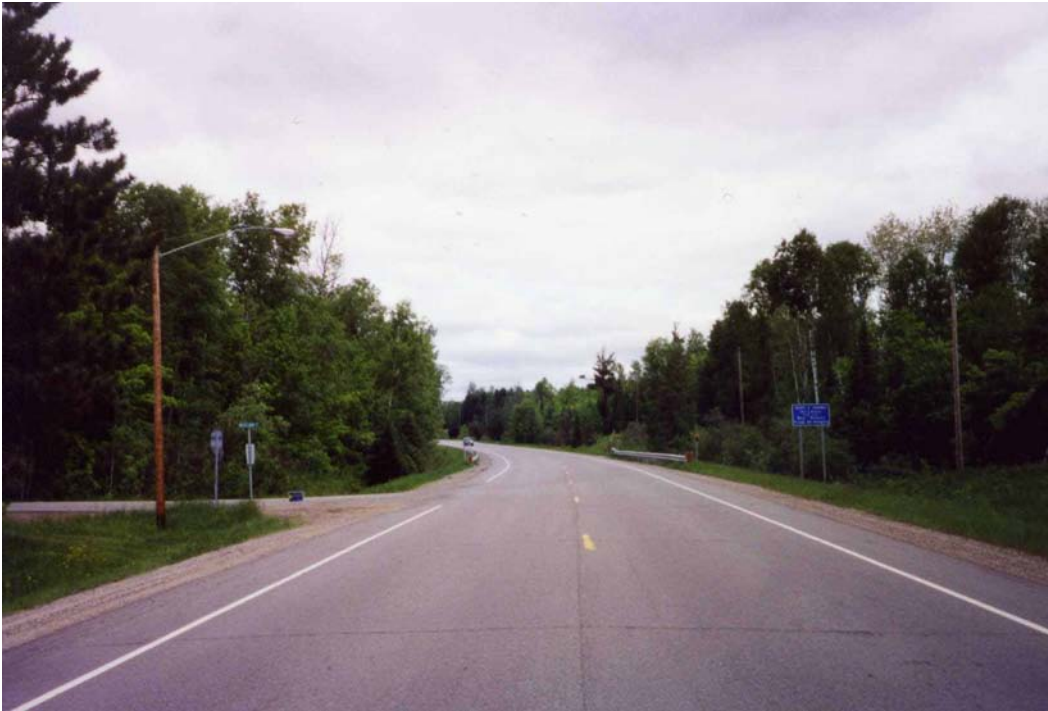
Itasca County: TH 65 and West Bay Drive (looking north)
