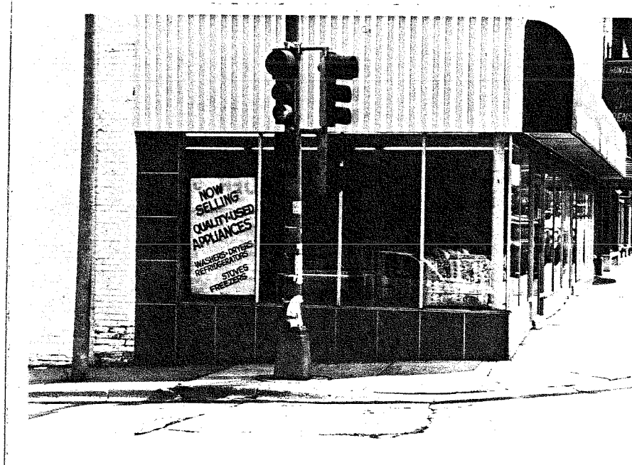
a. Before installation of countermeasure.
