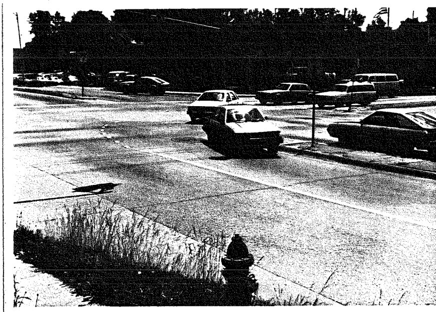
b. After installation of countermeasure.
