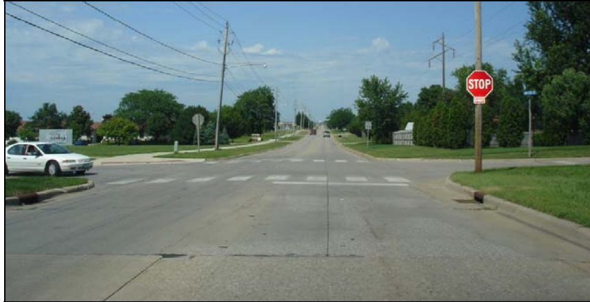
Figure 2-12. Existing four-way stop intersection looking north
