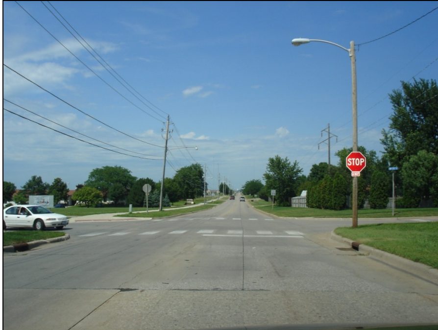
Figure 9-48. Existing four-way stop intersection looking north
