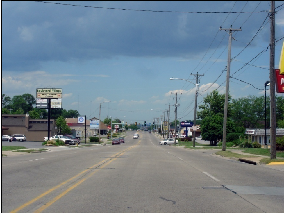
South section of US 69 with no access control
