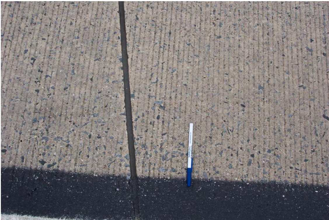
Figure 17. Delaware SR 896 southbound (between US 40 and Highway 71)
