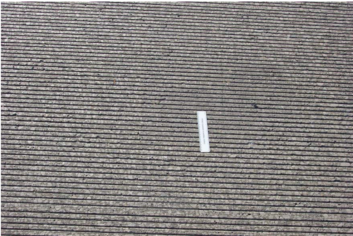
Figure 9. Euclid bridge, westbound driving lane
