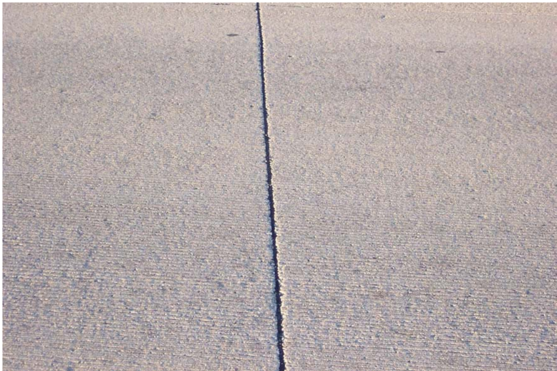
Figure 3. Highway 520 eastbound at mile post 157.85
