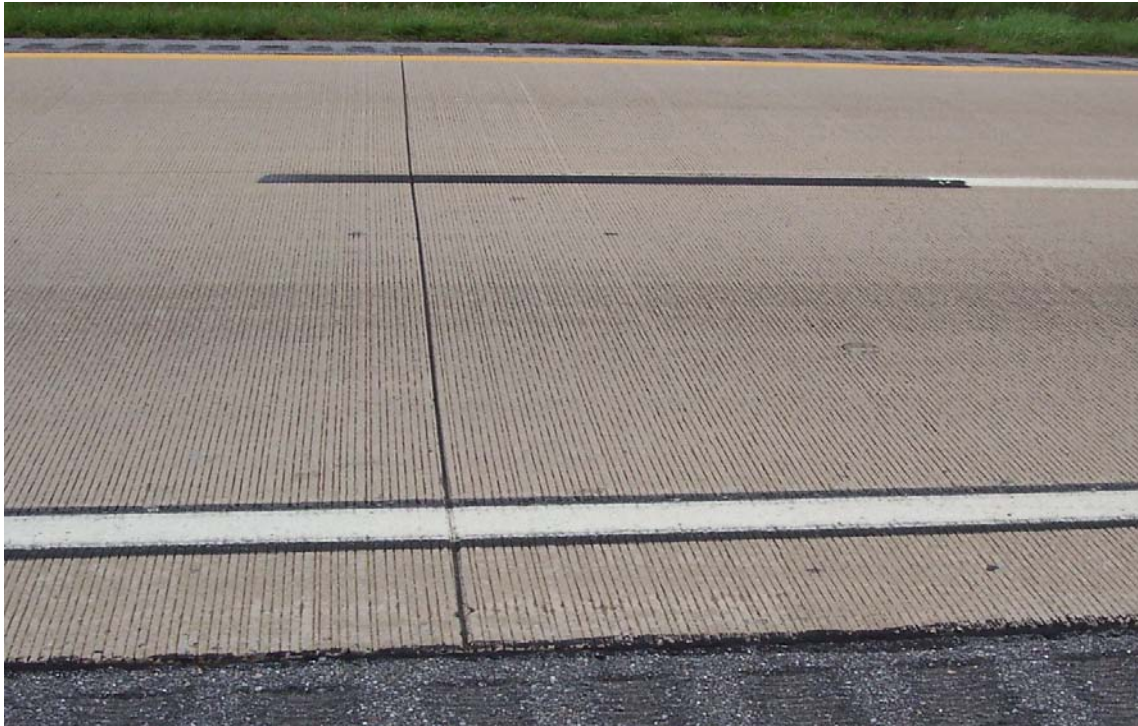
Figure 18. Delaware SR1, southbound (between Smyrna and Dover, north of MP 73)
