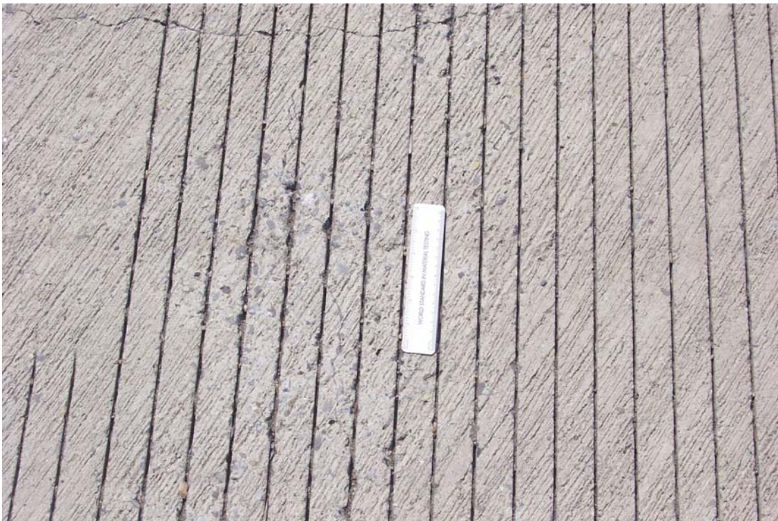
Figure 33. Close-up of exposed aggregate on the Route 378 deck
