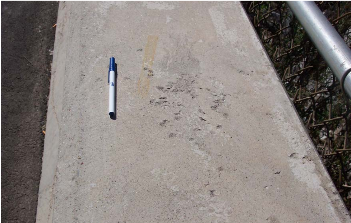
Figure 10. Barrier wall adjacent to exit 29A, Hartford, Connecticut
