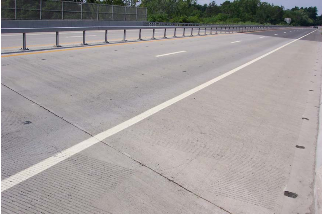
Figure 32. Overview of the Route 378 bridge over the D&H Railroad
