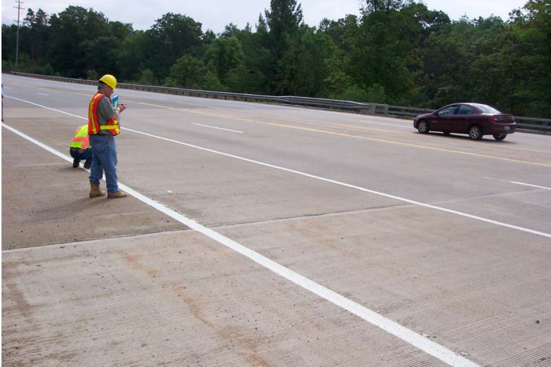
Figure 25. Overview of the short bridge on M-45 over Sand Creek
