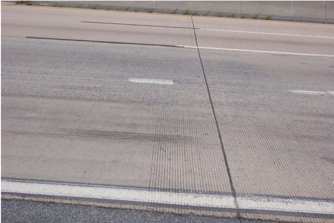
Figure 14. I-495 (between 9th Street and 12th Street, Wilmington, Delaware)
