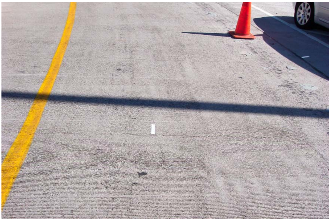
Figure 12. Bridge deck #1863, ramp to Whitehead Highway, SR 598
