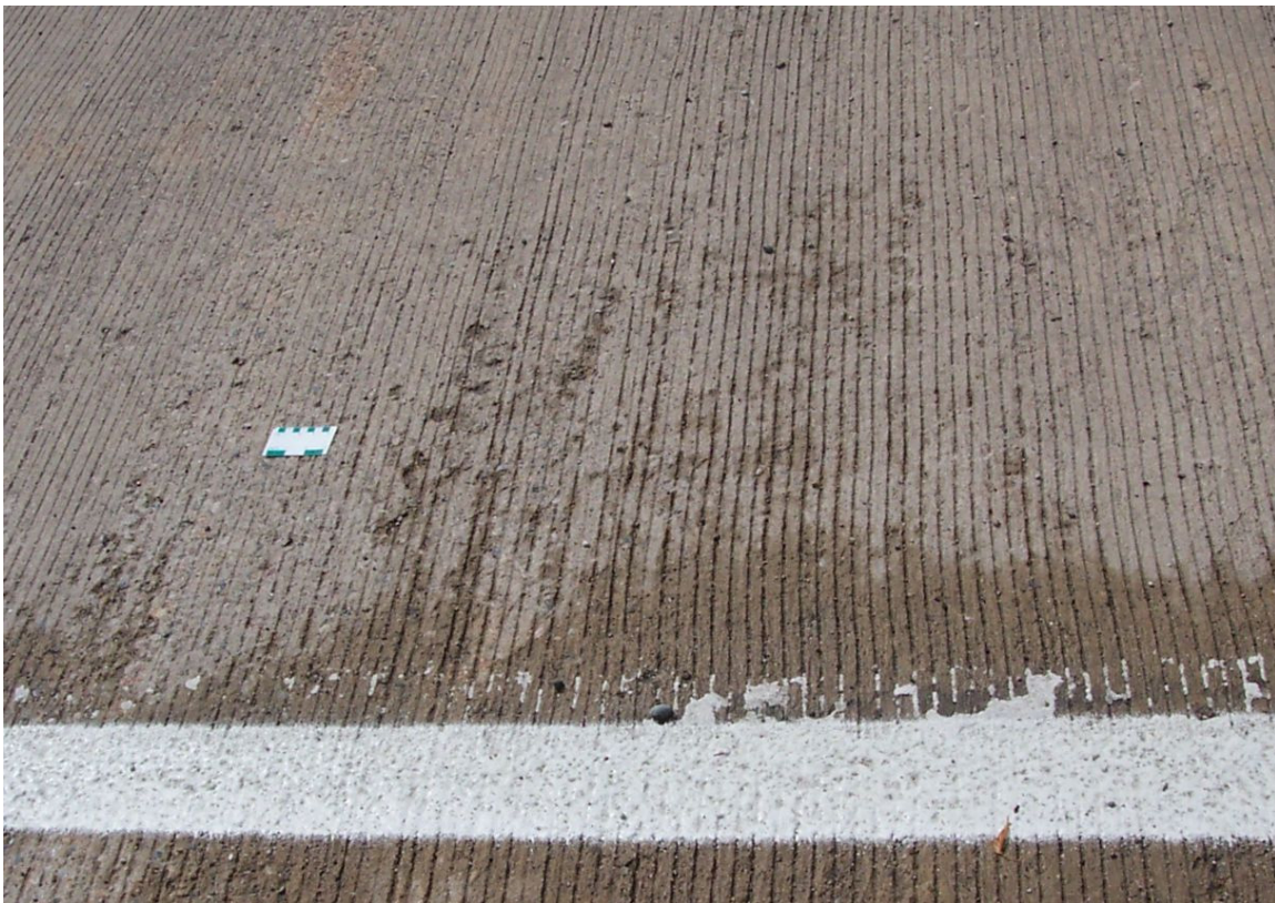
Figure 26. Close-up view of Figure 25 showing the varied tine depth across the deck
