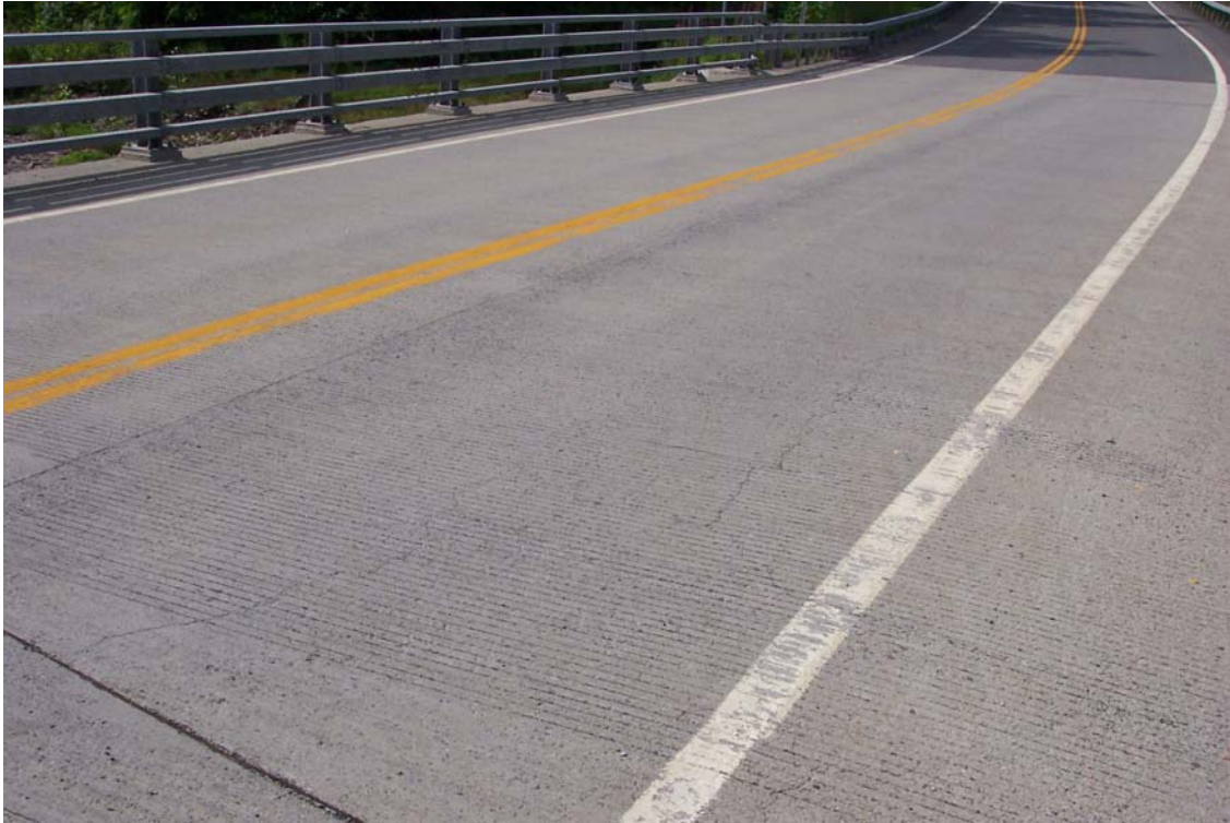
Figure 29. Overview of the Route 397 bridge over the Bozenkill
