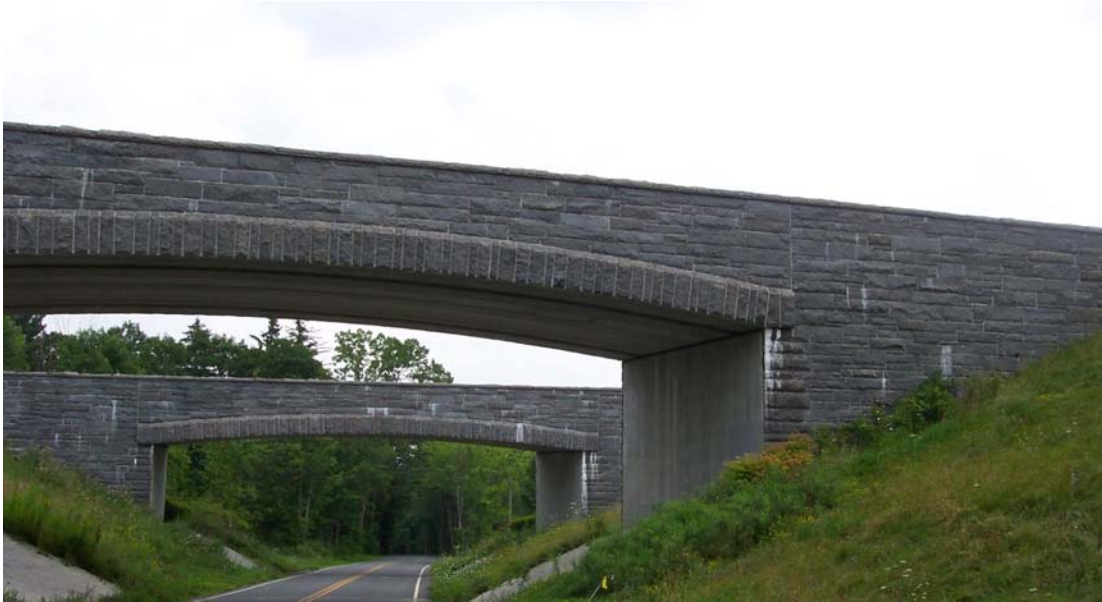
Figure 36. Overview of the Taconic St. Parkway bridges over Angel Hill Road
