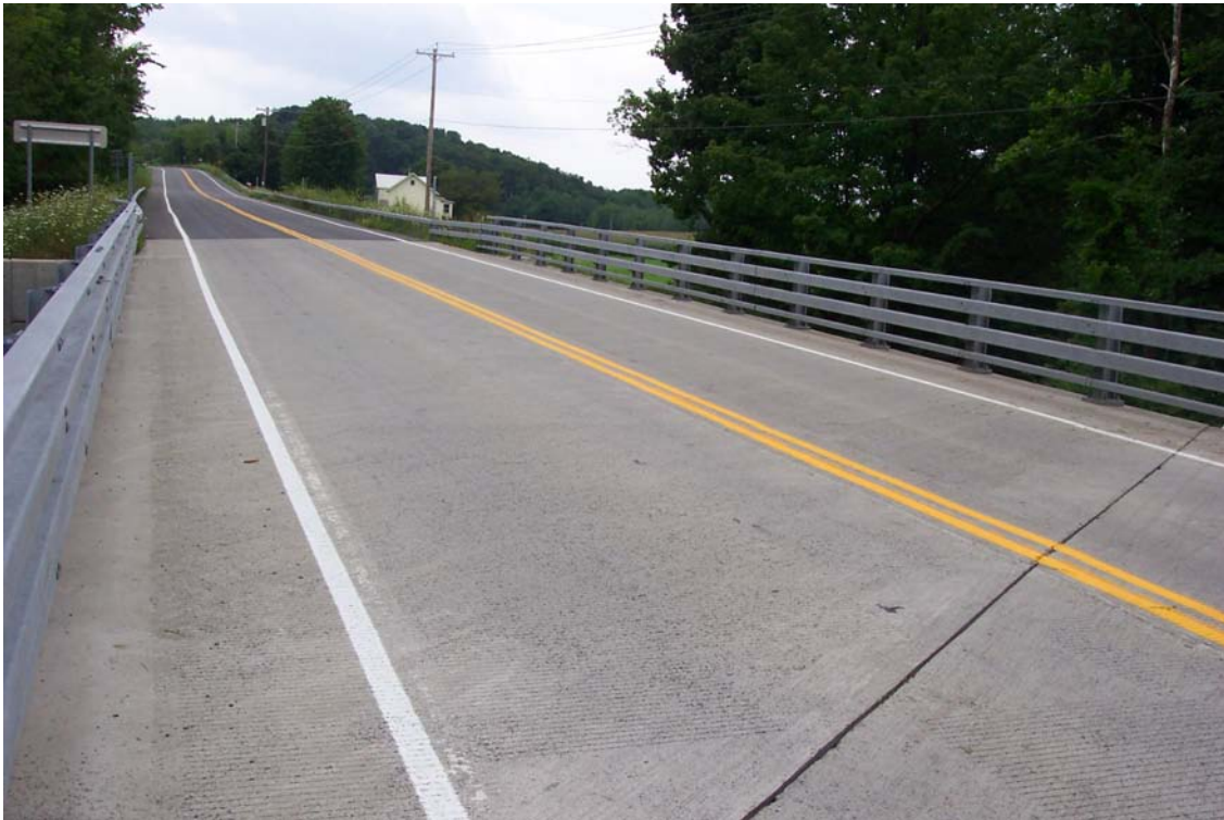
Figure 34. Overview of Route 351 bridge over the Quackenkill
