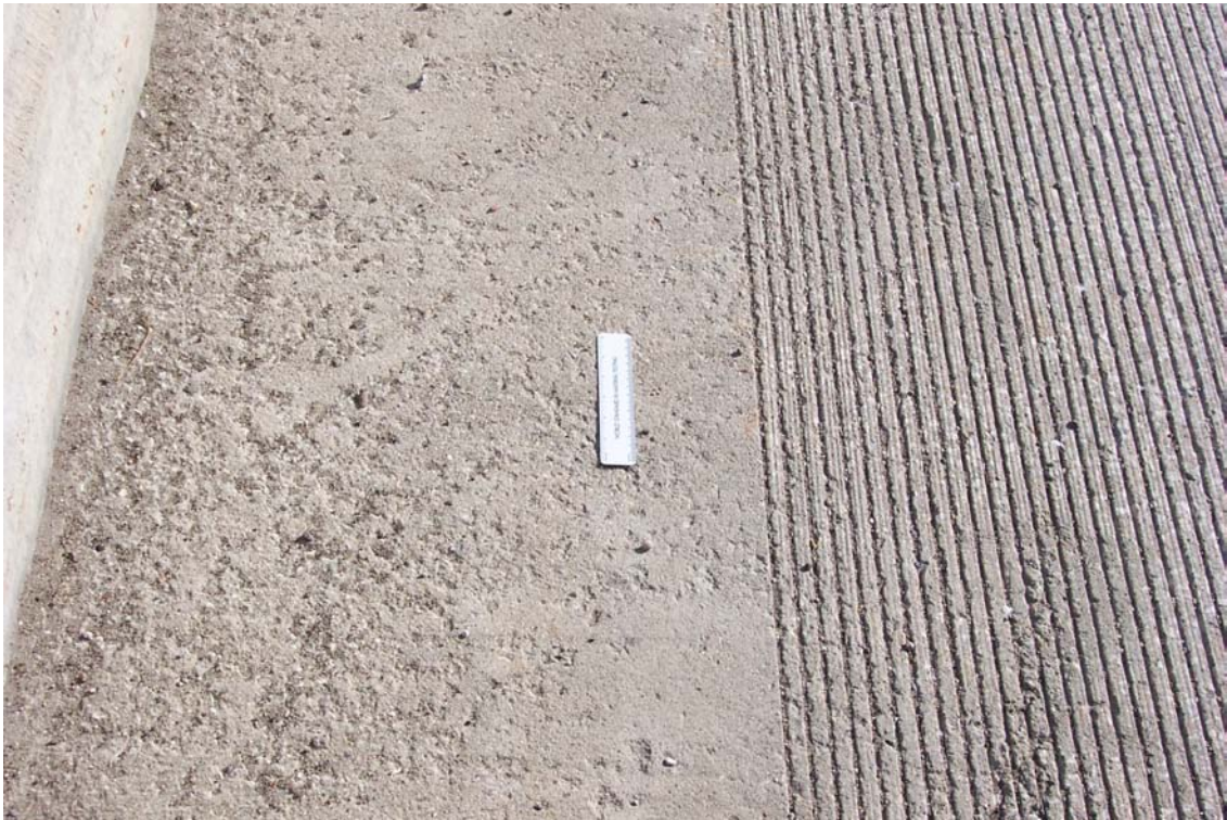
Figure 7. Euclid bridge, westbound
