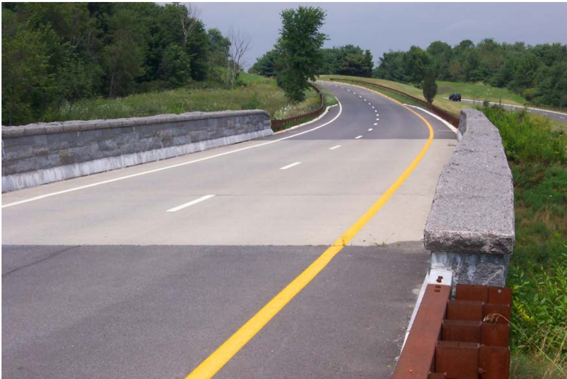
Figure 37. Overview of Taconic St. Parkway bridge, southbound deck (looking north)
