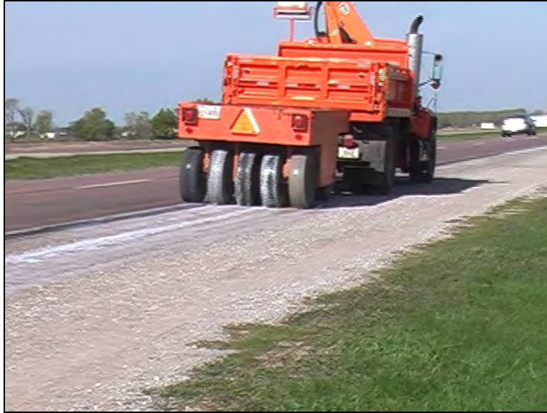
Figure 86. Compacting the shoulder section after three topical applications, April 28, 2005
