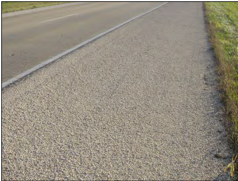
Figure 97. FA surface sealed using chip seal on I-35 milepost 150 northbound, September 1, 2005
