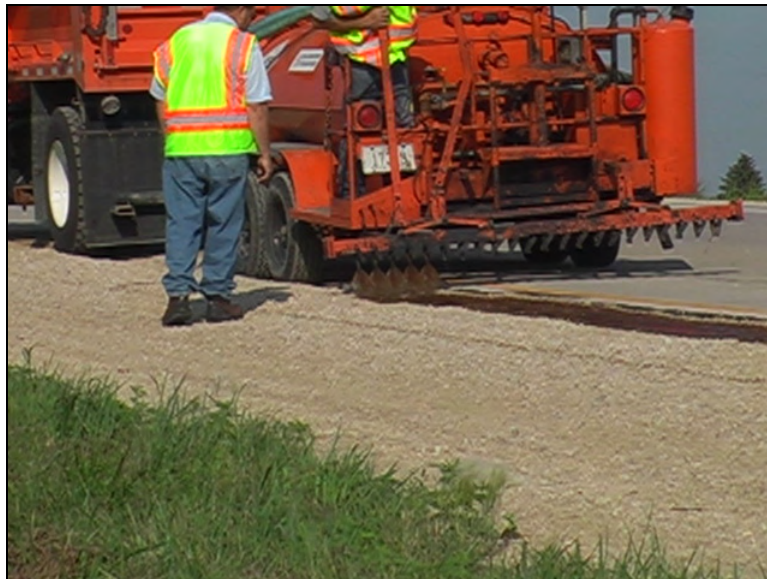
Figure 111. Applying Feed Energy soybean oil to the shoulder section, August 22, 2006
