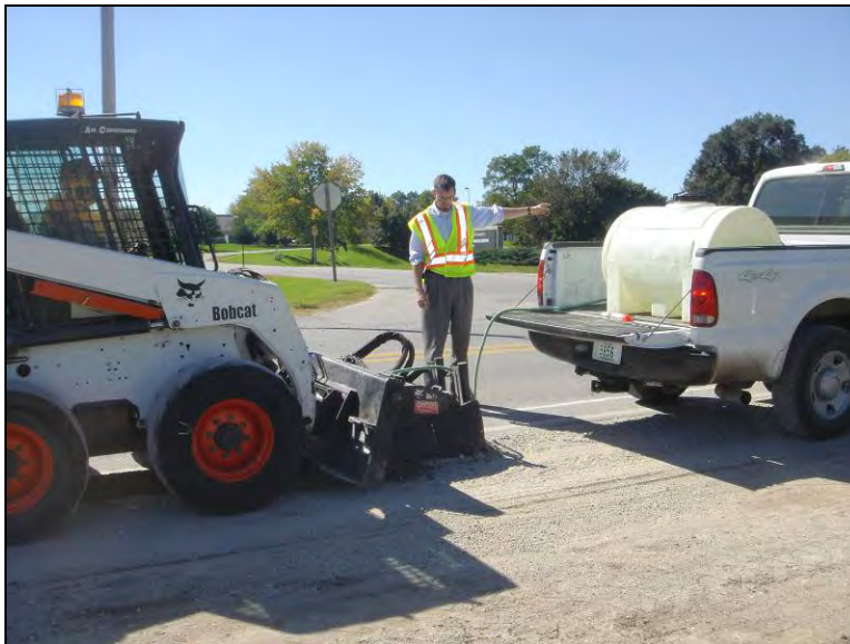
Figure 123. Truck carrying a water tank ahead of shoulder reclaimer, September 26, 2006
