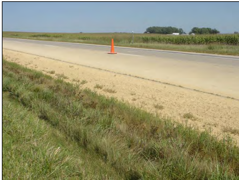
Figure 95. Fly ash added to the granular material on I-35 milepost 150 northbound, September 1, 2005
