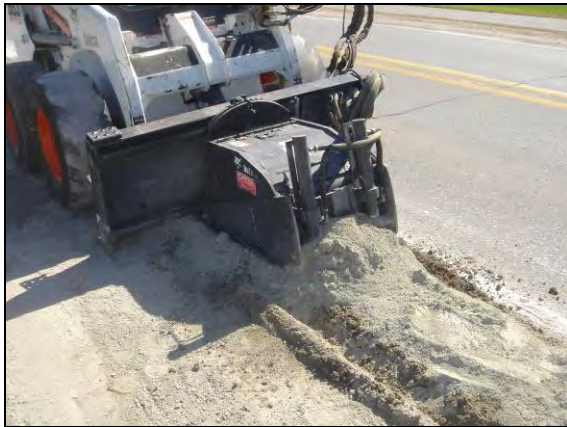
(a) Before reclamation
