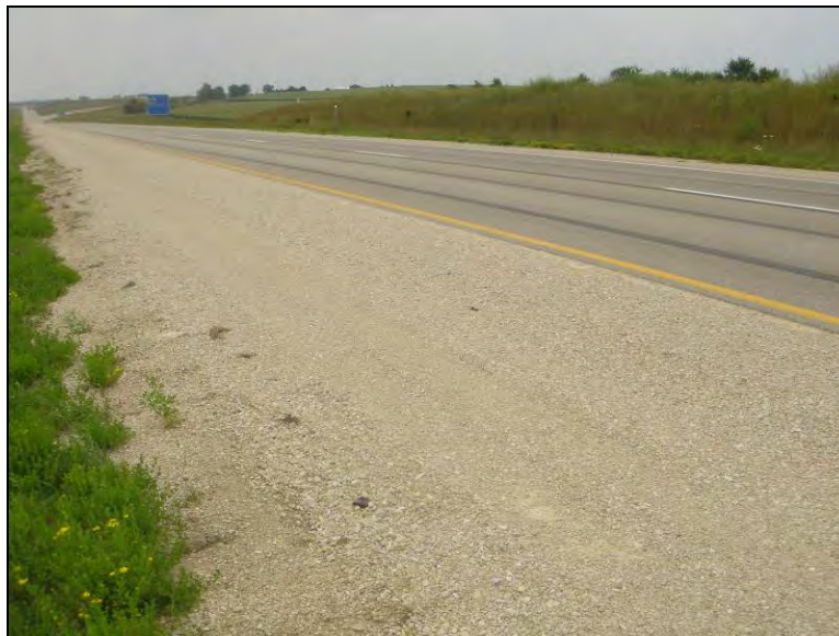
Figure 182. No rutting at the test section stabilized with BX1200, July 25, 2006
