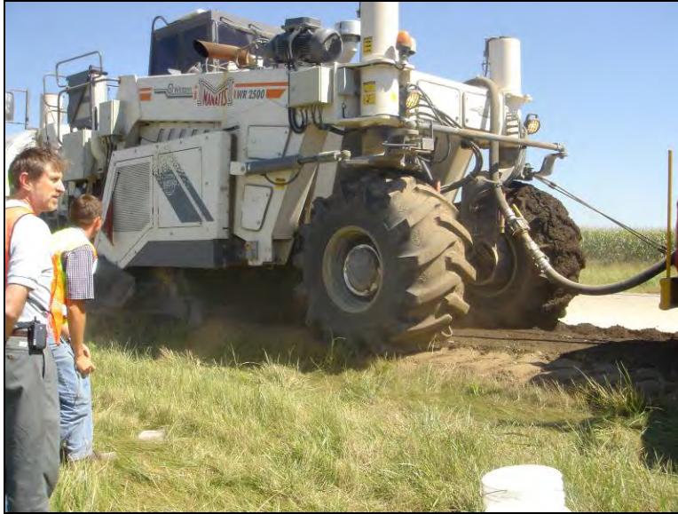
Figure 96. Full depth reclamation of FA on I-35 milepost 150 northbound, September 1, 2005
