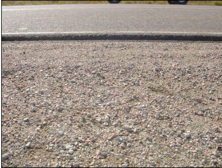
Figure 58. Granular shoulder section on Hwy IA 3 St. 940 W.B., October 14, 2005
