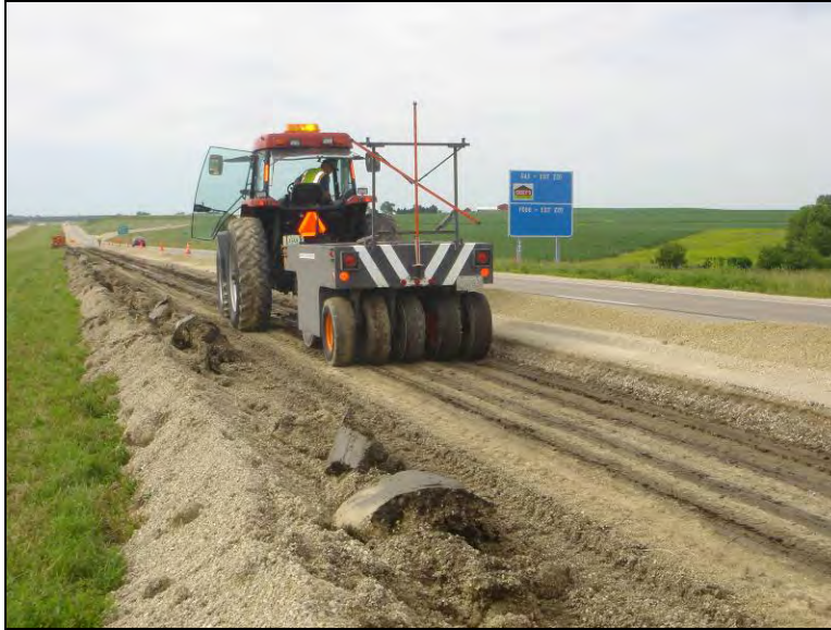
Figure 174. Pneumatic roller used to compact the subgrade, June 23, 2006
