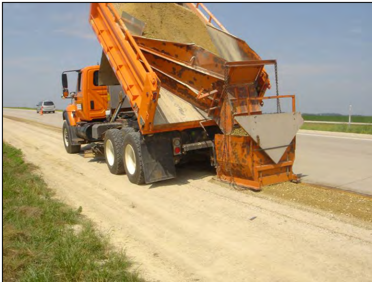
Figure 115. Placing crushed limestone material over the stabilized area, August 22, 2006
