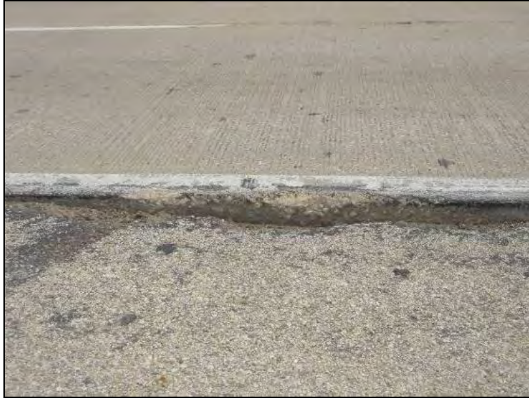
(a) Milepost 154 southbound
