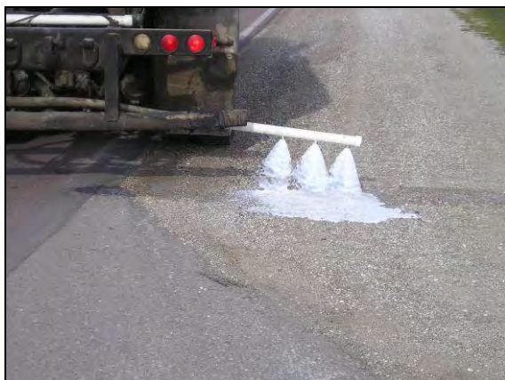
Figure 85. S.S. polymer topically applied to the granular shoulder, April 28, 2005
