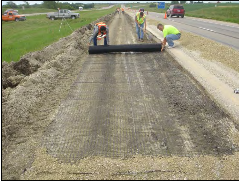
Figure 176. Rolling the BX 1200 geogrid over the soft subgrade layer, June 23, 2006
