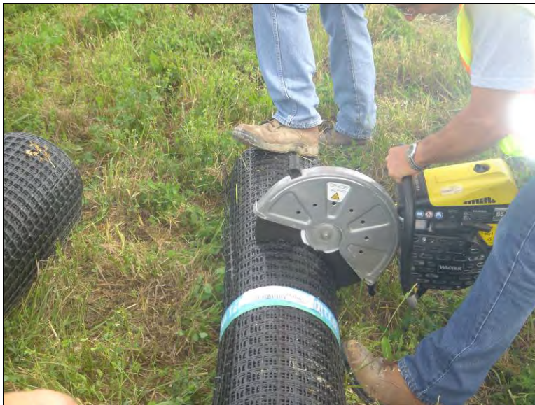
Figure 175. Cutting the geogrids to 8 ft. wide sections, June 23, 2006
