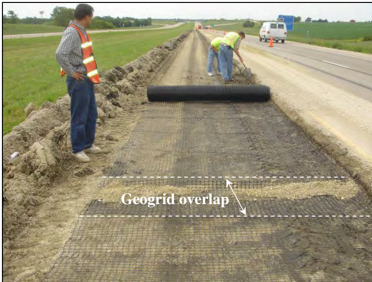
Figure 177. Overlapping geogrids in the direction of aggregate spreading, June 23, 2006
