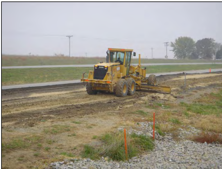
Figure 151. Motor grader used to recover windrowed aggregate, October 31, 2005
