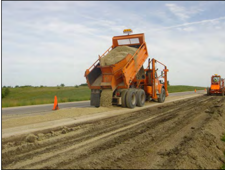
Figure 172. Placing virgin aggregate next to the test section, June 23, 2006
