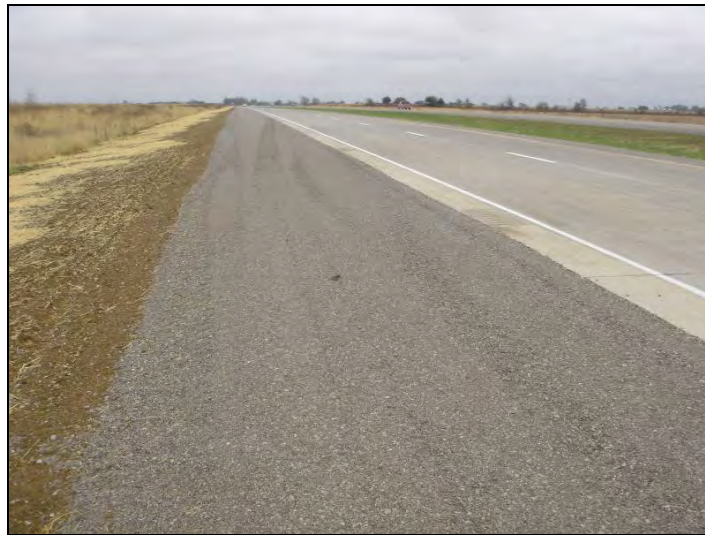
Figure 162. Newly constructed granular shoulder section, October 17, 2006
