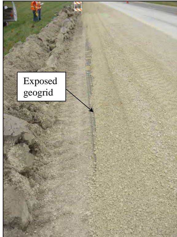
Figure 180. Exposed edges of the geogrid after construction was completed, June 23, 2006
