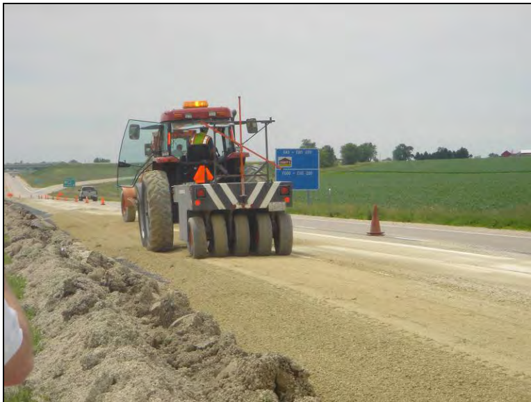
Figure 179. Compacting the granular layer using a pneumatic roller, June 23, 2006
