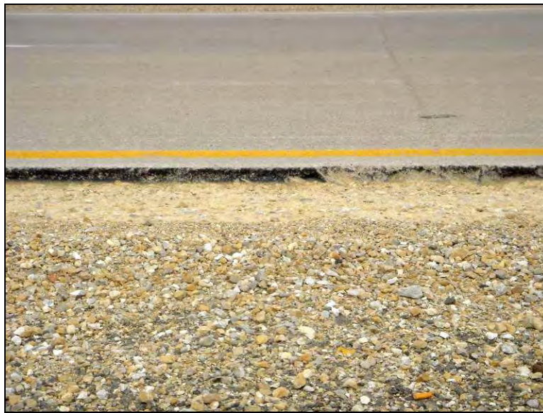
Figure 119. Three-inch edge drop-off after eight month on Hwy 18 milepost 202.50 near Rudd, IA, on June 23, 2006
