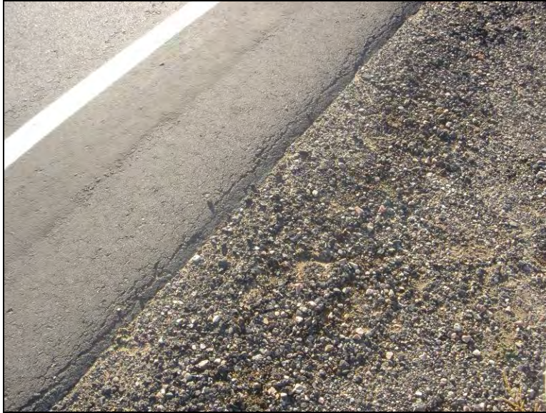
Figure 53. Granular shoulder with RAP material on Hwy IA 12 Station 1080+00', October 14, 2005
