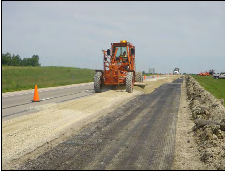
Figure 178. Spreading the new crushed limestone over the geogrid, June 23, 2006
