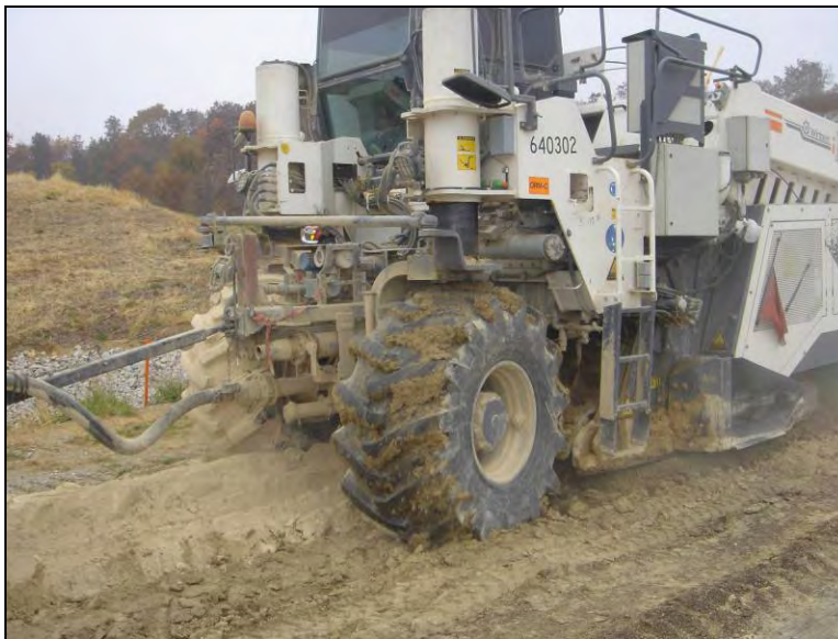
Figure 149. Mixing fly ash with subgrade soil using a road reclaimer, October 31, 2005
