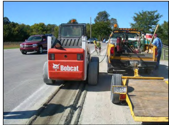
(b) After reclamation
