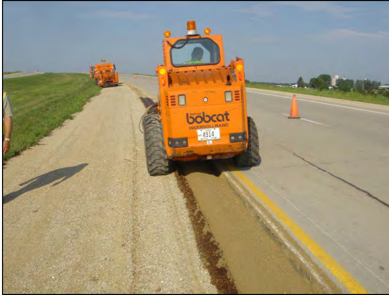
Figure 112. Mixing Feed Energy soybean oil with shoulder granular material, August 22, 2006
