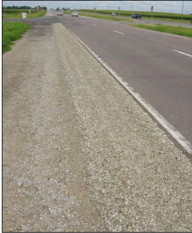
Figure 43. Granular shoulder section on Hwy 122, July 26, 2005
