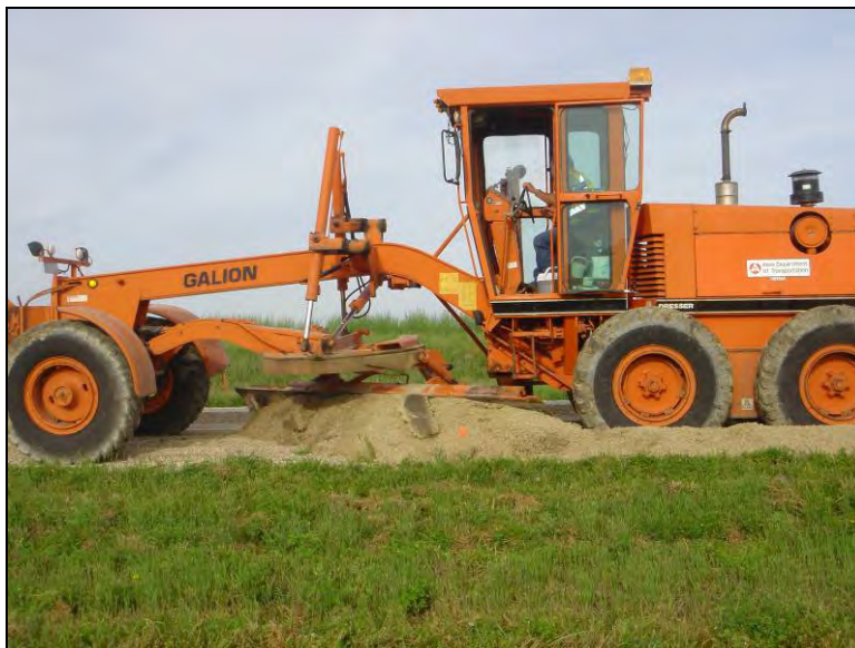
Figure 171. Motor grader removing the contaminated granular layer, June 23, 2006
