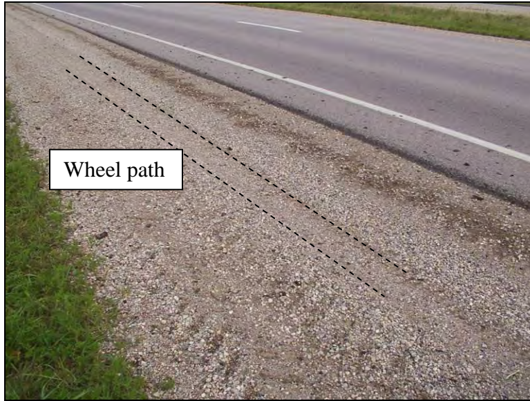
Figure 15. Granular shoulder section on U.S. 30 (milepost 160.25 E.B.), September 2, 2006
