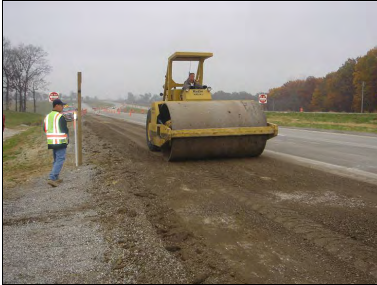
Figure 152. Smooth wheel roller used to compact the crushed limestone layer, October 31, 2005
