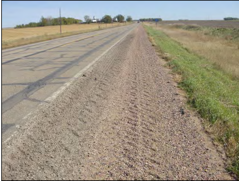
Figure 63. Granular shoulder section on Hwy 9 St. 135+00' W.B., October 14, 2005
