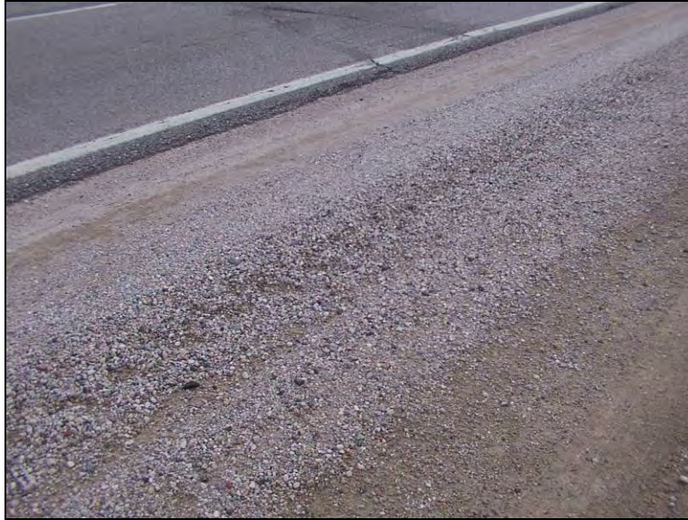
Figure 11. Shoulder section at U.S. 30 milepost 151.95 E.B., September 2, 2006
