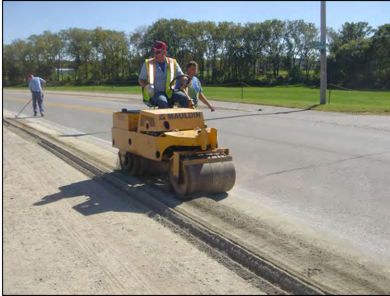
Figure 126. Compaction of stabilized section using smooth drum roller, September 26, 2006
