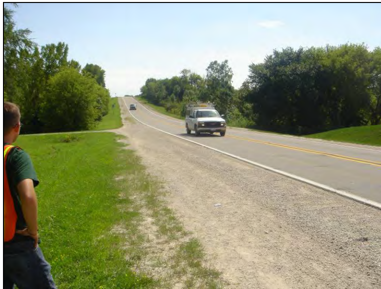
Figure 76. Aggregate shoulder section on State Ave., August 19, 2005
