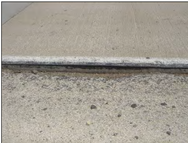
(b) Milepost 151 northbound
