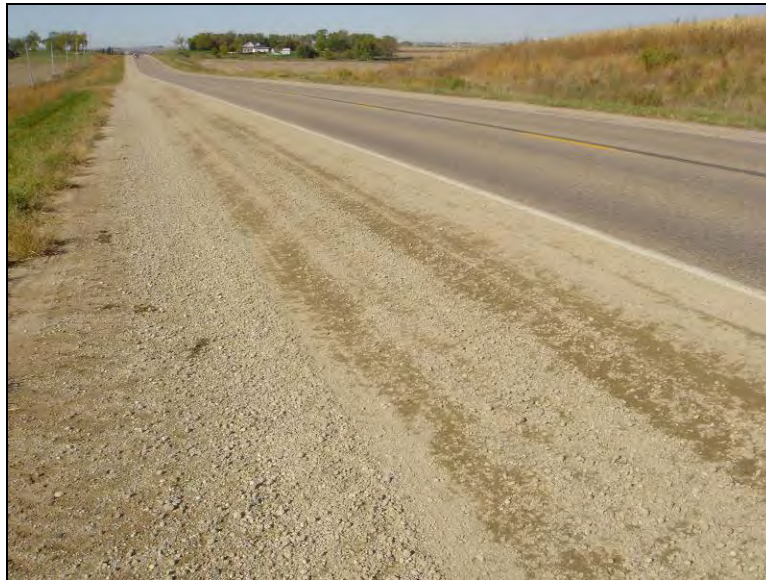
Figure 57. Granular shoulder section on Hwy IA 3 St. 940 E.B., October 14, 2005
