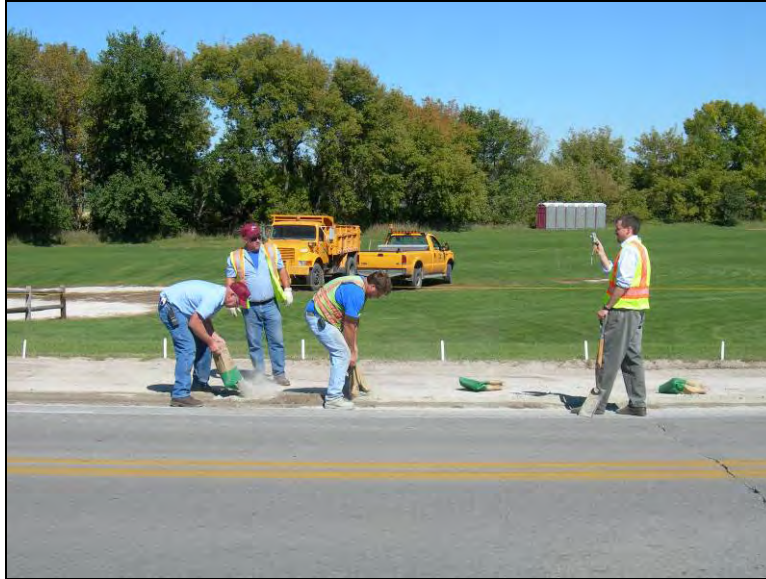
Figure 124. Spreading of cement over the reclaimed test section, September 26, 2006
