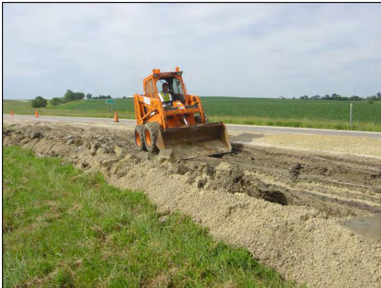
Figure 173. Skid loader leveling the subgrade, June 23, 2006
