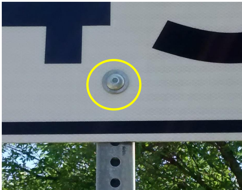
Figure 15. Sign theft prevention fastener
