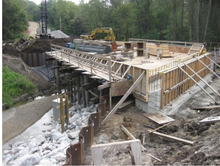
Figure 5-87. Construction of falsework for placement of bridge deck
