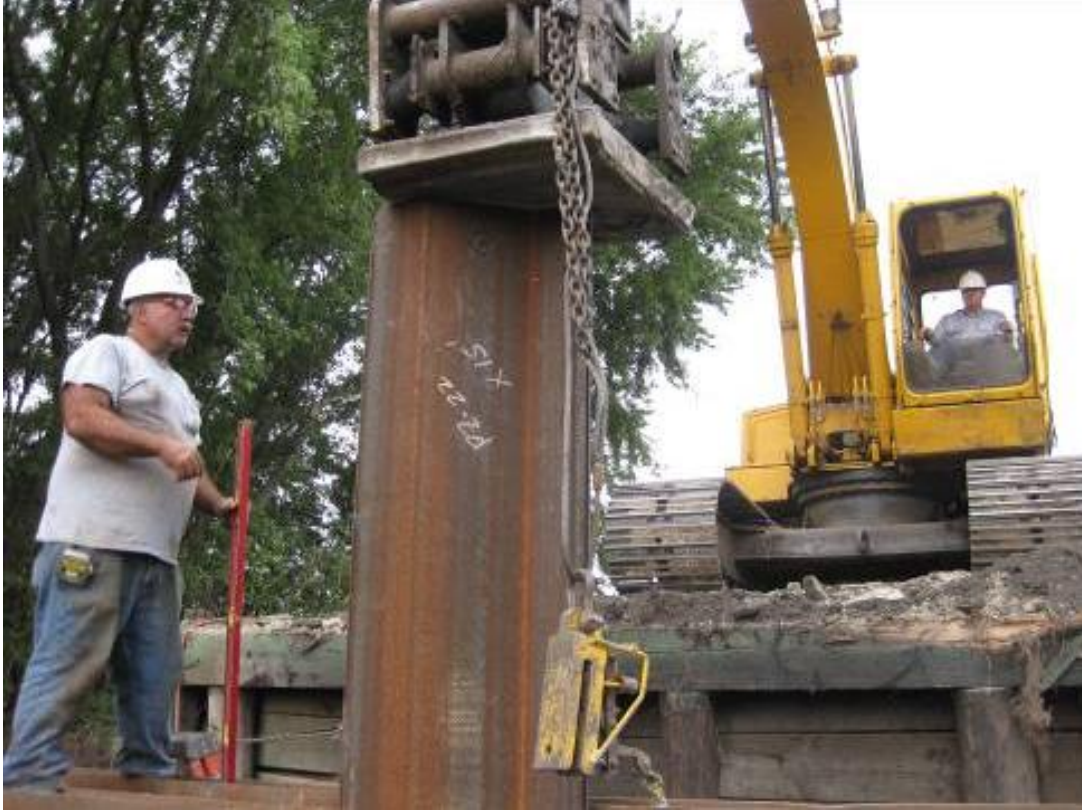
Figure 5-13. Driving of sheet pile sections with vibratory plate equipped excavator boom
