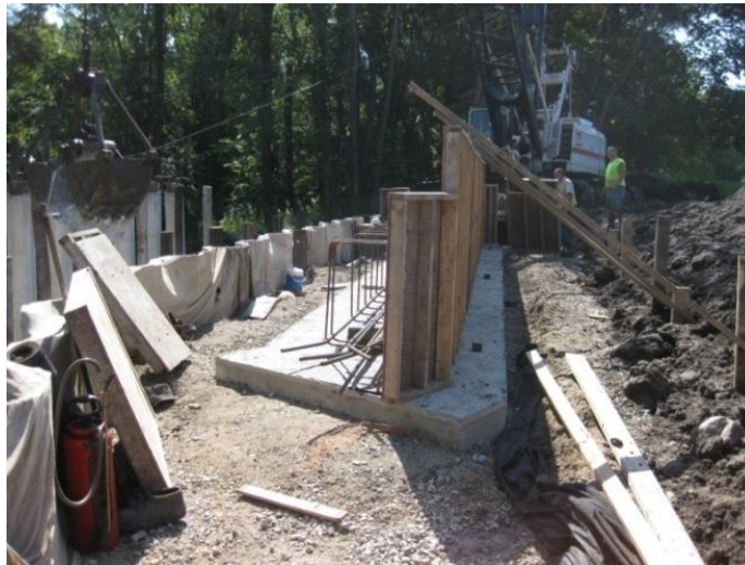
Figure 5-83. Reinforced concrete spread footing on west abutment
