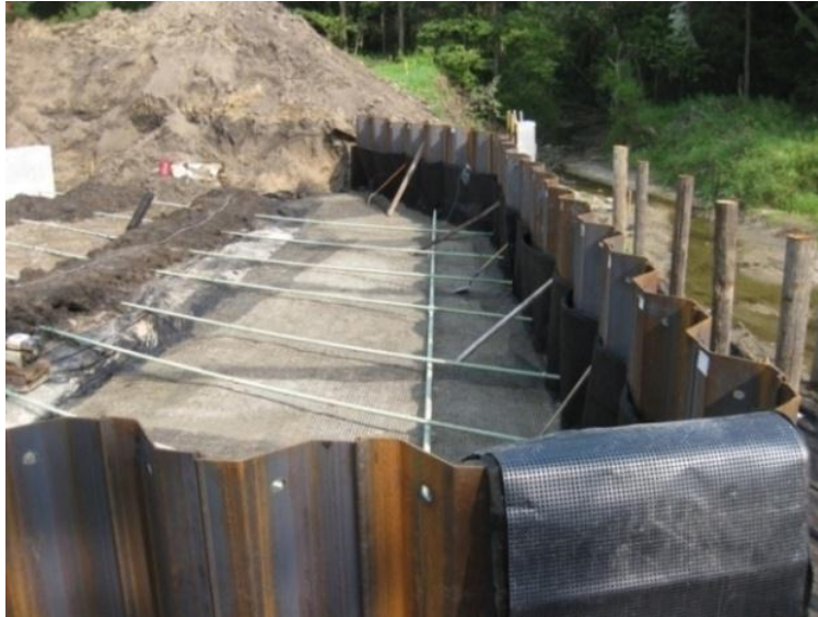
a.) Deadman and tie rods anchoring the west abutment sheet pile wall
