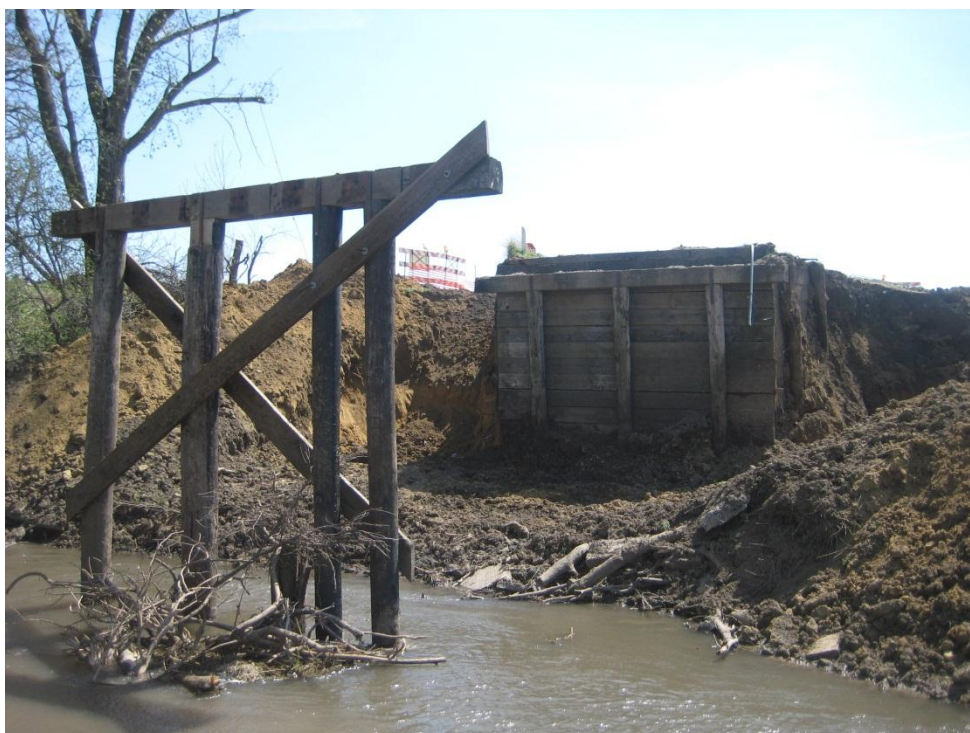
Figure 5-128. Partial demolition of existing bridge (April 14, 2010)
