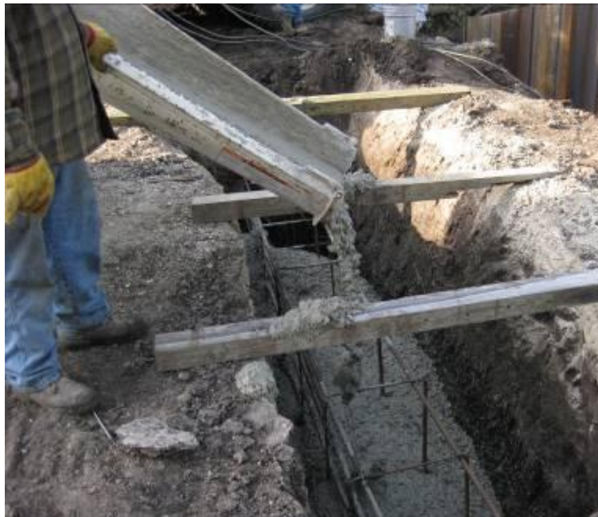
Figure 5-19. Reinforced concrete deadman placement behind east abutment
