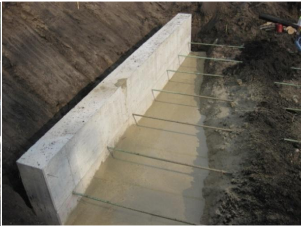
b.) Placement of flowable grout
