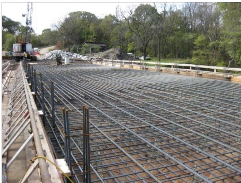
Figure 5-88. Reinforcement in place for continuous concrete slab bridge
