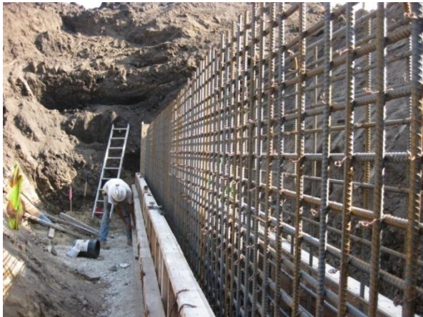
b.) Reinforcement and formwork being placed
