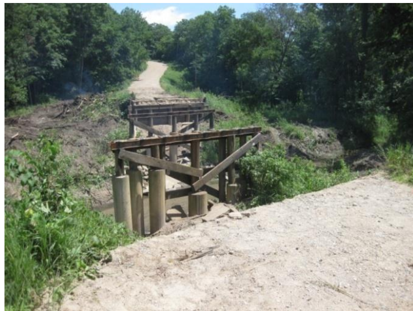
b.) Superstructure removed
