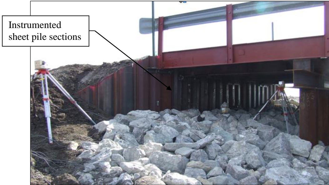
a.) View of abutment and pier
