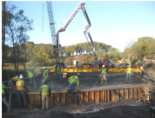
Figure 5-89. Concrete pumping for continuous concrete slab
