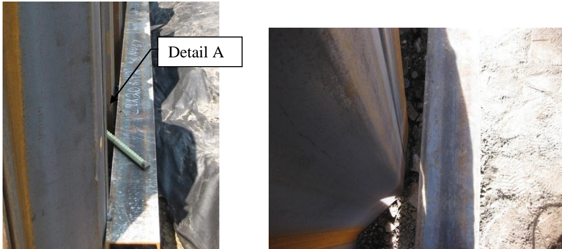
a.) Bottom waler channel welded to sheet pile wall
