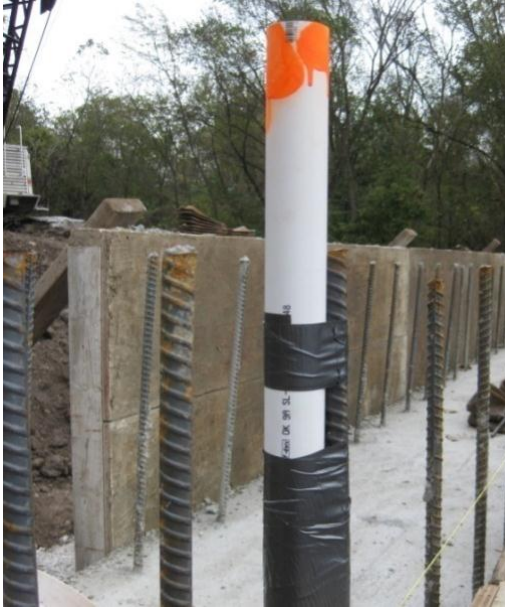
a.) Before placement of the bridge deck
