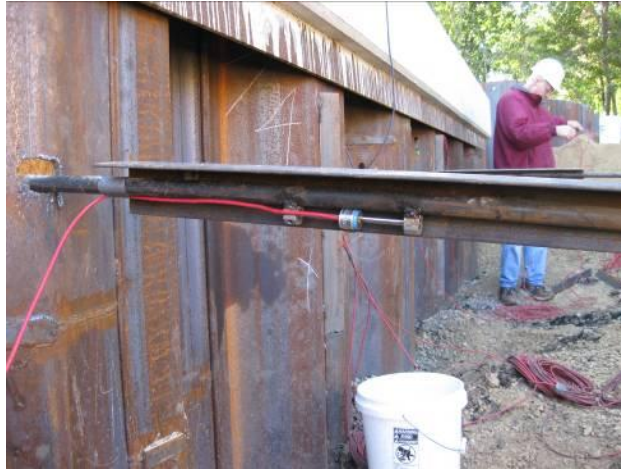
Figure 5-23. Tie rod strain gage installation
