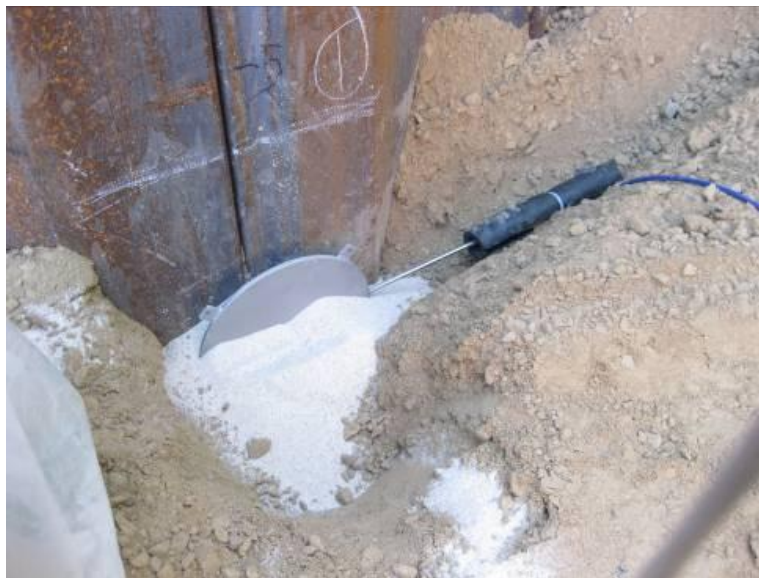
Figure 5-24. Earth pressure cell installation
