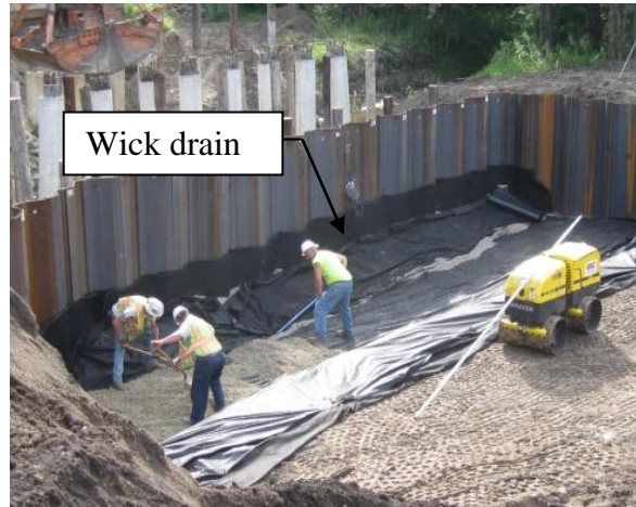
a.) Engineering fabric placement
