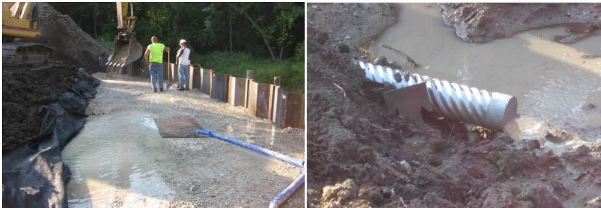
a.) Pumping water from stream
