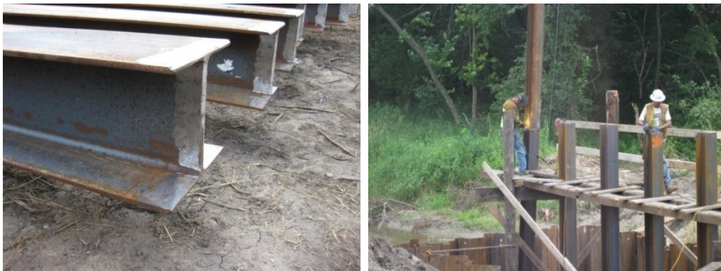
a.) Preparation of piles for welding b.) Welding two 40 ft sections together
