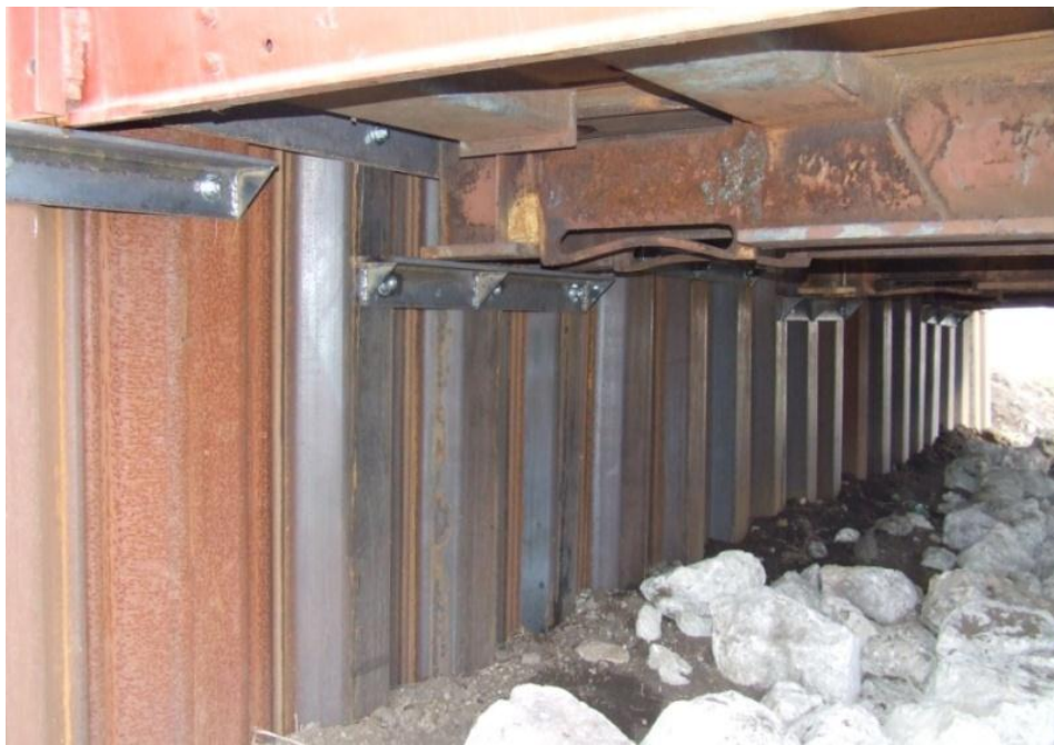
b.) Stiffened angles bolted to piling supporting superstructure
