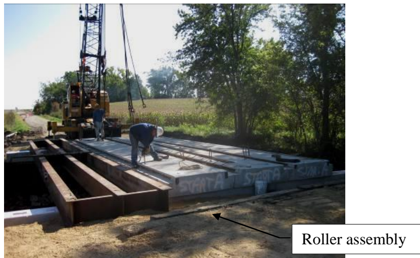
Figure 5-29. Roller assembly used to assist in placement of deck elements
