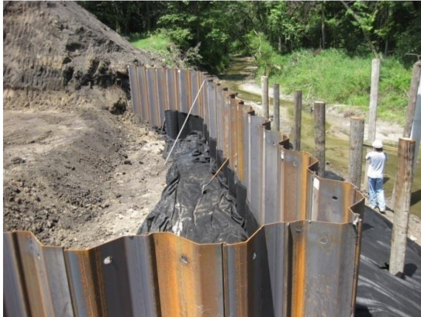
Figure 5-67. West abutment after all sheet piling in place
