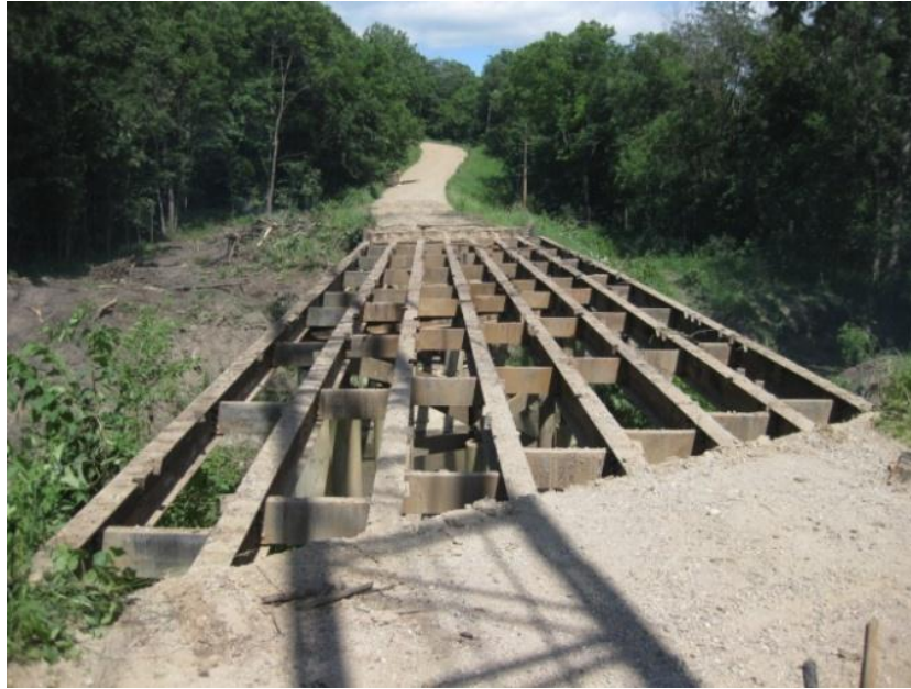
a.) Timber decking removed (exposing steel girders)
