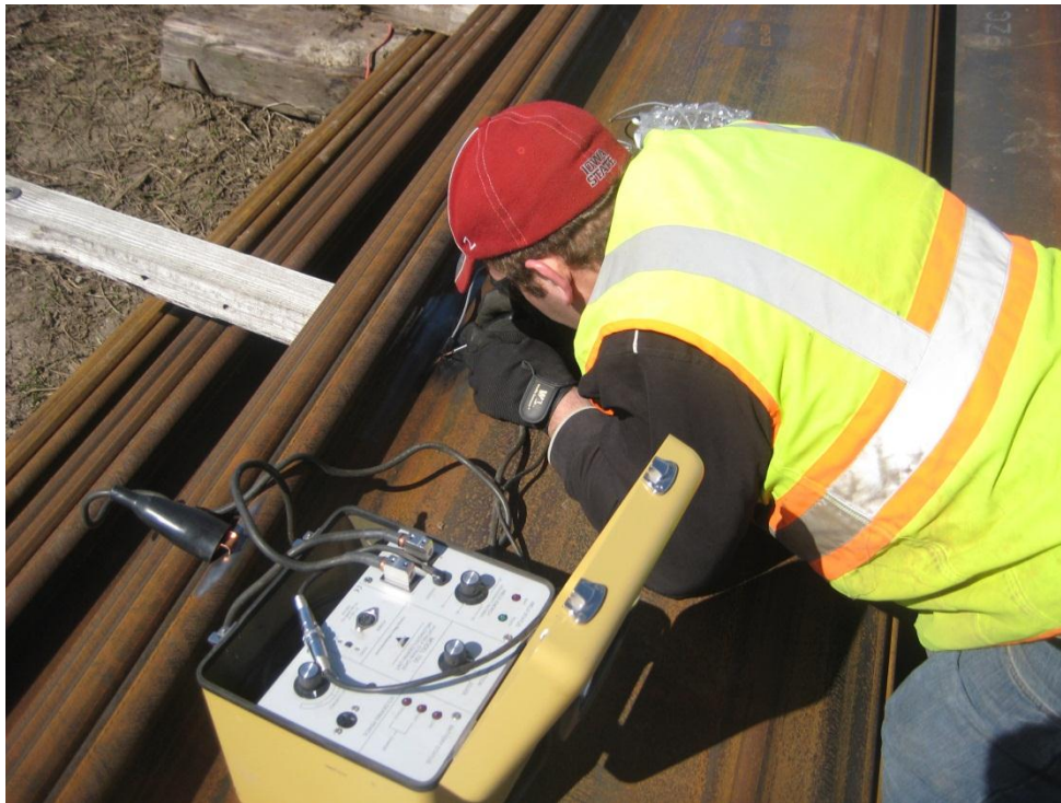
Figure 5-127. Sheet pile being instrumented (March 23, 2010)
