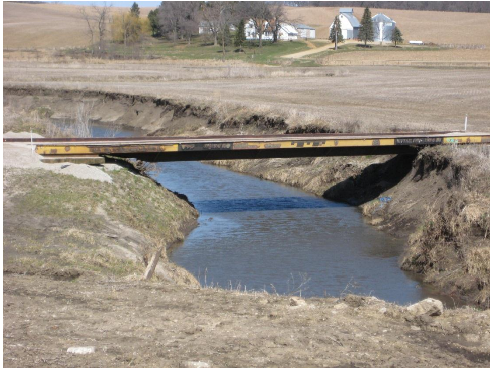
Figure 5-126. Temporary flat car bridge (March 23, 2010)
