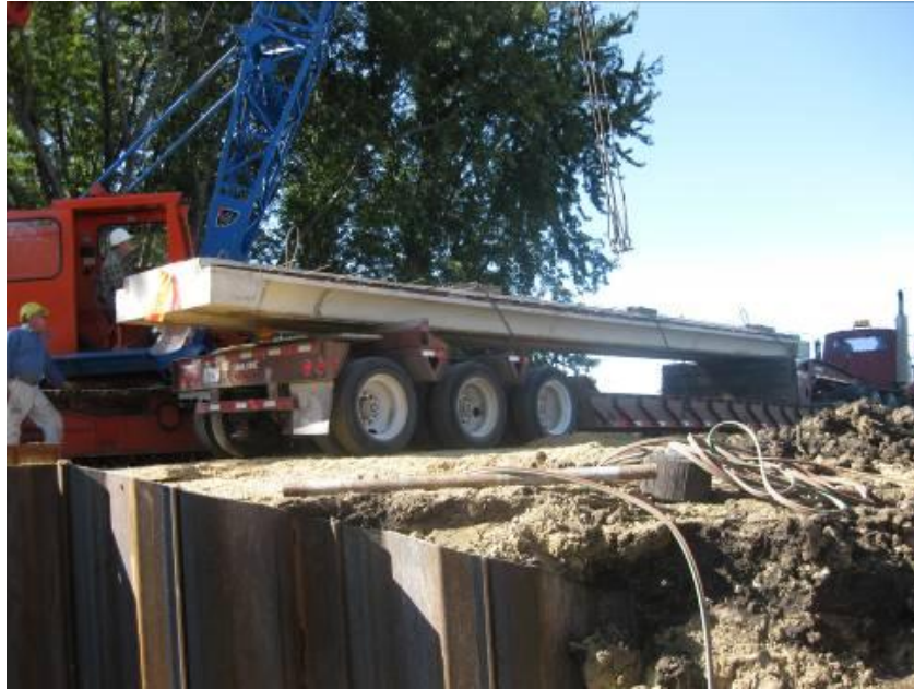
Figure 5-28. Precast beam-in-slab bridge deck element
