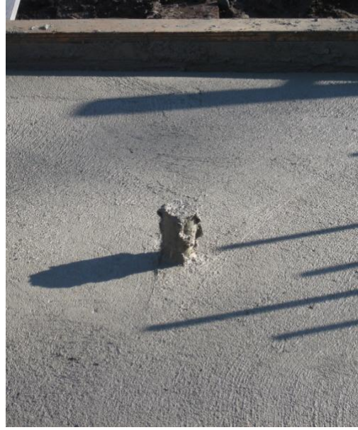
b.) After placement of the bridge deck
