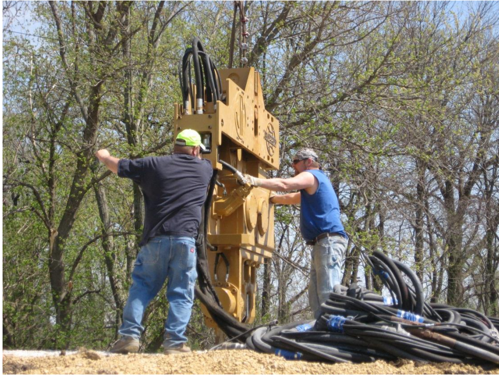
Figure 5-129. Pile driving equipment (April 14, 2010)
