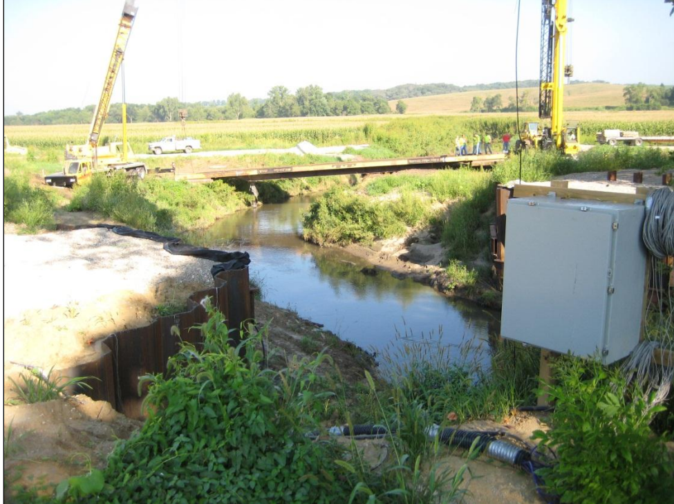
Figure 5-131. Lifting temporary deck into place (August 13, 2010)
