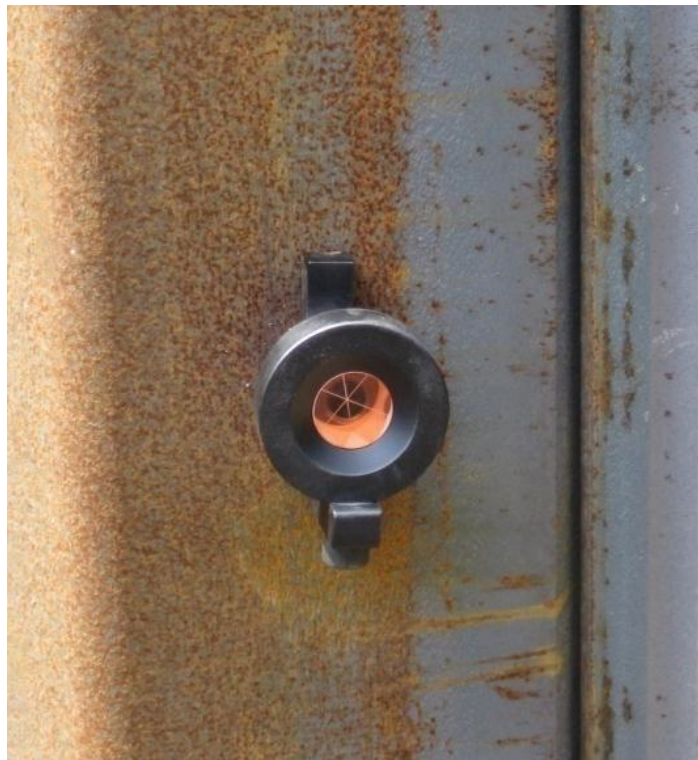
Figure 5-99. Prisms for surveying displacement of sheet pile wall
