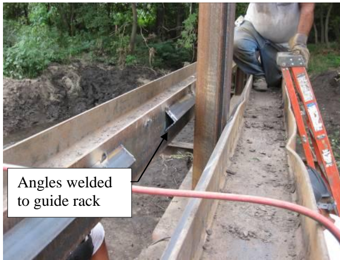
a.) Guide rack with angles attached
