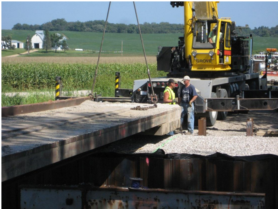
Figure 5-132. Setting flat car on sheet pile abutments (August 25, 2010)
