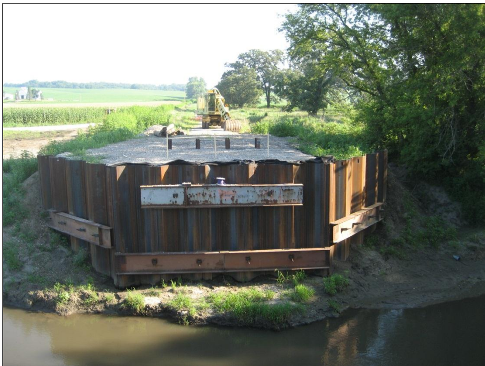
Figure 5-130. Completed abutment looking south (July 27, 2010)
