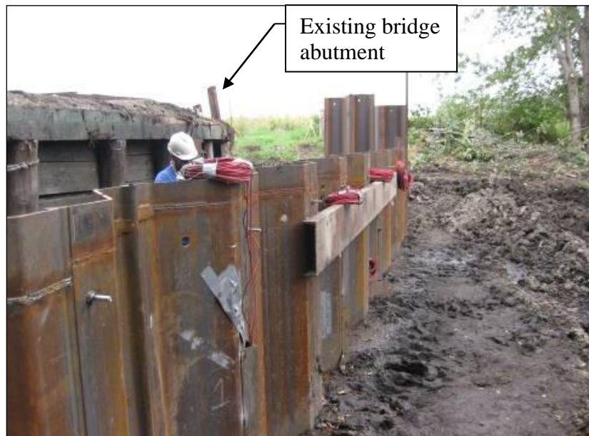
Figure 5-27. West abutment of previous bridge remained in place (behind wall)
