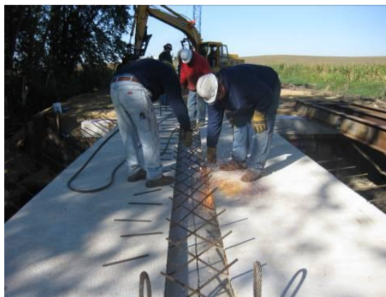
Figure 5-31. Finishing of bridge deck joints
