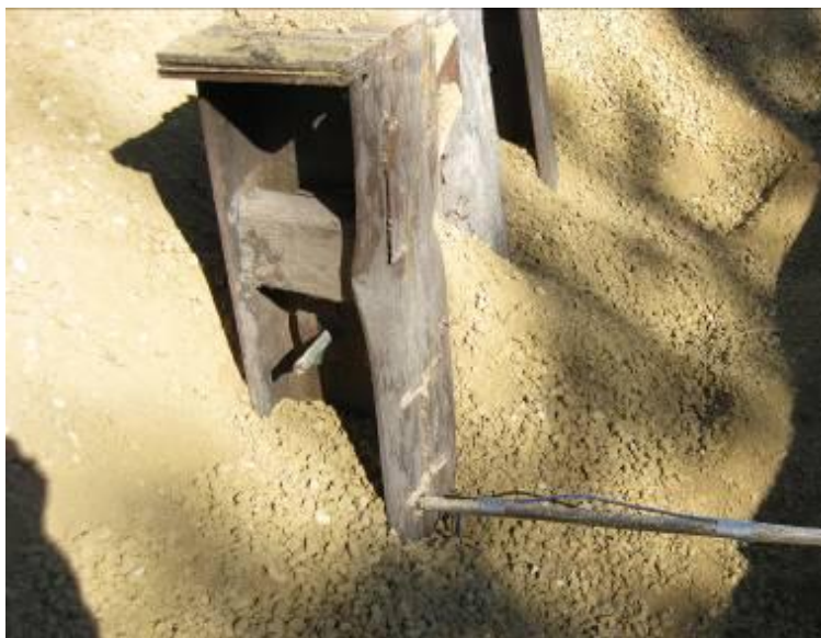
Figure 5-21. Tie rod to H-pile connection
