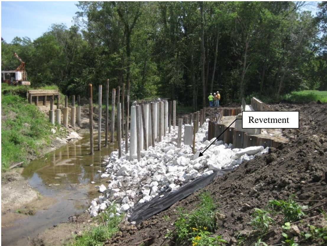
Figure 5-86. Finished west abutment and pier
