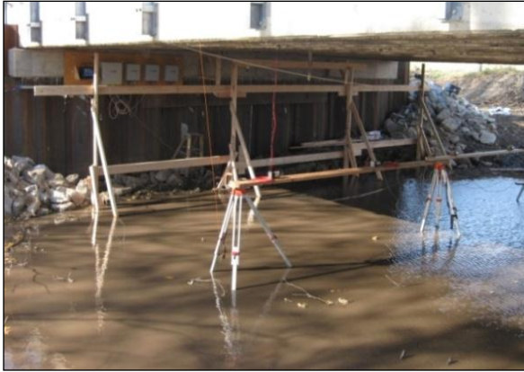
a.) View of west abutment
