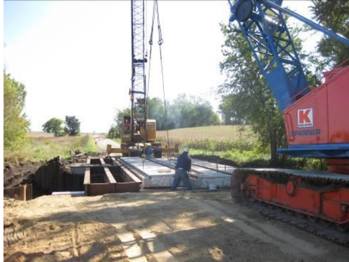
Figure 5-30. Dual crane operation for placement of bridge superstructure
