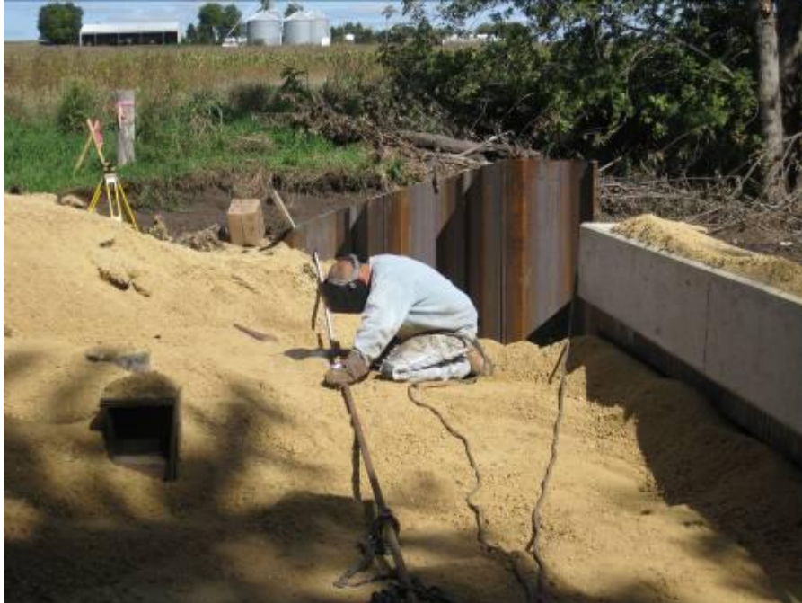
Figure 5-20. Installation of wingwall tie
