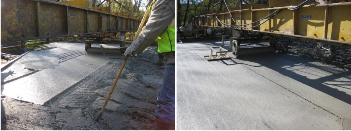
a.) Unfinished concrete after placement
