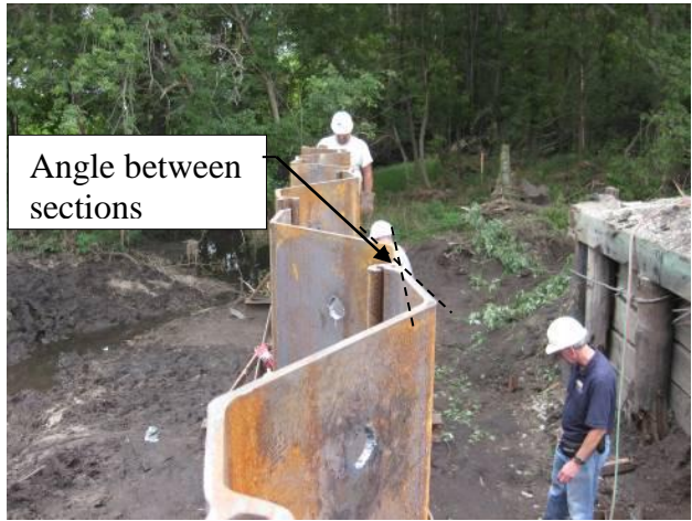
a.) Angle between sections
