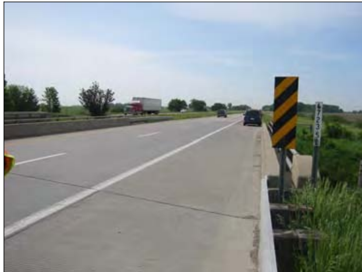
Figure 85. Recently replaced bridge approach slab (SBL)
