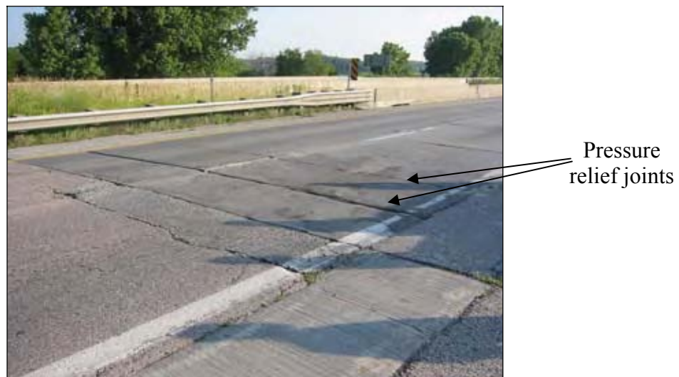
Figure 106. Pressure relief joint made by cutting the approach slab
