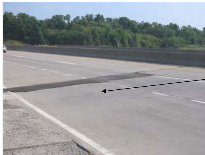
Figure 165. Differential settlement at approach slab
