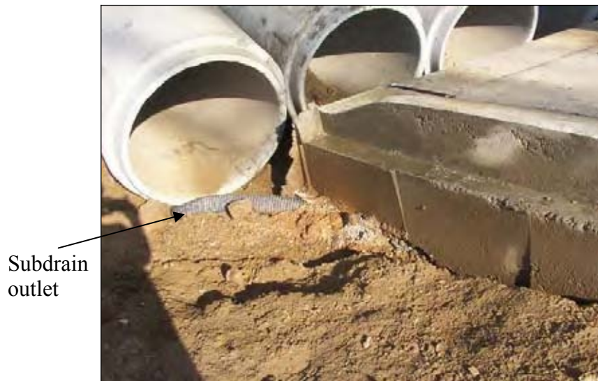
Figure 214. Subdrain outlet at the bottom of the embankment
