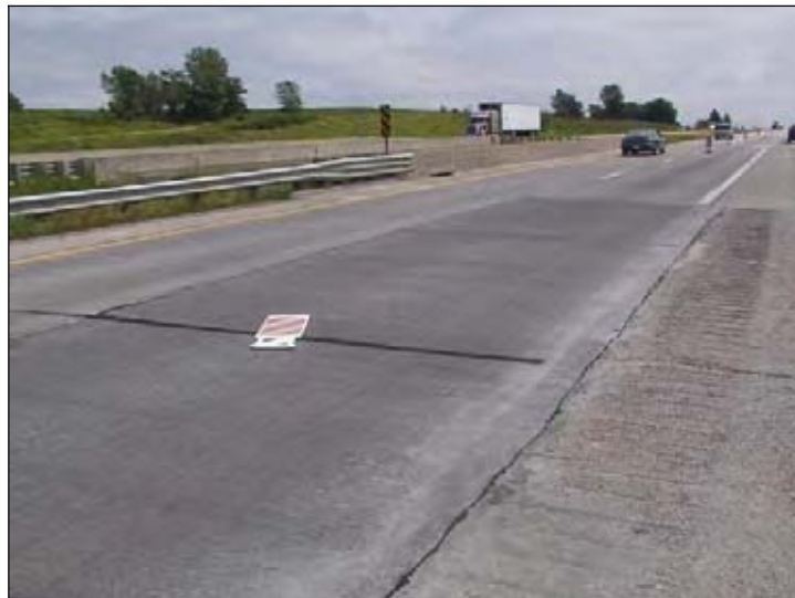
Figure 136. Replaced bridge approach slab
