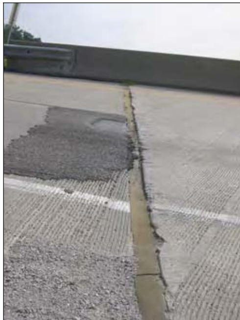
Figure 167. Flexible foam used as joint filler
