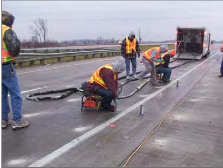
Figure 259. Injecting high-density polyurethane under the approach slab
