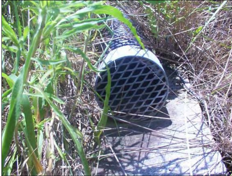
Figure 242. End drain in a satisfactory condition (South end of SBL)
