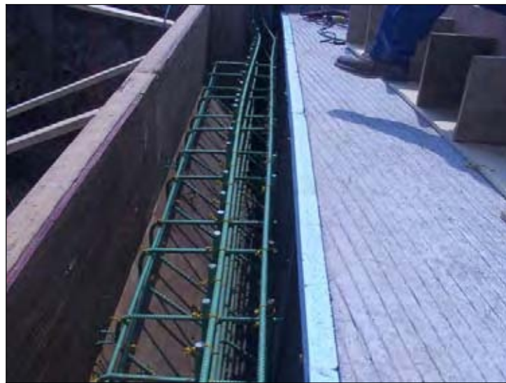
Figure 238. Abutment reinforcement (North end of NBL)
