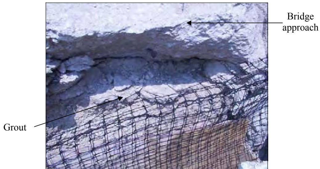
Figure 236. Grout pumped under existing approach (South end of SBL)
