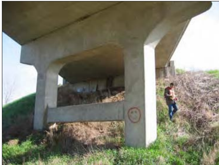
Figure 62. Concrete bridge with deep slab and no girders
