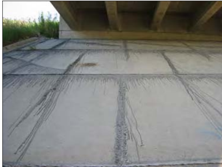
Figure 116. Sealed concrete slope protection cover
