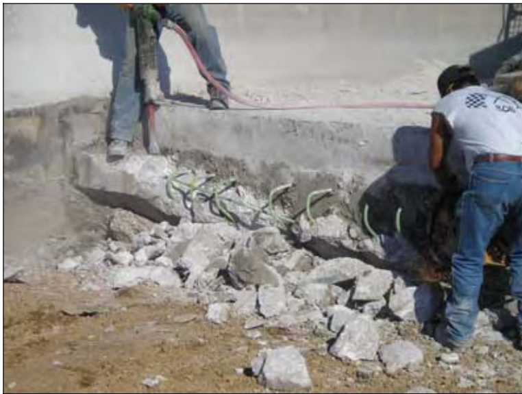
Figure 293. Tearing down the old pavement notch (South end of SBL)
