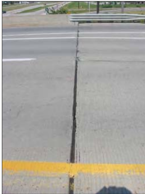
Figure 126. Expansion joint 2 inches wide and in good condition
