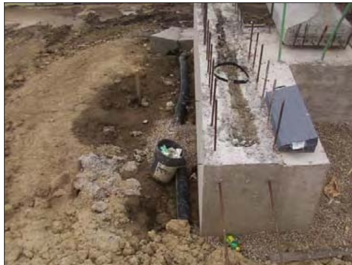
Figure 187. Subdrain along the side of the abutment
