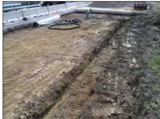
(b) Trench excavated to connect the subdrain to the end drain
