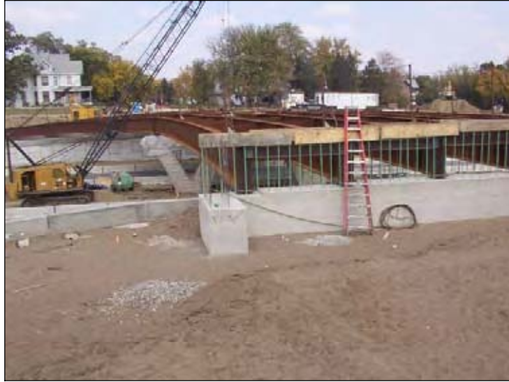
Figure 209. Construction of steel girders and backwall
