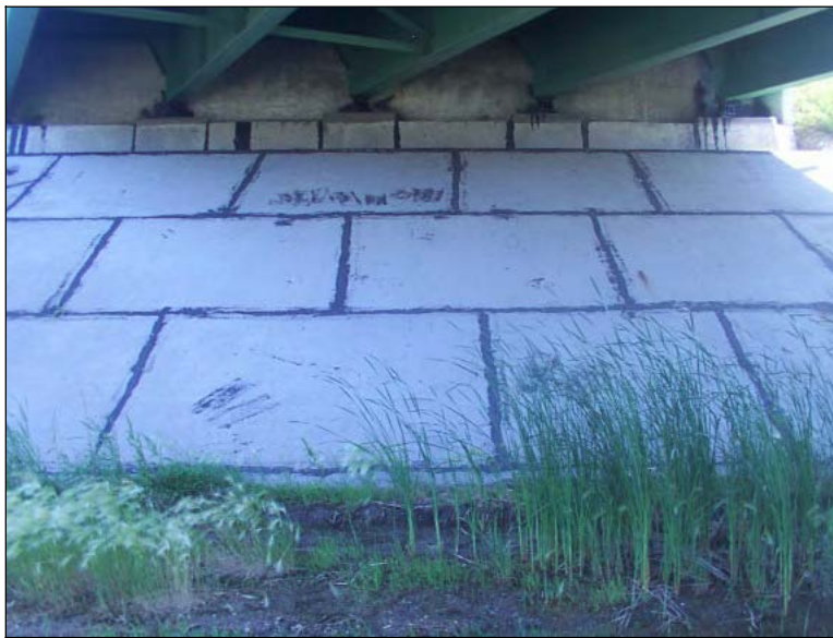
Figure 321. Bridge embankment in a satisfactory condition
