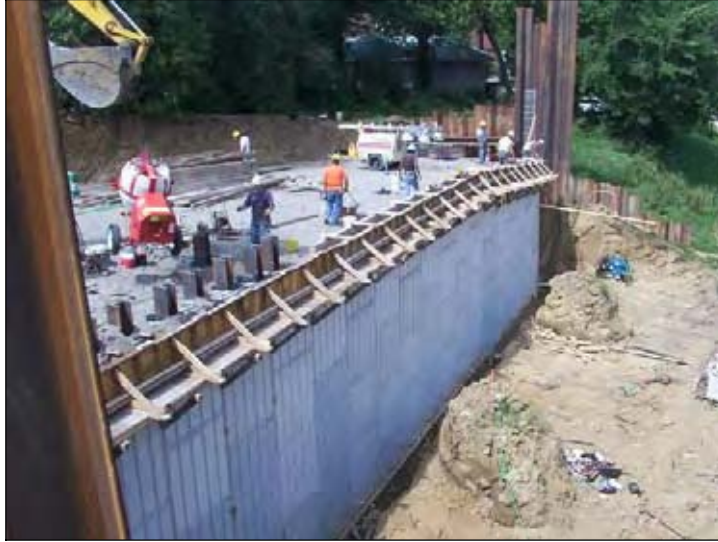
Figure 196. Construction of retaining wall (South end of NBL)
