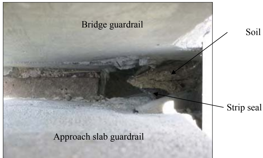
Figure 99. Top view of the strip seal cut short (North bound)
