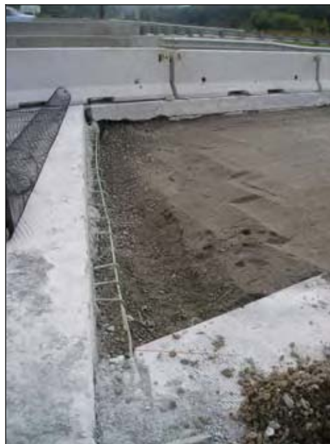
Figure 277. Compacted special backfill (South end of SBL)
