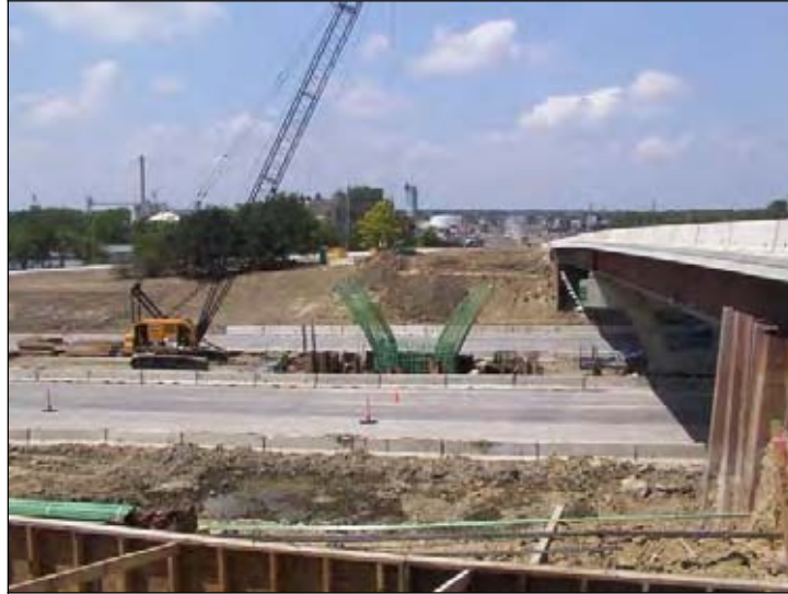
Figure 222. Construction of the southbound bridge
