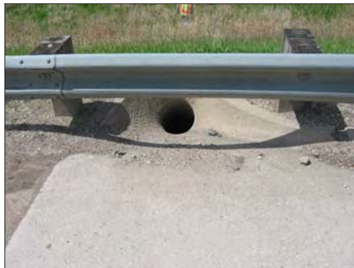
Figure 81. Surface drainage inlet at the bridge approach
