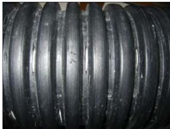
(b) Closer view of pipe openings
