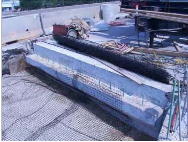
Figure 237. Construction of new bridge approach (South end of NBL)
