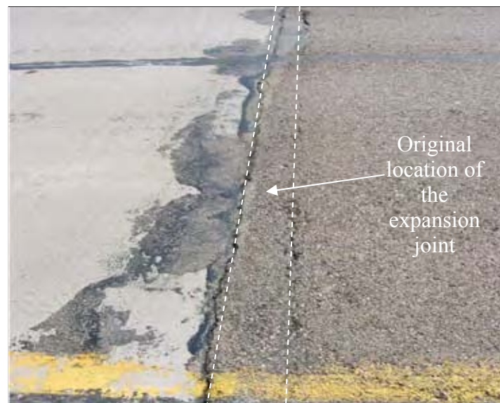
Figure 75. Asphalt overlay covering the expansion joint at the bridge approach
