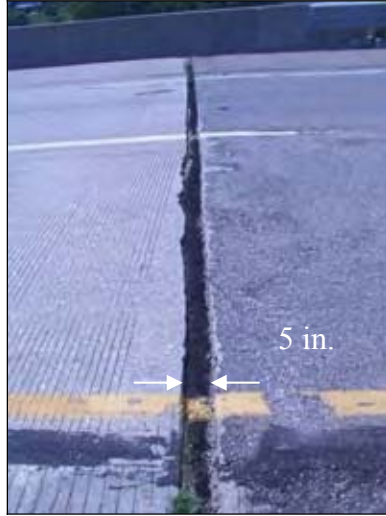
Figure 302. Recycled tires used as joint filler
