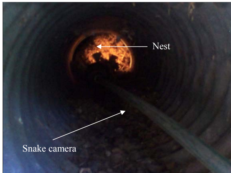
Figure 290. Rodent nest blocking the subdrain at 5 feet from the outlet
