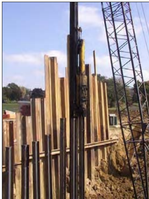
Figure 199. H-piles being driven
