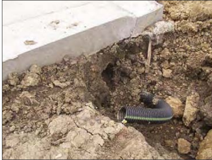
Figure 186. Subdrain outlet at the bottom of the embankment
