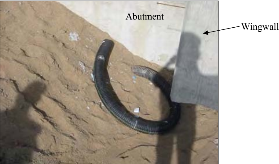
Figure 231. Granular backfill surrounding the subdrain
