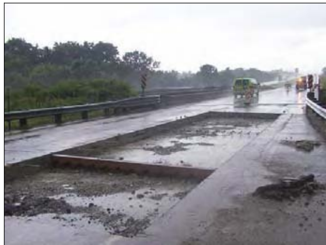
Figure 130. Bridge approach panel removed for replacement
