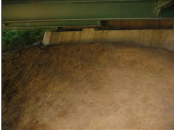
Figure 114. Loess soil used for the embankment
