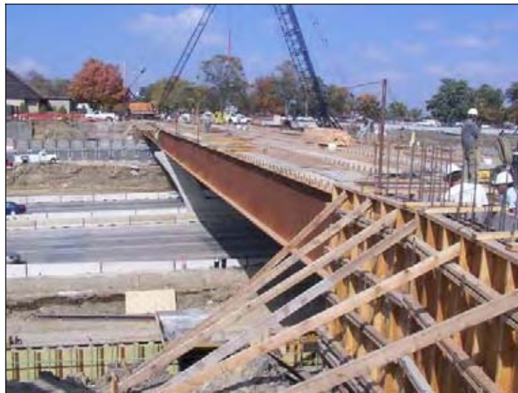
Figure 216. Construction of bridge slab (NBL)
