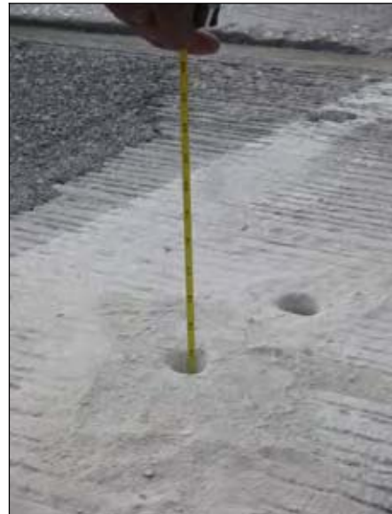
(b) Measuring the void
