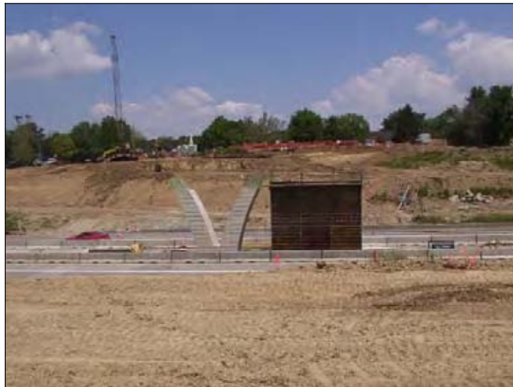
Figure 212. Construction of center pier
