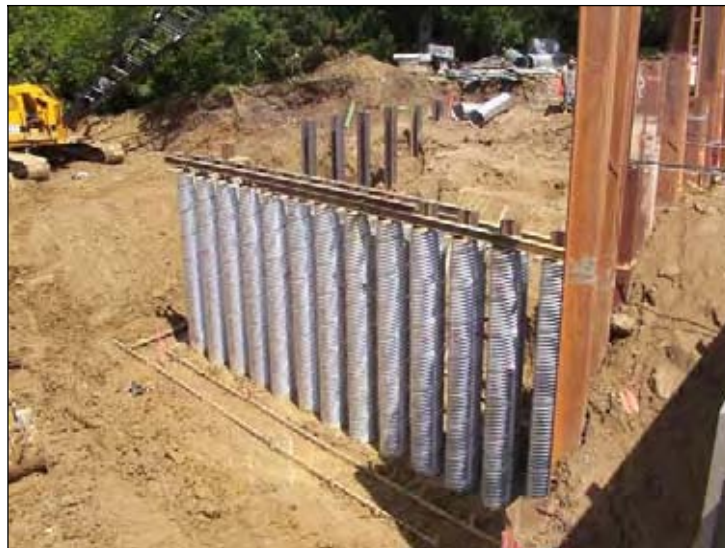
Figure 195. Installation of H-Piles (North end of NBL)
