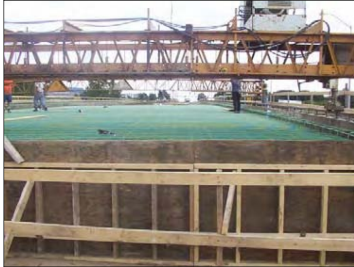
Figure 220. Construction of bridge slab
