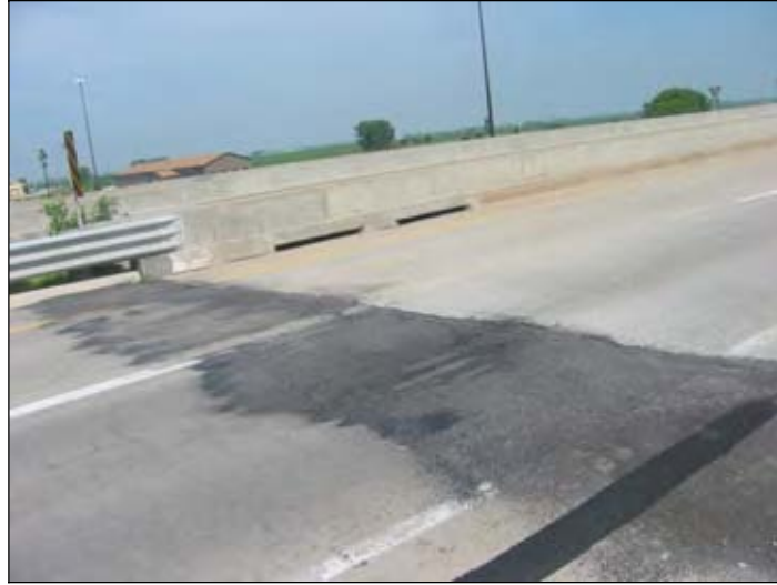
Figure 125. Asphalt patch placed at the approach slab
