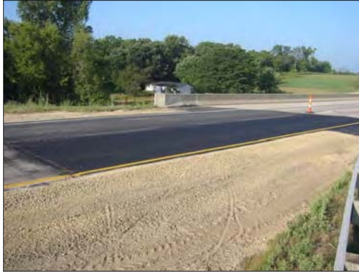
Figure 161. Approach slab asphalt overlay
