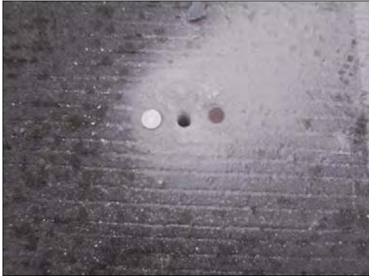
Figure 257. Holes drilled for injecting expansive material under the approach
