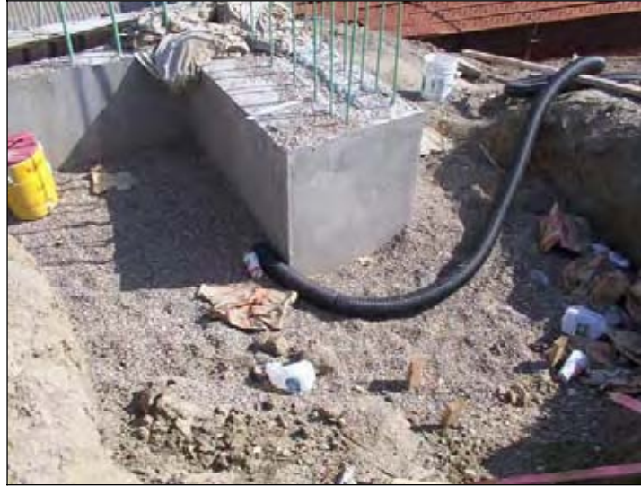
Figure 228. Constructed bridge backwall with visible subdrain surrounded by porous backfill
