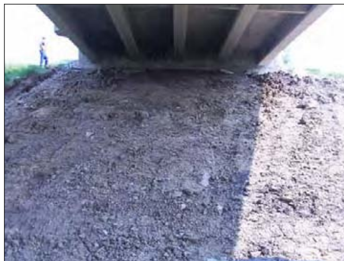
Figure 147. Bridge embankment prior to placing the new overlay
