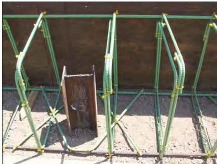
Figure 225. H-pile embedded in the bridge backwall
