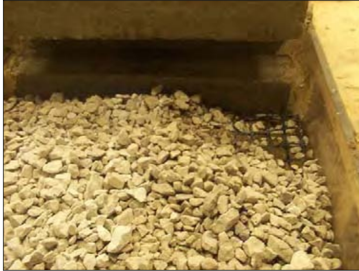
Figure 359. Geogrid placed between the granular and special backfill
