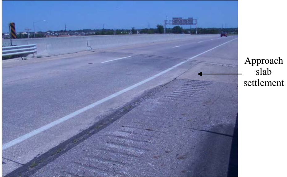
Figure 318. Settlement of bridge approach (North end of SBL)
