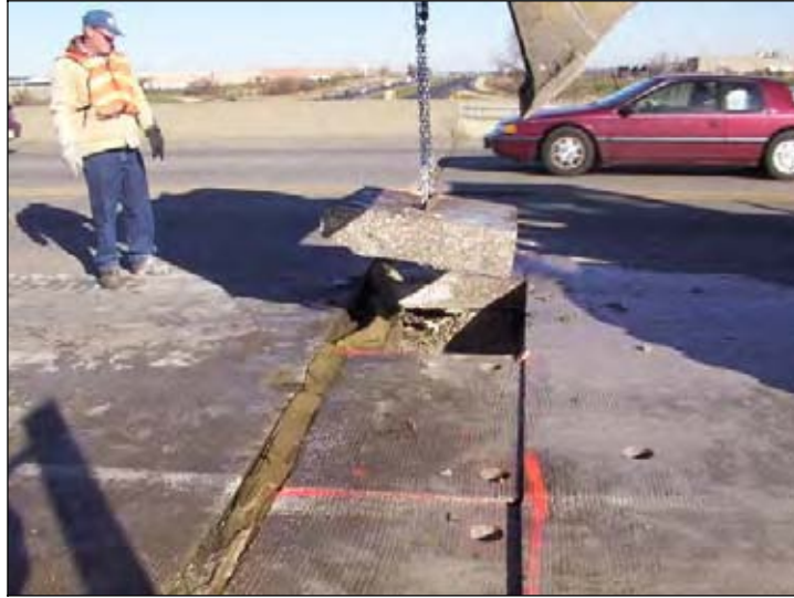
Figure 55. Removing a segment of the bridge approach
