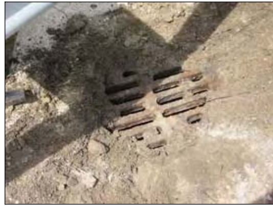
(b) Bridge approach surface drain after debris removal
