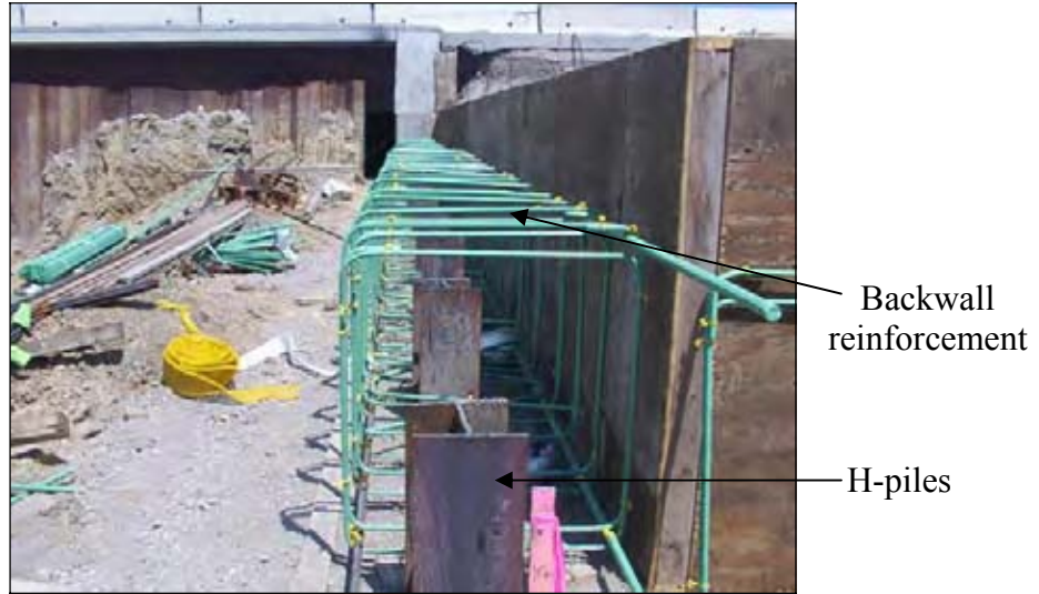
Figure 224. Reinforcement for the bridge backwall
