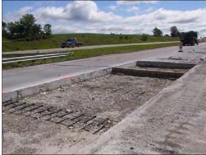
Figure 133. Replacing the bridge approach slab section
