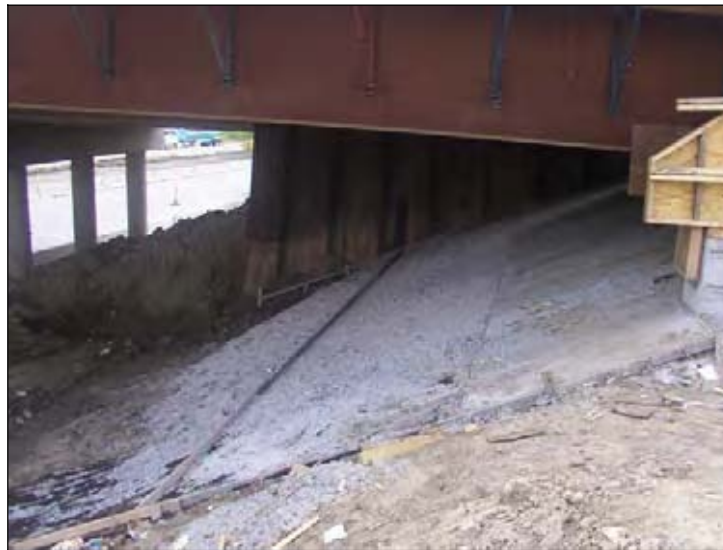
Figure 221. Construction of slope protection at the embankment
