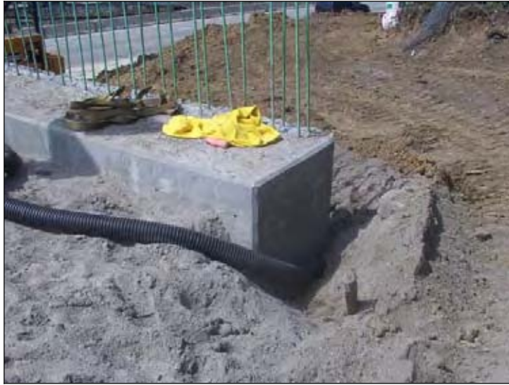
Figure 198. No porous fill surrounding the subdrain (North end NBL)
