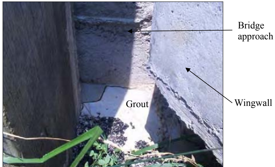
Figure 152. Grouting under the approach slab (South end of NBL)
