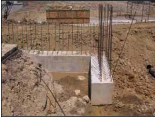
(a) Backwall construction
