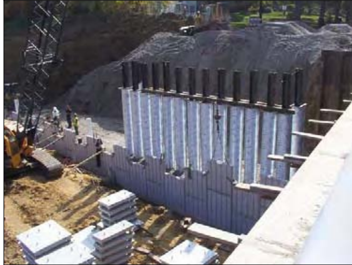
Figure 200. Construction of the retaining wall (South end of SBL)
