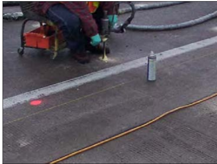
Figure 260. Steady injection until material leaks out of hole
