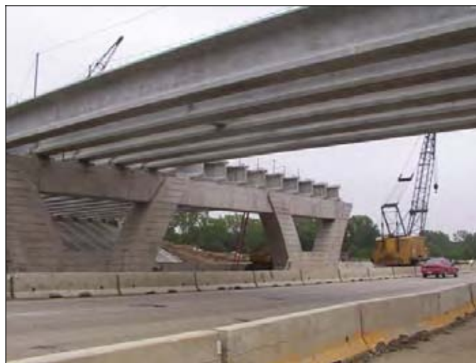
Figure 183. Girders under construction (NBL)
