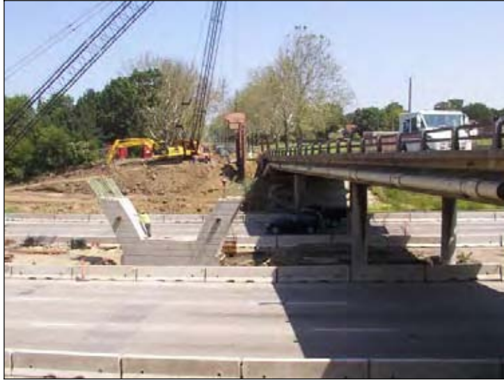
Figure 192. Construction of the new northbound bridge
