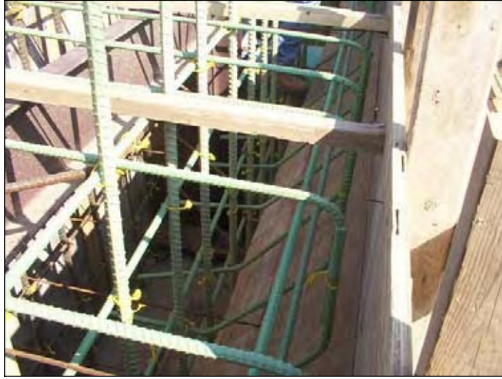
Figure 217. Abutment and paving notch rebar tied with reinforcement from the backwall
