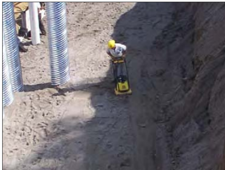
Figure 201. Compaction of retaining wall fill material (South end of SBL)
