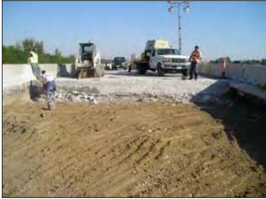
(a) Replaced approach slab
