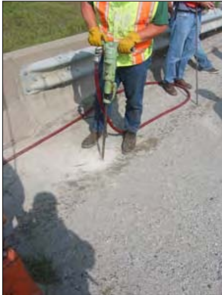
(a) Drilling at the approach slab
