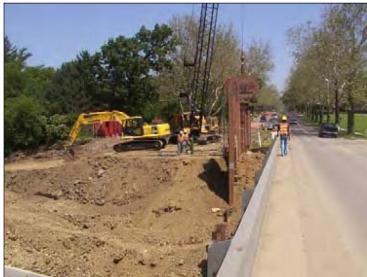
Figure 193. Installation of the sheet piles (NBL)
