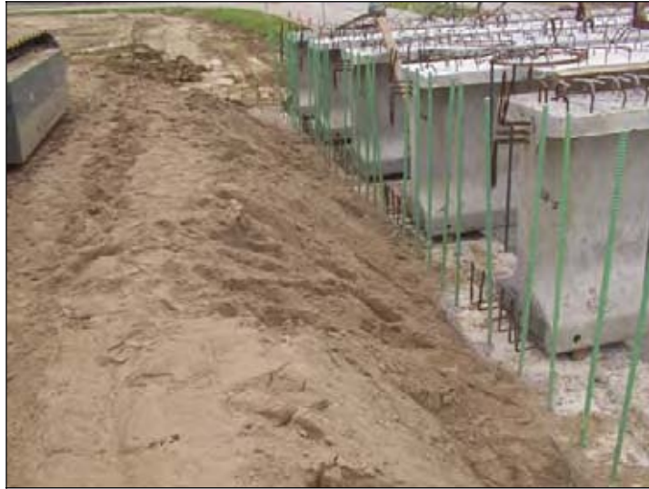
Figure 184. Granular Backfill used behind the abutment
