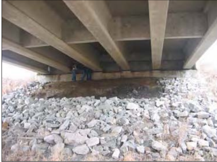
Figure A1. Rocks used to decrease erosion at the embankment
