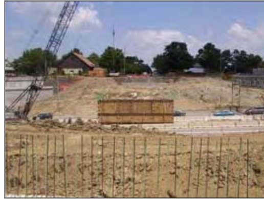
(b) Center pier construction
