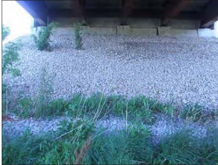
Figure 248. Aggregate slope protection at the bridge embankment (North end of NBL)
