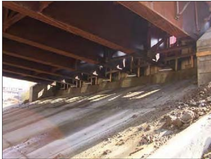
Figure 213. Embankment concrete slope protection
