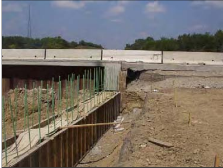
Figure 226. Abutment reinforcement and backfill placed at the northbound approach slab
