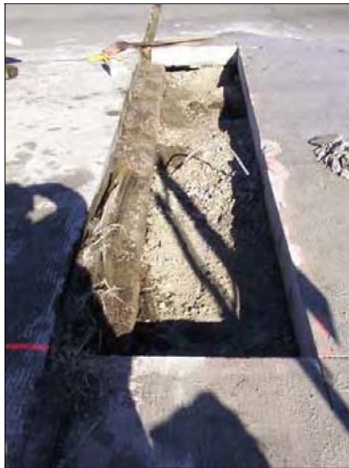
Figure A8. Removed section of the approach slab
