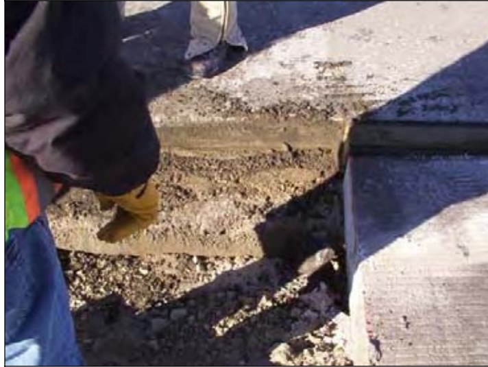
Figure 57. Layer of fine sand covering the paving notch
