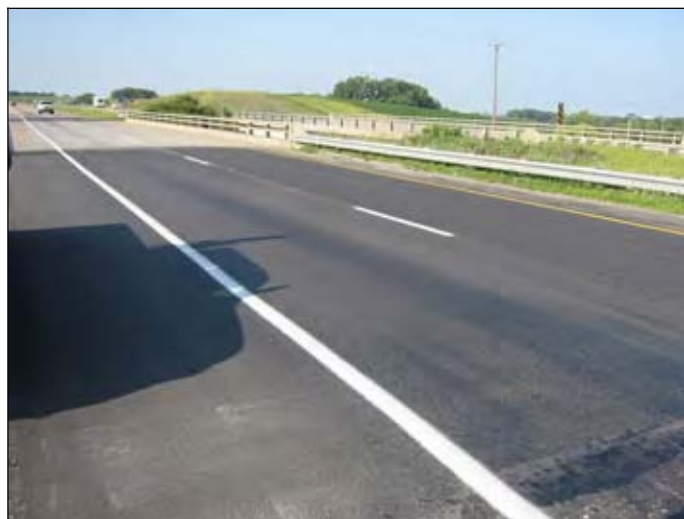
Figure 115. New asphalt-resurfaced approach
