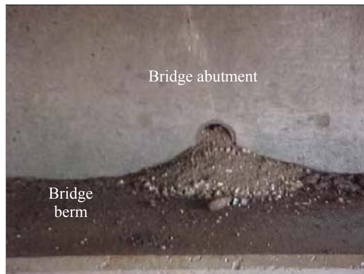
Figure 37. Weep holes filled with backfill material
