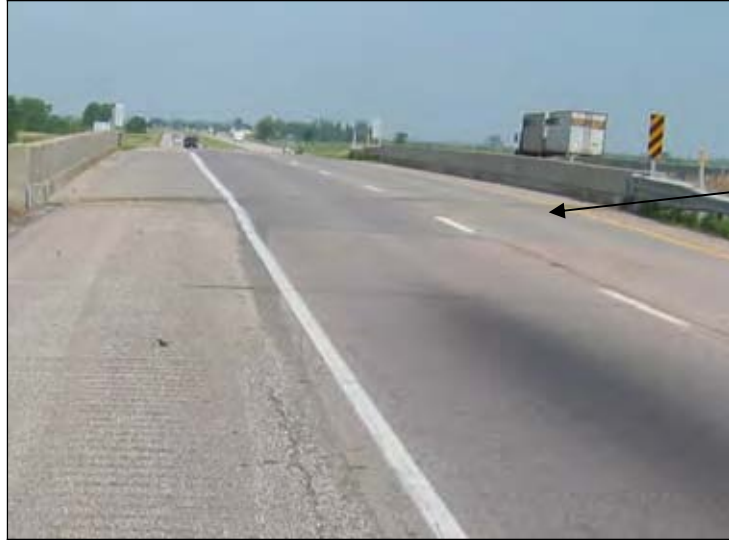
Figure 127. Settlement of bridge approach
