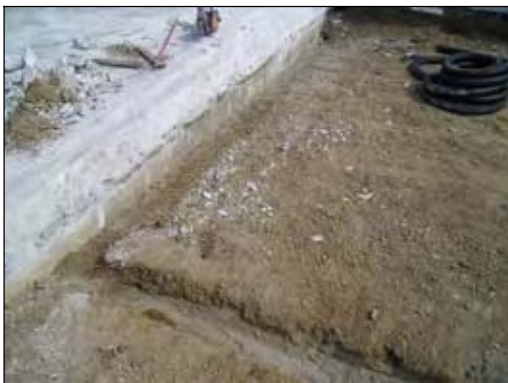
(a) Trench excavated to install subdrain
