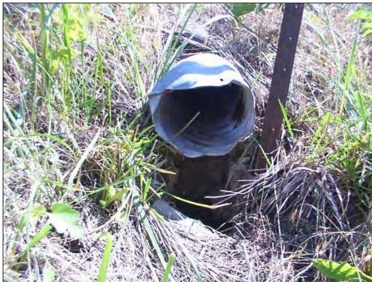
Figure 246. Subdrain prior to insertion of snake camera (North end of NBL)
