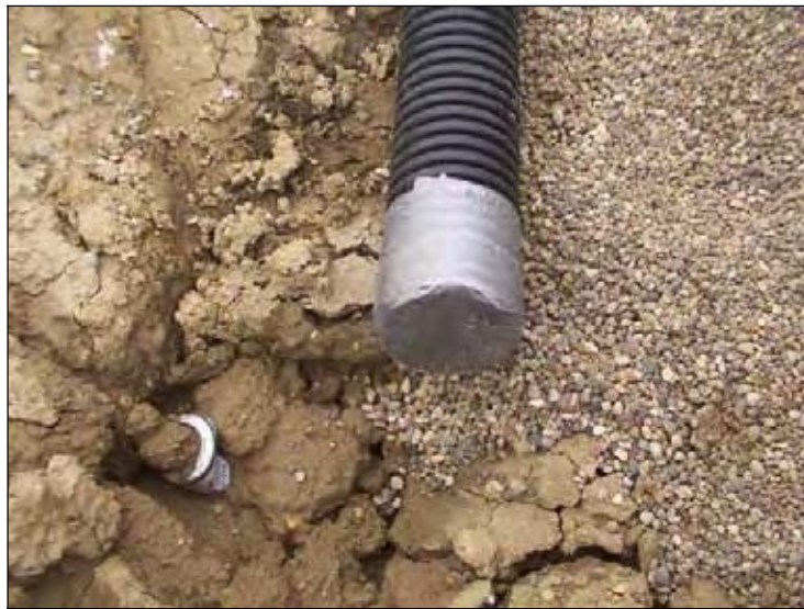
Figure 185. Porous fill placed around the drainage pipe
