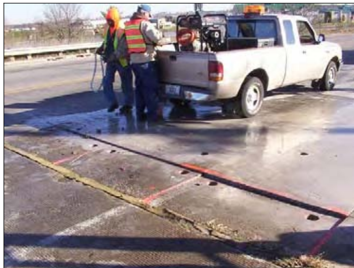
Figure 54. Section of the approach slab cut and ready to be removed
