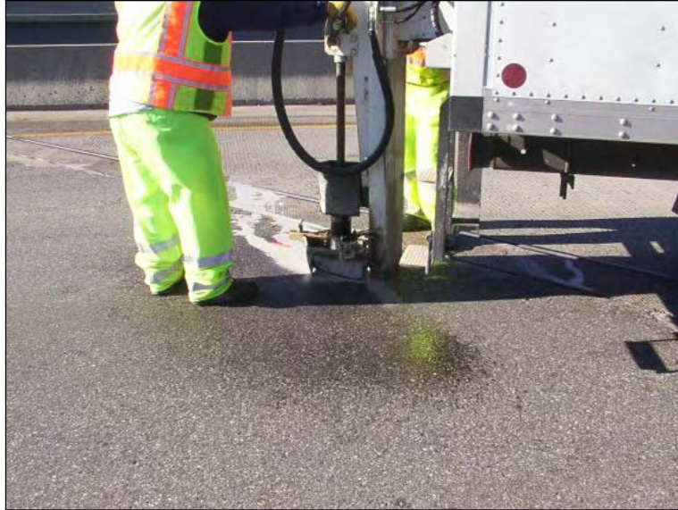
Figure 313. Coring at bridge approach (NBL)
