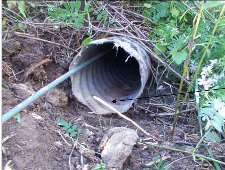
Figure 291. Iowa DOT snake camera inserted inside the subdrain
