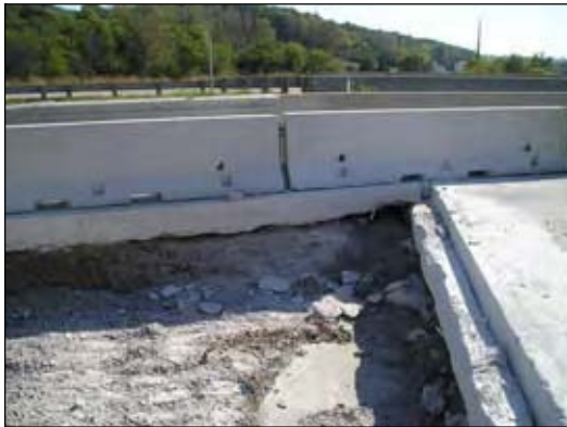
(a) North end approach slab
