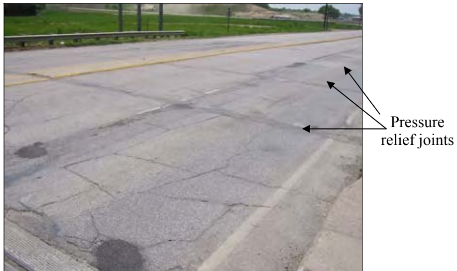
Figure 102. Pressure relief joints cut at the approach slab
