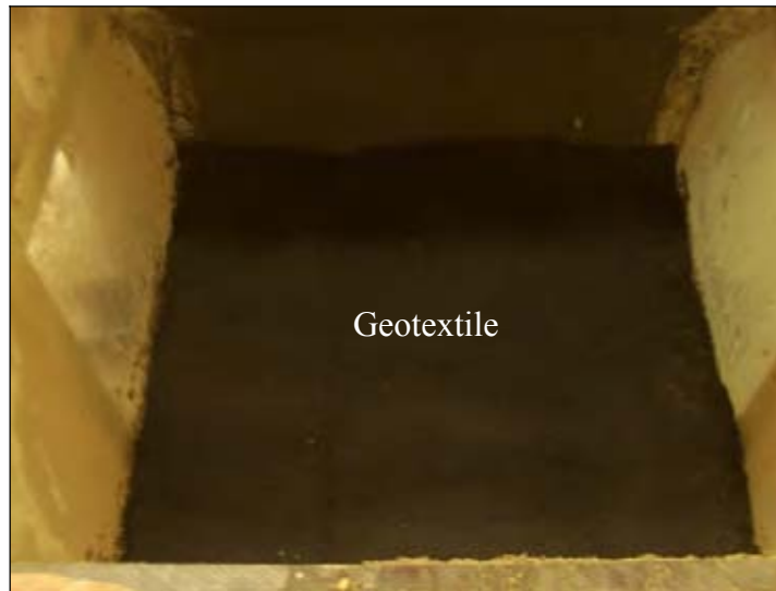
Figure 376. Placing backfill reinforcement
