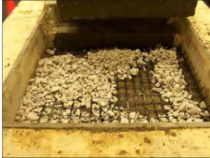
Figure 362. Placing special backfill over geogrid
