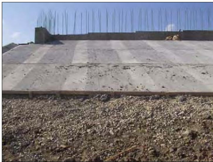
Figure 229. Construction of embankment slope protection
