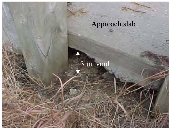
Figure 33. Void developed under the approach slab (South end of North bound bridge)
