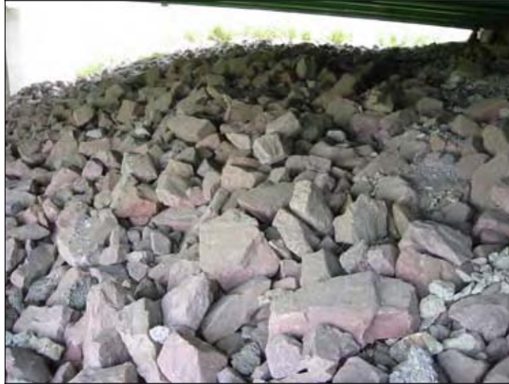
Figure 101. Aggregate used as embankment slope protection
