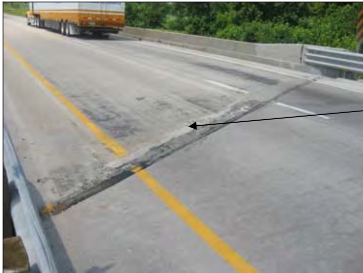
Figure 128. Concrete spalling at the expansion joint
