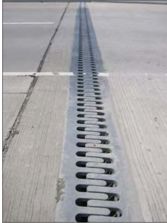
Figure 100. Finger type joint
