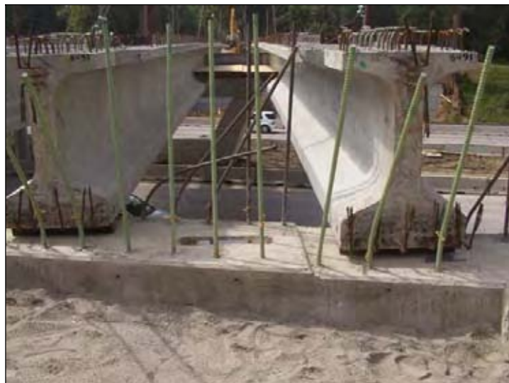
Figure 197. Sand used as granular backfill material
