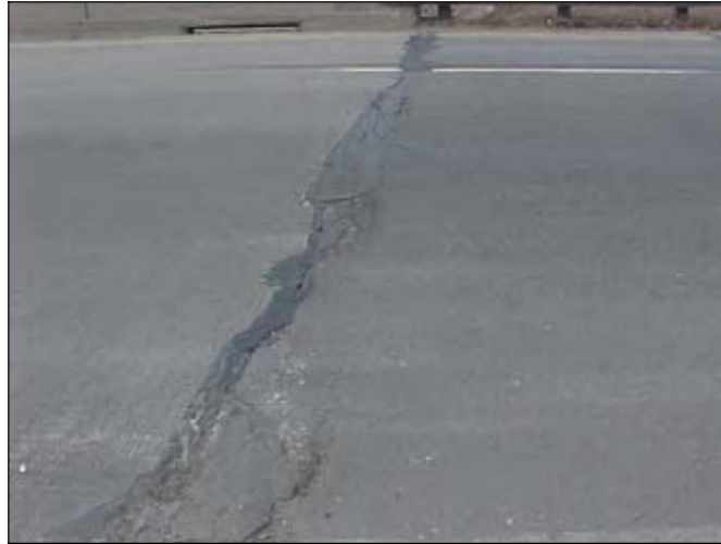
Figure 38. Expansion joint covered after placing the approach slab overlay (EBL)
