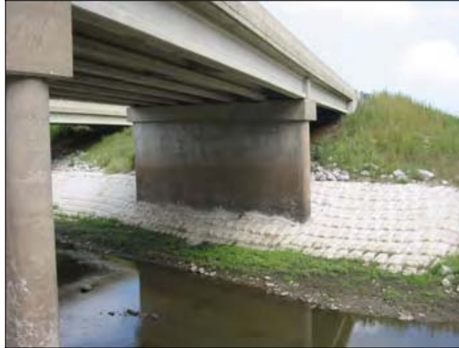
Figure 174. Rocks and pillows used for embankment stabilization
