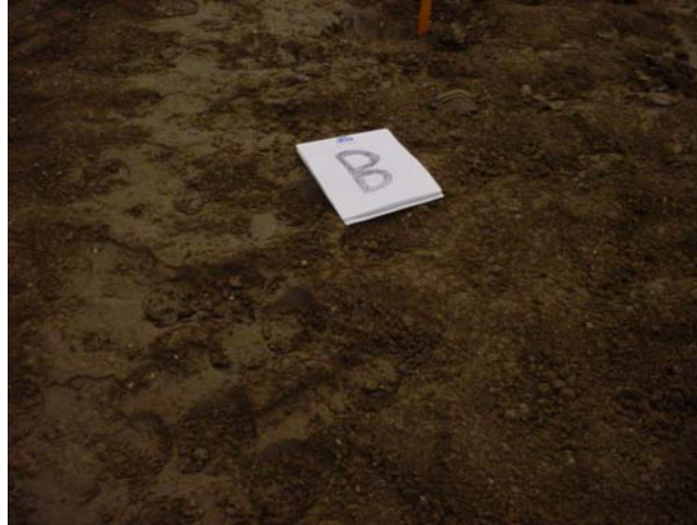
Figure 34. Surface condition after compaction for Test Strip B
