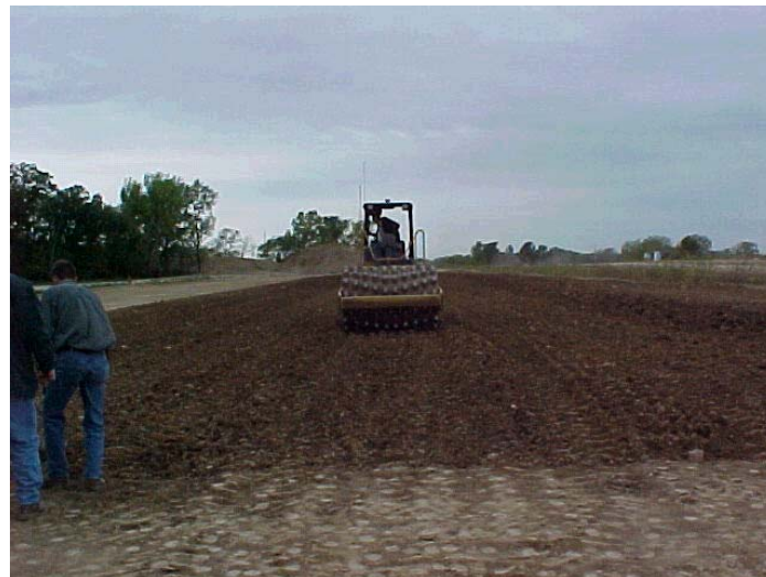
Figure 11. Compaction being performed by CAT CP-533E roller in reverse direction for test strip 2A
