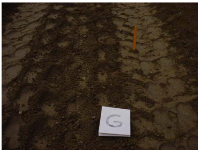
Figure 39. Surface condition after compaction for Test Strip G
