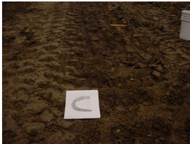
Figure 35. Surface condition after compaction for Test Strip C
