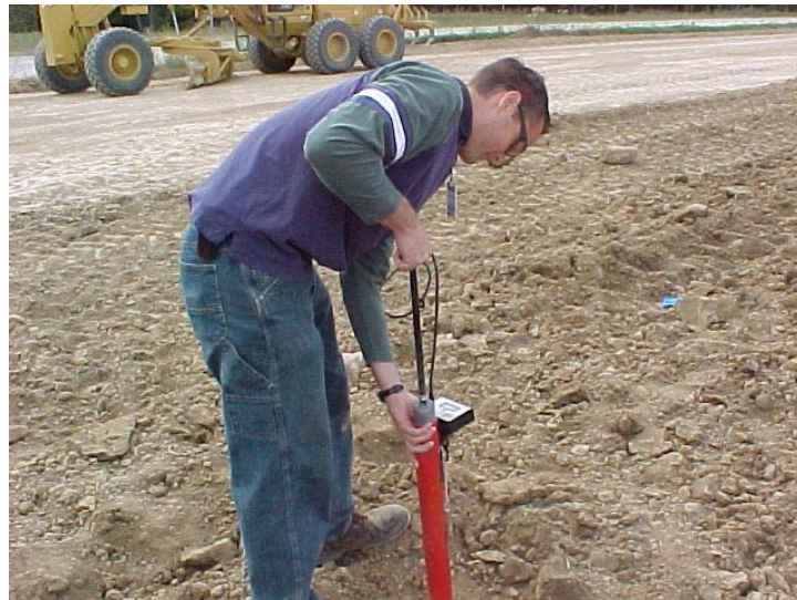
Figure 13. CIV stiffness measurements using the Clegg impact hammer
