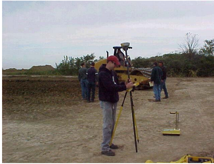
Figure 12. Trimble GPS base-station system used in situ test point locations
