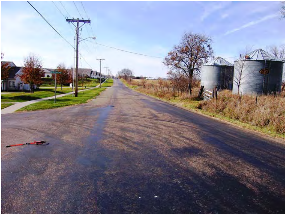
Figure F.6. Typical view of pre-coated pea rock on 74th Street (digitally enhanced photo)
