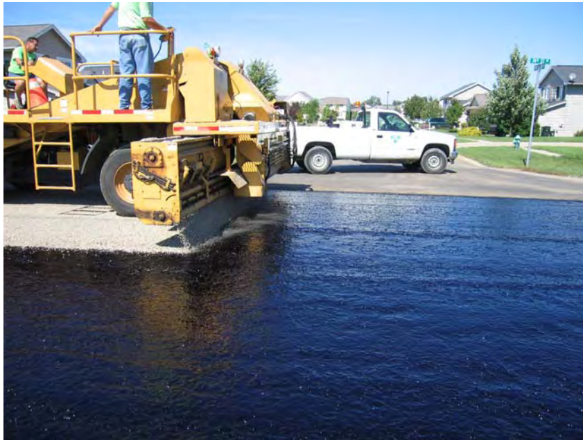
Figure 10. Seal coat construction on 74th Street
