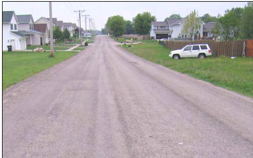
Figure 32. 74th Street double seal coat
