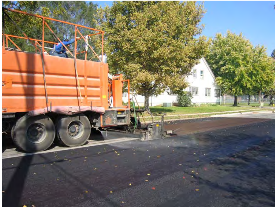
Figure 23. Micro-surfacing construction
