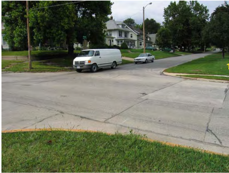
Figure 21. Vine Street before construction
