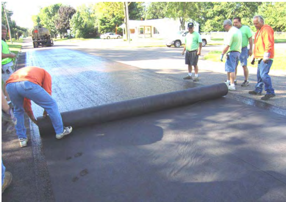
Figure 5. Placement of the fabric in the tack coat
