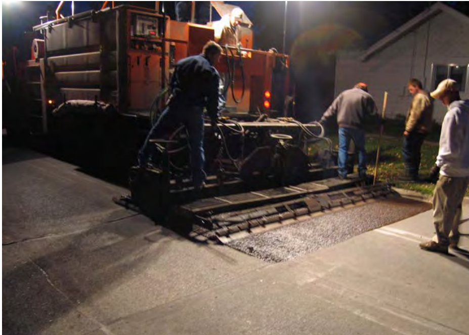
Figure 22. Night test section construction
