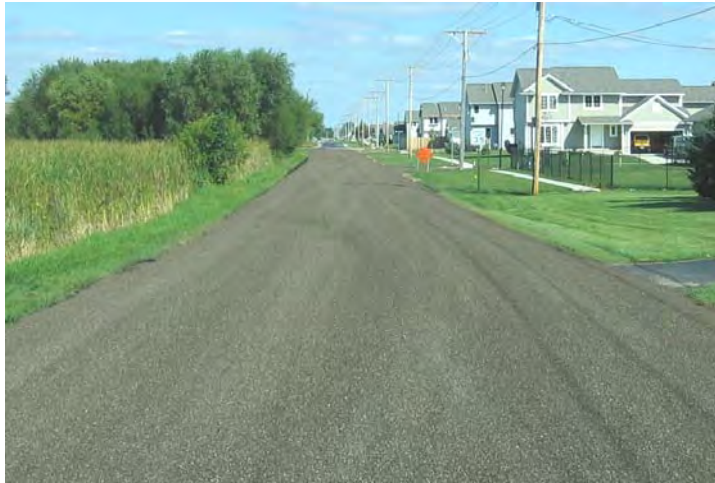
Figure 28. 74th Street pre-coated chips
