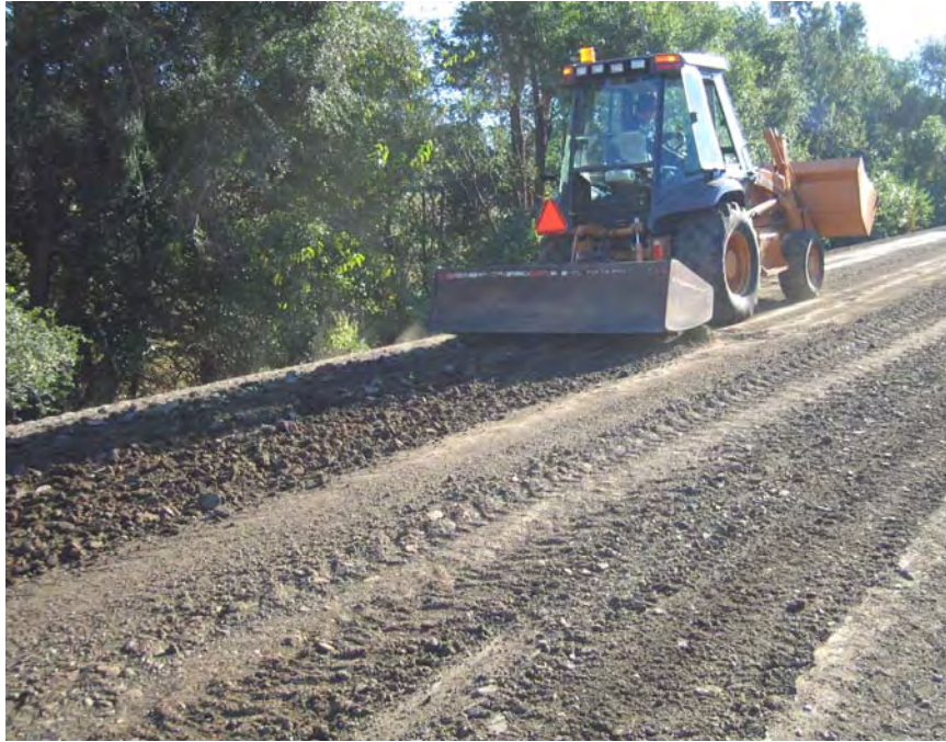
Figure 14. Stabilization of College Road
