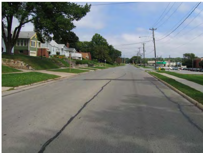
Figure 20. Fourth Street before construction
