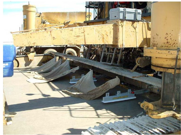
Measuring pavement profile during construction using the Ames Engineering Real Time Profiler (RTP)
