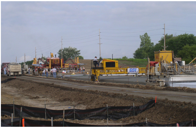
Measuring pavement profile during construction using the GOMACO Smoothness Indicator (GSI)
