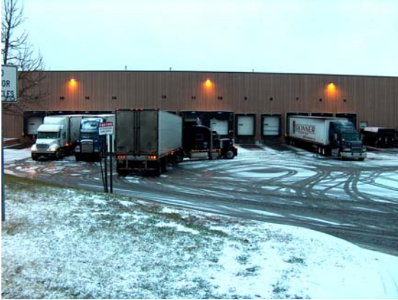
Figure 2-2. Terminal with inadequate maneuvering and parking space
