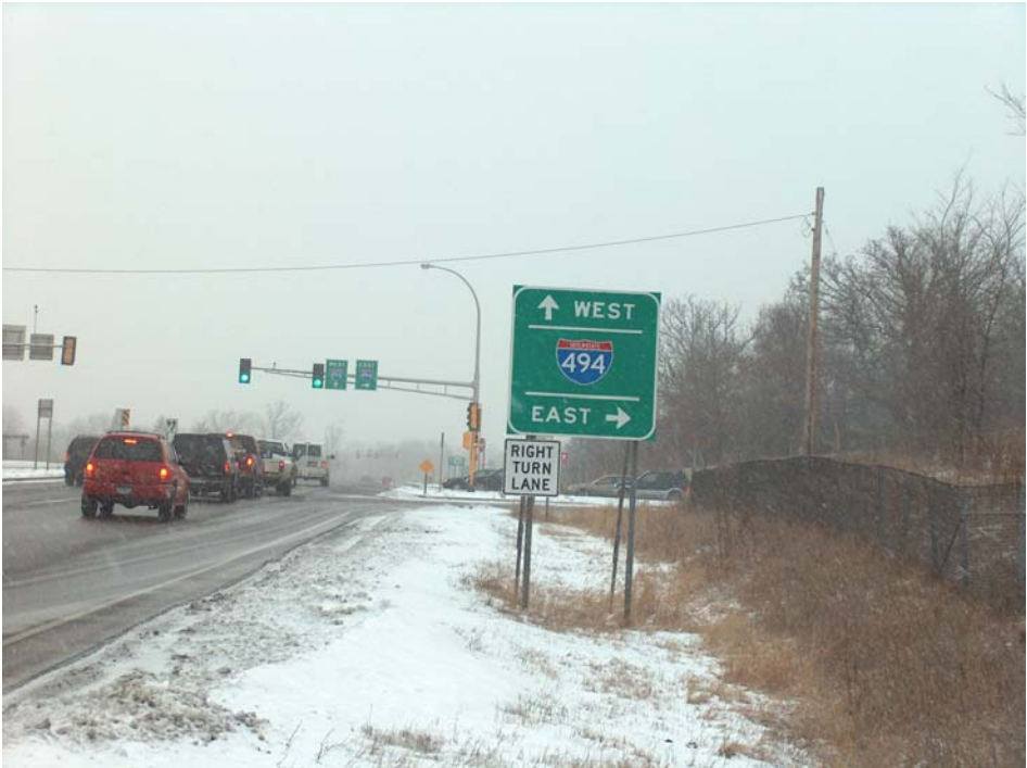
Figure 5-4. Guidance signage at south ramp terminal intersection
