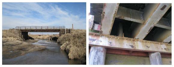
Figure 3. A representative steel-timber bridge
