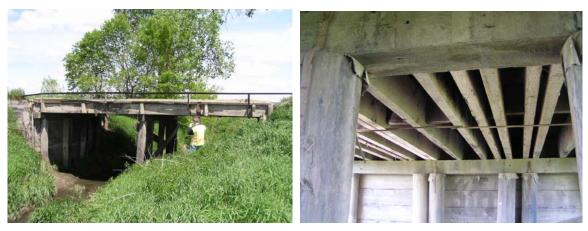
Figure 4. A representative timber-timber bridge
